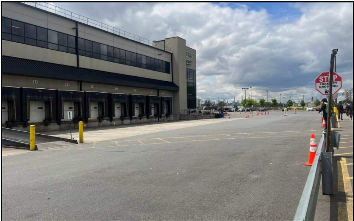
Photo 2: Facing west in the northern portion of Site E OU-1; asphalt and reinforced concrete slab in the northern truck loading dock in good condition.
