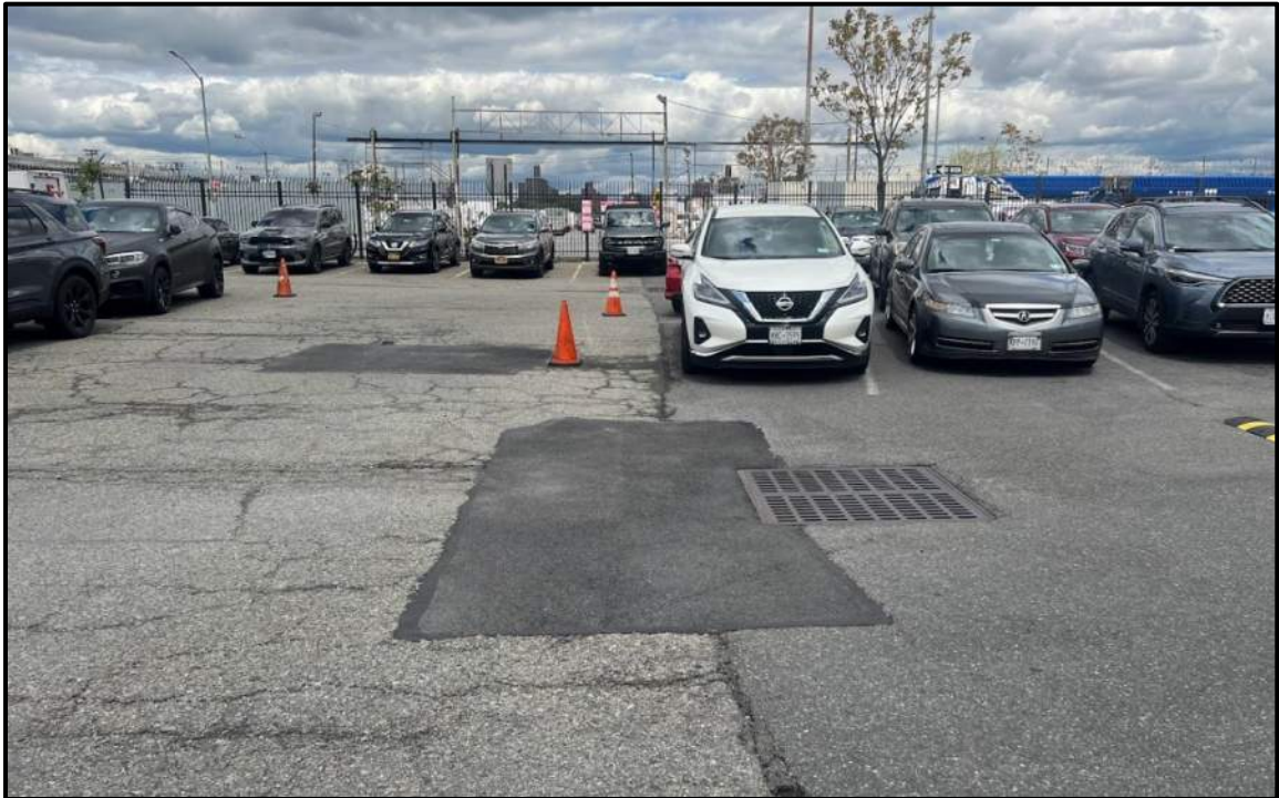
Photo 7: Facing north in the northern portion of the site in the employee parking area; lot generally in good condition, with minor cracking in the pavement. Evidence of asphalt patching.
