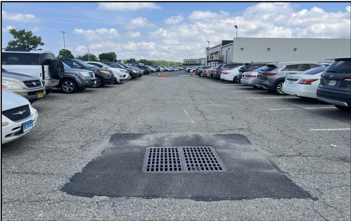
Photo 2: Facing east in the northern employee parking lot of Site E OU-1, adjacent to Site entrance; catch basin was recently reset and the surrounding pavement repaired on June 1, 2024. Minor wear in the surrounding pavement.
