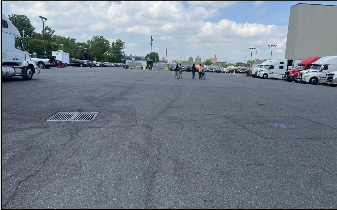
Photo 3: Facing north near the western truck loading area of Site E OU-1; asphalt in fair condition, with minor cracking, as well as former asphalt patching around utilities.
