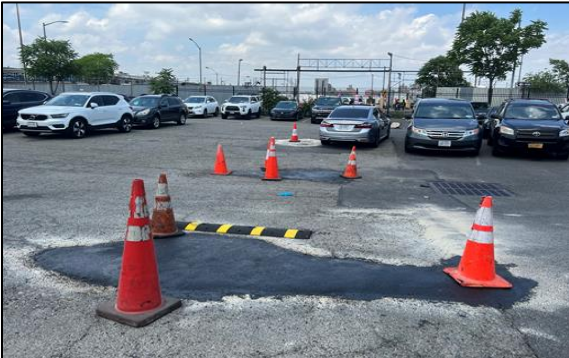
Photo 4: Facing north in the northern employee parking lot of the Site; evidence of the June 2024 non-invasive patching efforts, as well as former pavement repairs which are in fair condition.
