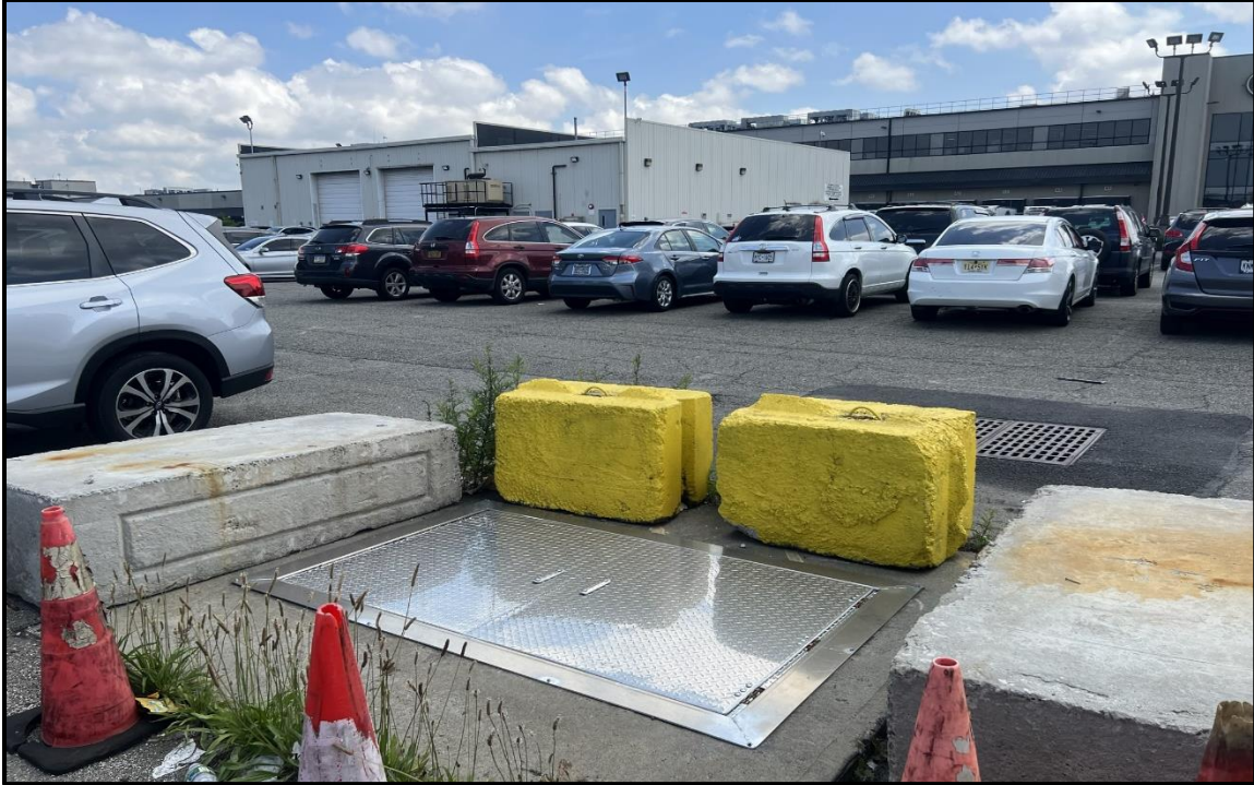
Photo 1: Facing south along the northern Site perimeter, in the employee parking lot; concrete pad around utility vault in fair condition with vault doors recently replaced.
