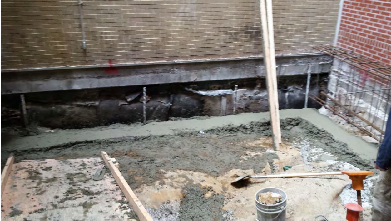
November 9, 2015 photo of eastern wall in renovated space. Top 2-3 ft of Vapor Barrier (black Hydroduct) temporarily exposed.
