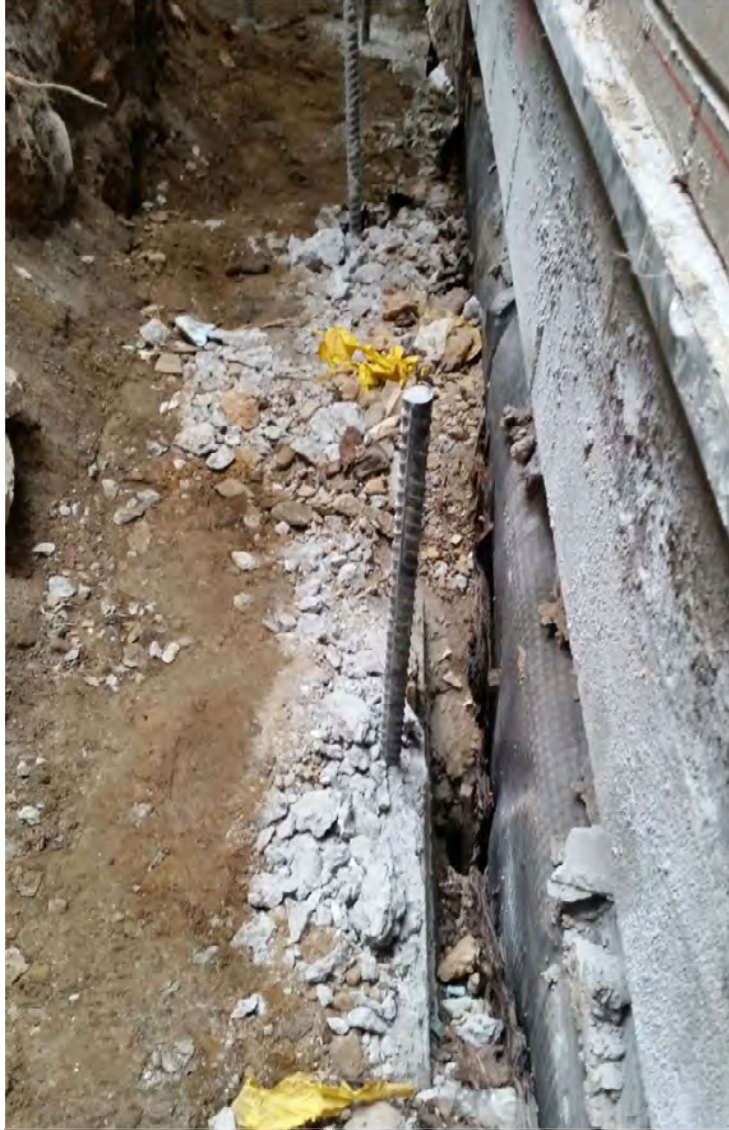
October 2015. A portion of the Vapor Barrier along western portion of the subject school building exposed to approximately 2-3 ft below grade.
