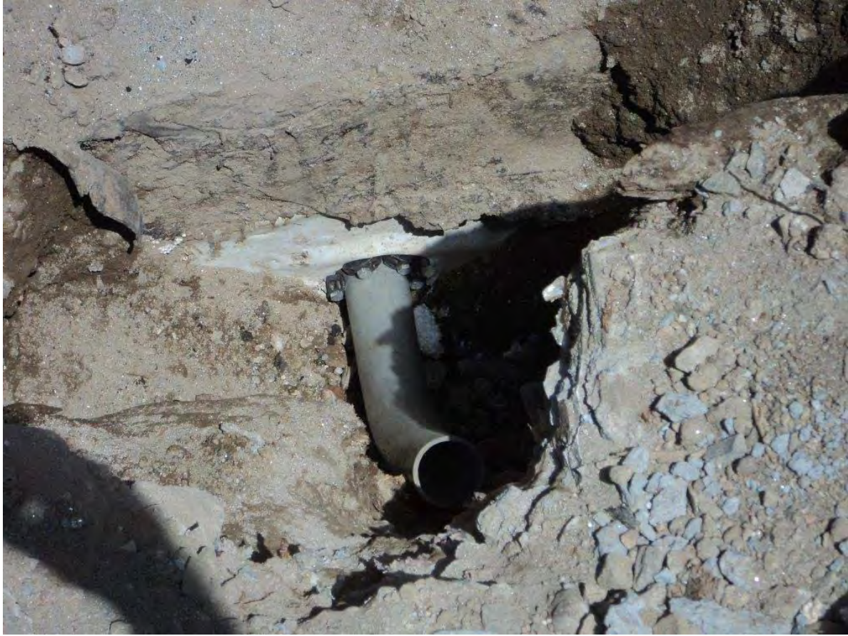
Photos of fiber conduit penetration. Existing vapor barrier components visible above and surrounding (in white).
