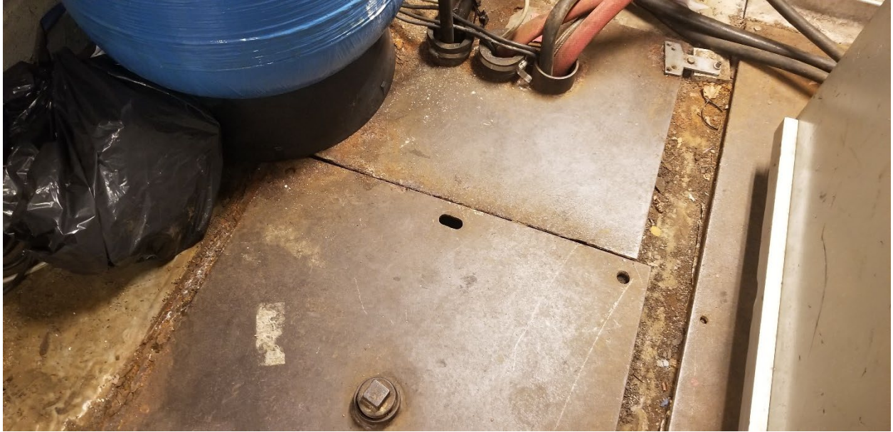
Metal plate covering the sump pit in the SW Pit Room, 06/24/2021.
