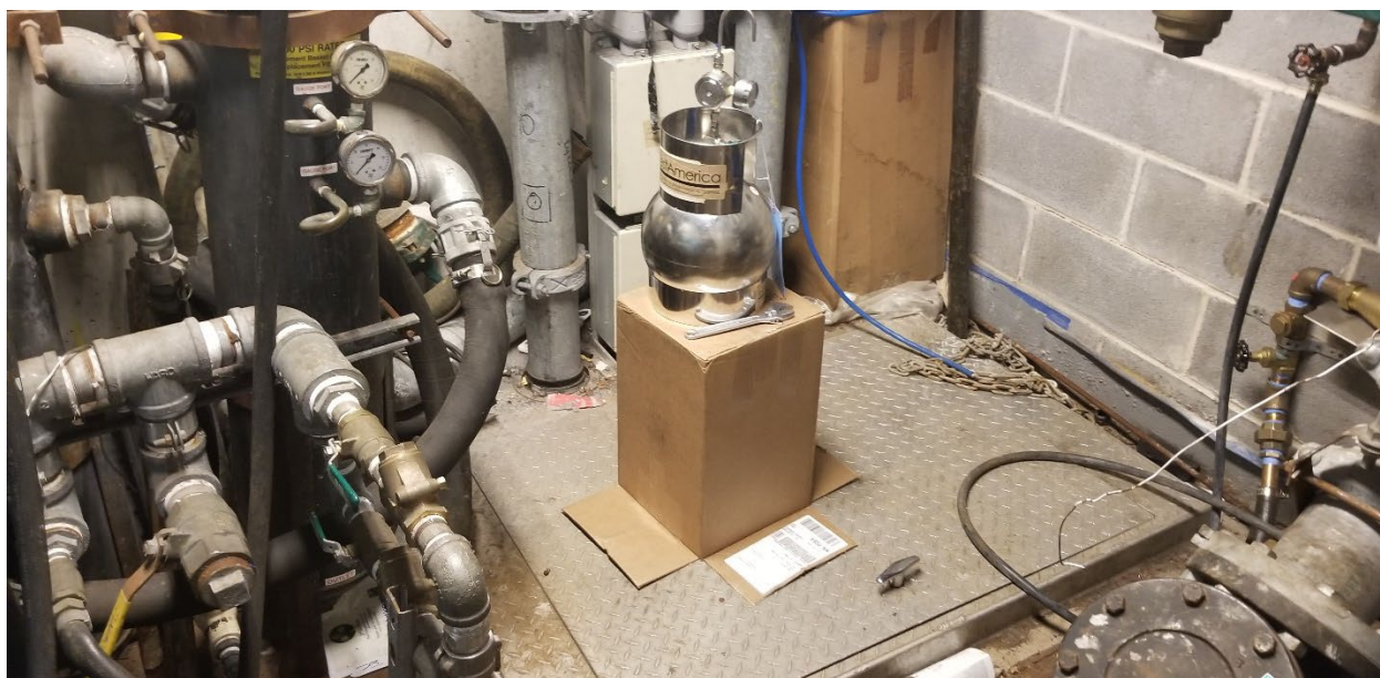
SW Pit Room sample collection, 06/24/2021.
