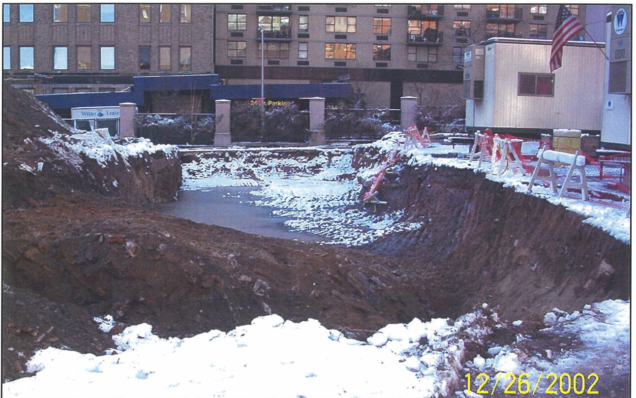
Photo 2. Western extent of remedial excavation.
