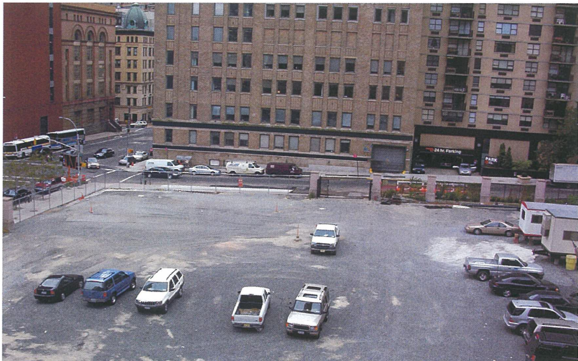
Photo 20. View of Parking Lot Site following completion of all remediation and site restoration.
