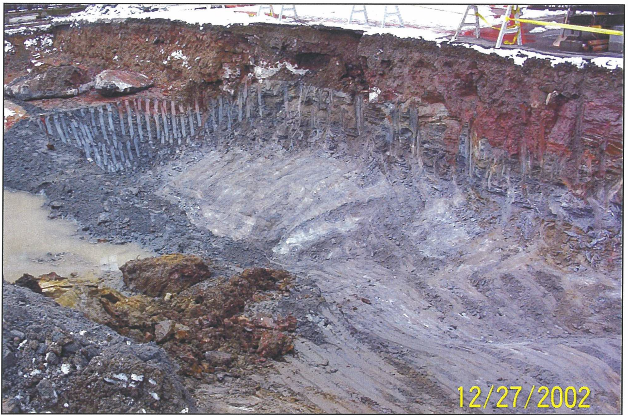
Photo 3. VOC – impacted soil area in the southwestern portion of the Site. Remedial excavation extended to top of competent bedrock due to VOC impacted weathered bedrock.
