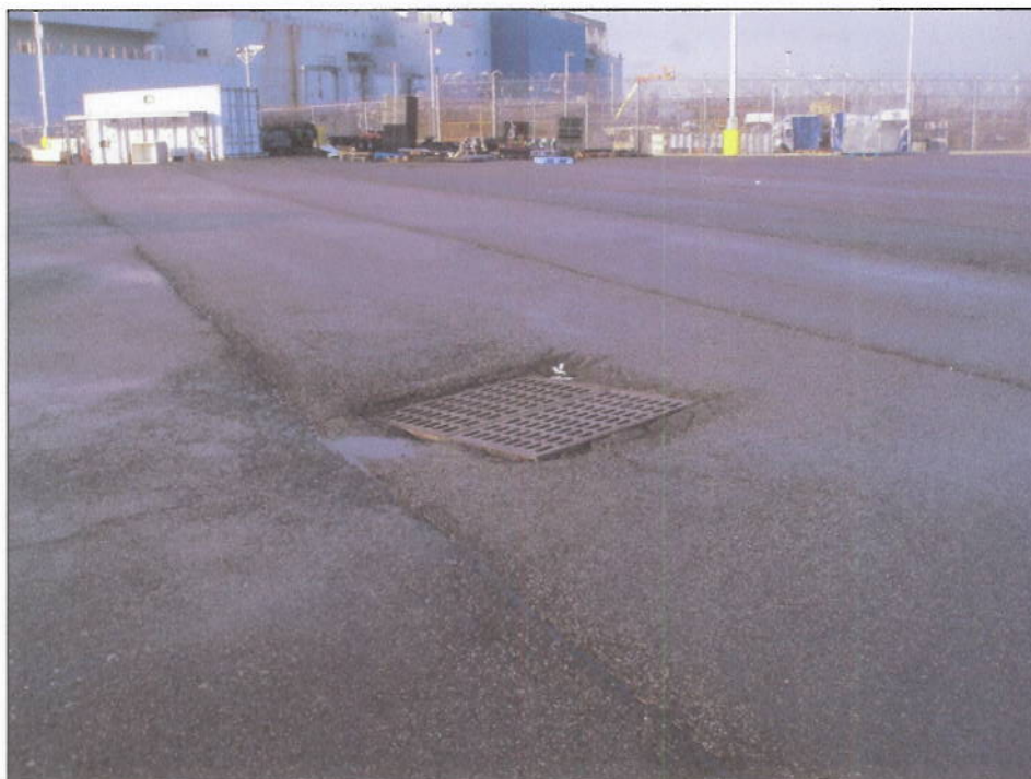
Photograph No. 12 – The New Fulton Fish Market southwest parking portion, one of the remaining Catch Basins for repair
