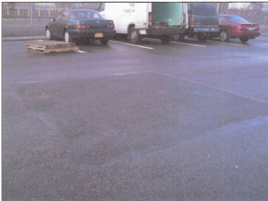
Photograph No. 11 – The New Fulton Fish Market west parking portion, pothole repair at Site B
