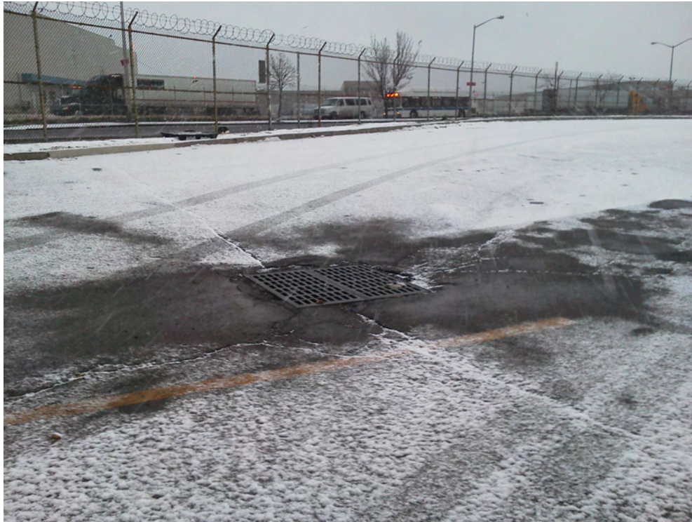
Photograph No. 9 – The New Fulton Fish Market southwest parking portion, one of the remaining Catch Basins for repair
