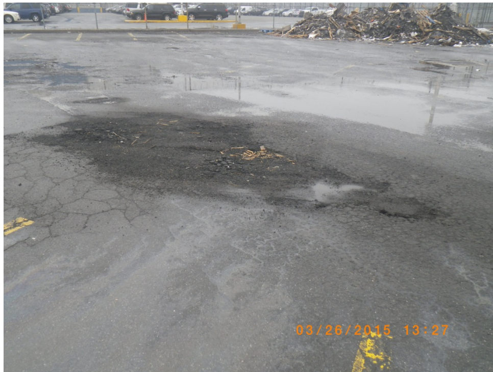
Photograph 3 – The New Fulton Fish Market Southern Parking Lot, example of asphalt area with deterioration that will be repaired (looking south)
