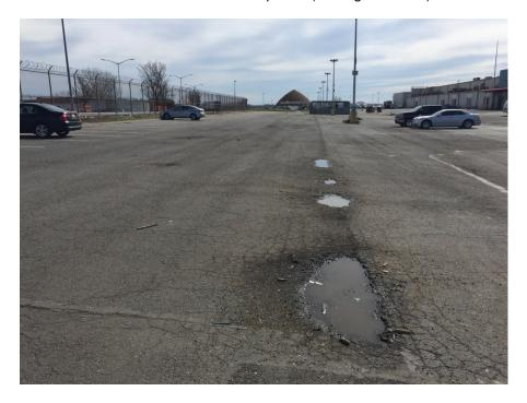
Figure 4 – New Fulton Fish Market northern roadway (looking east) Potholes visible.
