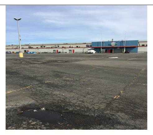
Photograph 3 – The New Fulton Fish Market Southern Parking Lot, example of asphalt area with deterioration that will be repaired (looking northeast)
