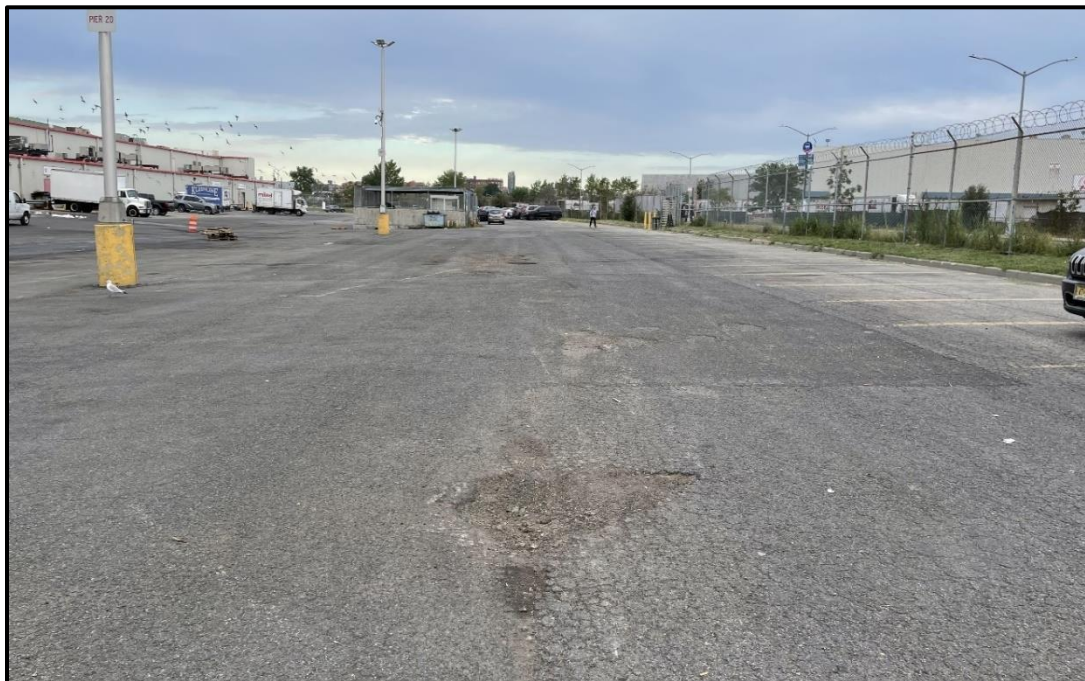
Photo 12: Facing north in the eastern portion of Site; engineering controls are still in place. Normal wear from heavy truck traffic in the form of asphalt cracks and potholes of various sizes are present in the parking lot.
