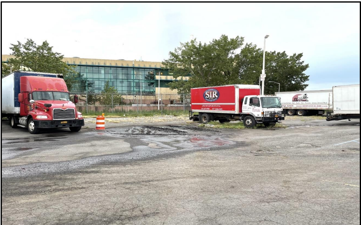
Photo 2: Facing west in the western portion of Site; low laying area with soil and debris accumulation. The engineering cap remains in place with some vegetation growing through cracks in the asphalt.
