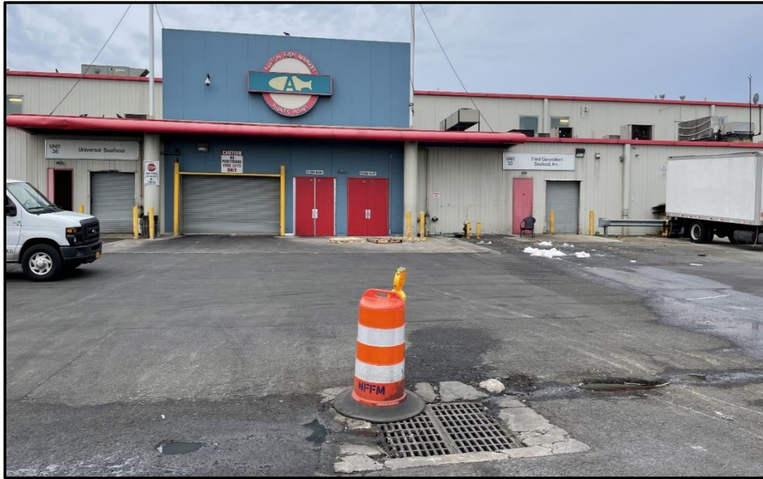
Photo 11: Facing west in the eastern portion of Site; engineering controls are still in place. Normal wear from heavy truck traffic in the form of asphalt cracks and potholes of are present in the parking lot, particularly around the catch basins. No subgrade exposed.
