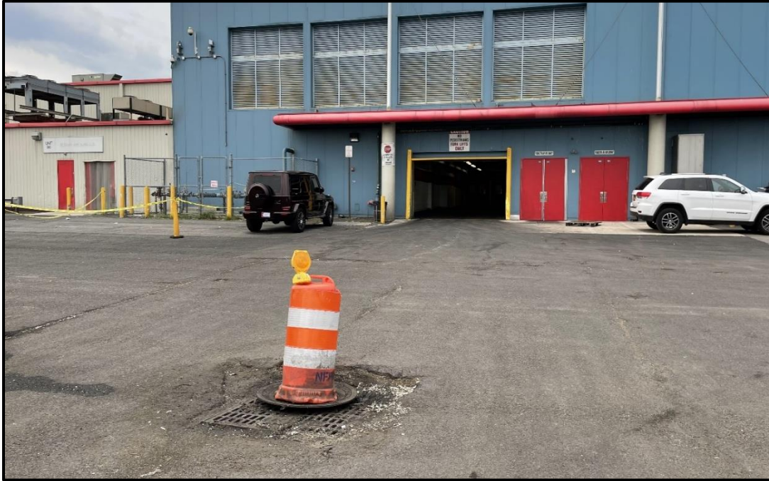
Photo 13: Facing west in the eastern portion of Site; engineering controls are still in place. Normal wear from heavy truck traffic in the form of asphalt cracks and potholes of various sizes are present in the parking lot, particularly around the catch basins. No subgrade exposed.
