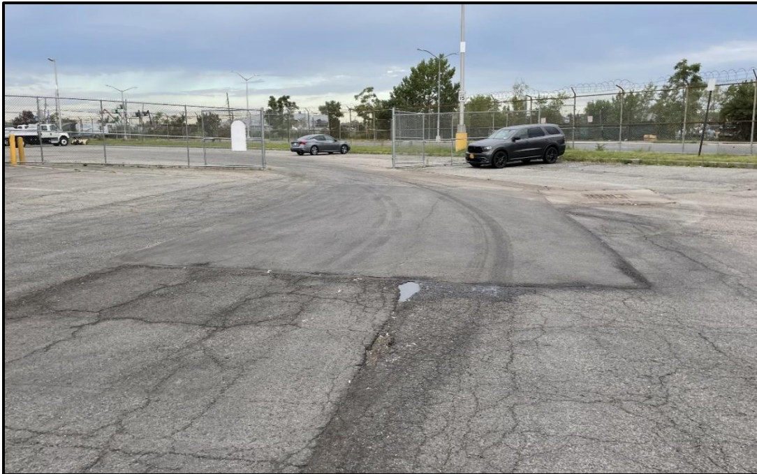
Photo 8: Facing north in the northern portion of Site; cracking and small potholes present.
