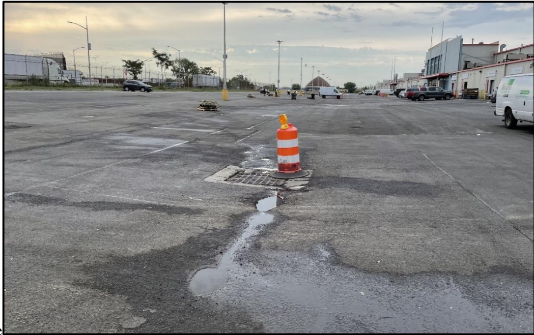
Photo 9: Facing southeast in the eastern portion of Site; potholes and cracking noted in the asphalt, particularly surrounding the catch basins.
