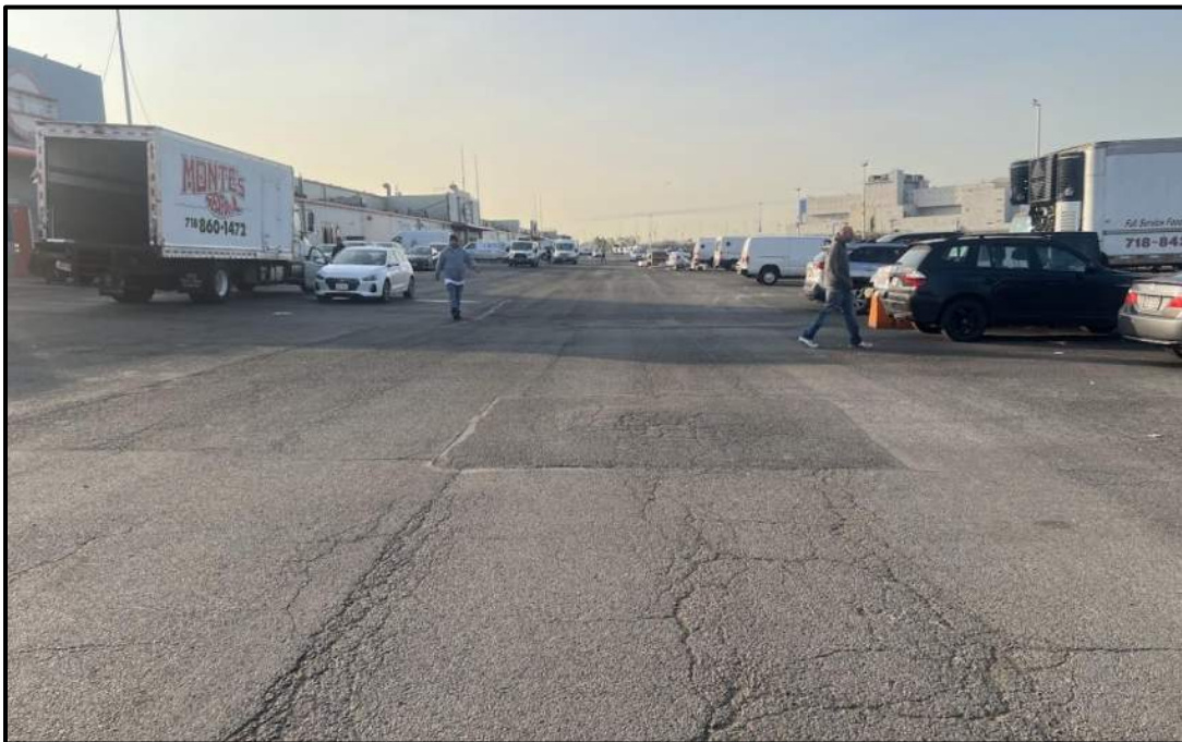
Photo 6: Facing south in the southwestern portion of Site; area of previous asphalt patching completed in August 2022. Minor cracking present.
