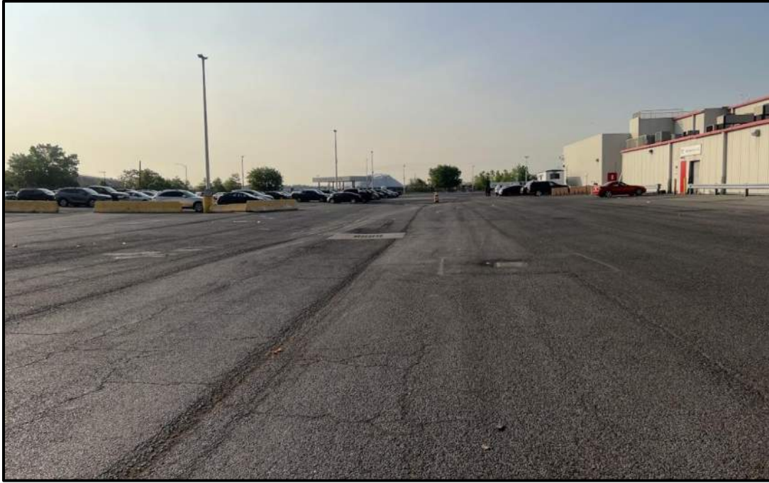
Photo 7: Facing southeast in the northeastern portion of Site; pavement in good condition with minor cracking. Previous utility repair in the background.
