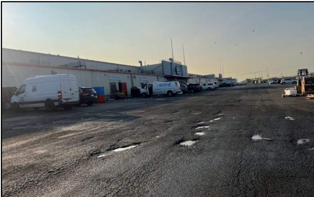
Photo 12: Facing south in the western portion of Site; engineering controls are still in place. Normal wear from heavy truck traffic in the form of asphalt cracks and potholes of various sizes are present in the parking lot.
