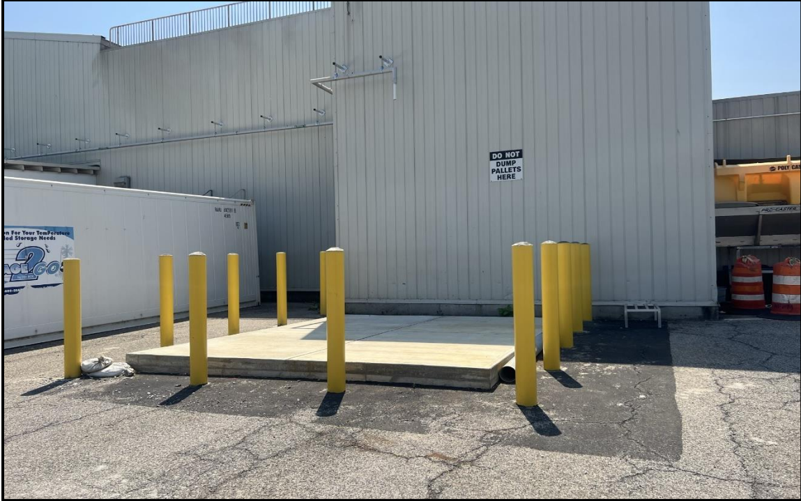
Photo 1: Facing south in the northern portion of Site, along the western dock; nitrogen tank foundation slab, constructed in July 2023, in good condition with engineering controls in place.
