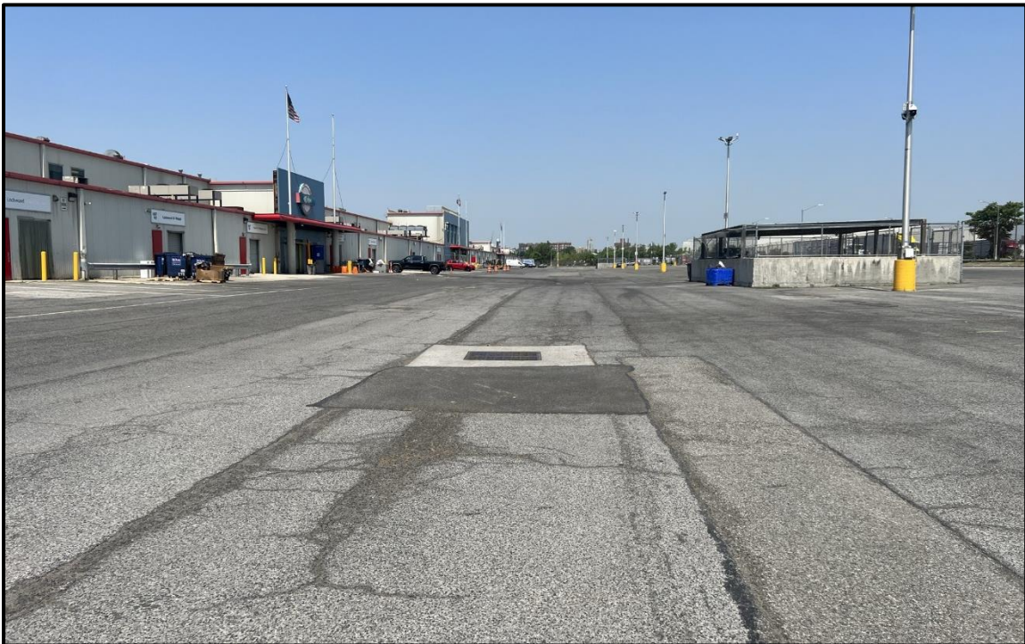
Photo 2: Facing northwest in the eastern portion of Parcel B; area of pavement repair completed in September 2023, as well as prior asphalt patching and utility repair efforts. Minor cracking present.
