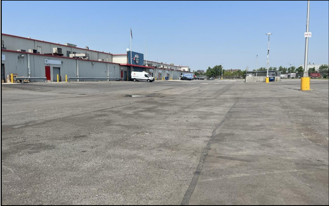
Photo 7: Facing northwest in the eastern portion of Site; engineering controls are still in place. Normal wear (minor cracking and potholes) from heavy truck traffic and patching from prior repair efforts noted.
