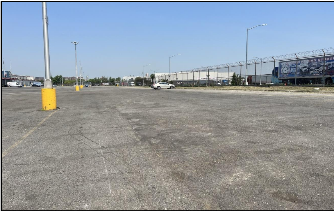
Photo 10: Facing north along eastern perimeter of Parcel B; minor cracks and potholes noted. Unpaved area along fenceline in fair condition, with vegetation noted.
