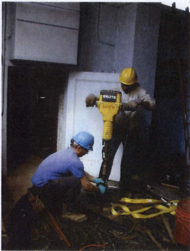
5. Rotary Hammer Installation of B-104.
