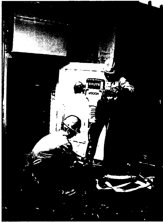
5. Rotary Hammer Installation of B-104.
