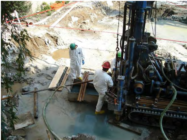
Hot Spot Delineation Borings Retrieving Bedrock Core from Location DB-9 April 29, 2009
