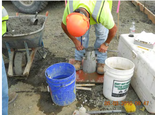
Site Restoration – Dumpster pad construction Performing Slump Test for Dumpster Pad Concrete August 3, 2010
