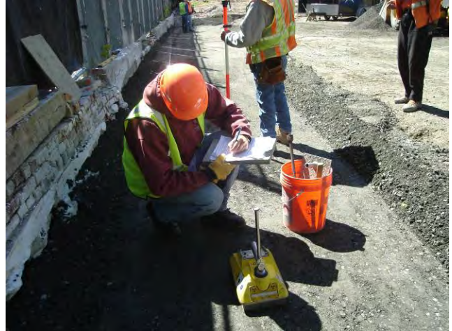
Site Restoration –Backfill Compaction Testing in Northeast Corner of Site April 29, 2010
