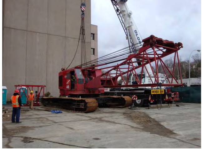
Auger ISS - Mobilization Crane Assembly February 12, 2009
