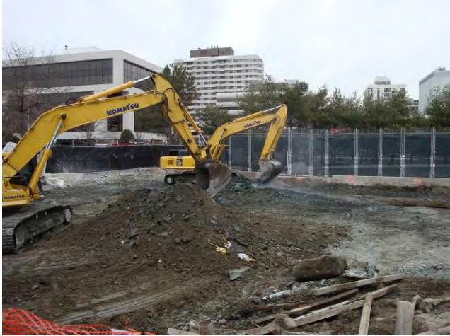
Excavator ISS – Lowering top elevation of ISS Scraping Down Top of ISS Monolith February 25, 2009
