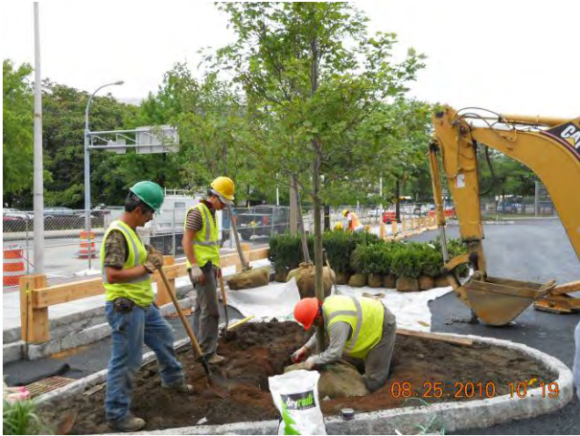
Site Restoration – Plantings Planting tree in Northwest planter island August 25, 2010
