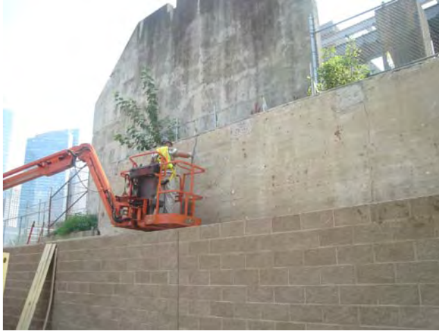
Site Restoration – Retaining Wall Stucco Installation Filling Cracks in Retaining Wall August 12, 2010
