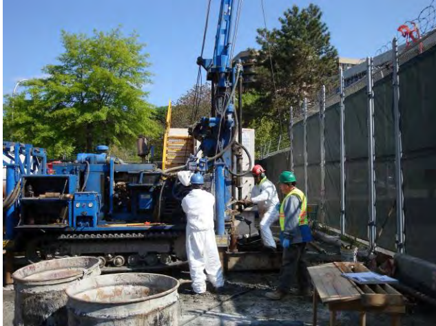
Excavator ISS – Delineation Borings Collecting ISS Core Samples May 12, 2009
