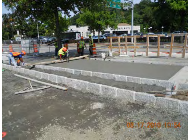
Site Restoration – Sidewalk Construction Concrete Finishing for Sidewalk Section August 11, 2010
