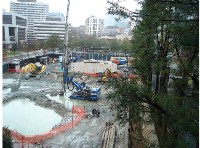
Jet Grouting – Column Installation Activities Installing Jet grout Column Int-88 December 9, 2009
