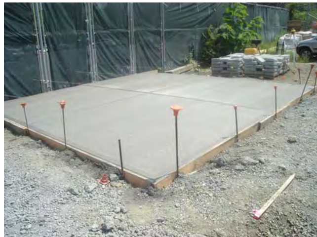
Site Restoration – Dumpster pad construction Concrete Pour for Dumpster Pad August 4, 2010
