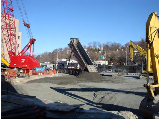
Backfill Placement & Compaction (East Side) Unloading Item #4 Backfill Material March 20, 2009
