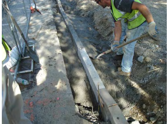
Site Restoration – Curbing Concrete Poured around New Street Curb August 13, 2010
