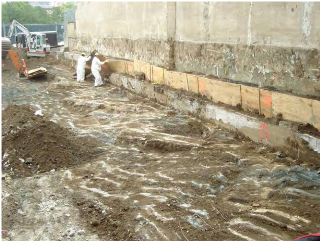
Site Restoration – Retaining Wall Removing forms from Cellular Concrete Pour June 14, 2010
