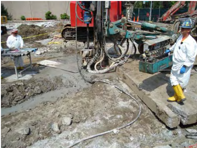
Jet Grouting – Test Column Installation Installation of Jet grout Test Column JG-3 June 29, 2009
