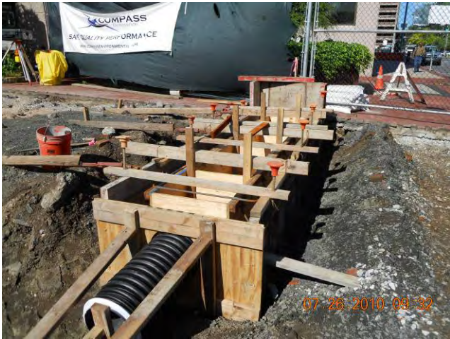
Site Restoration – Trench Drains Forms and rebar for Trench Drain CB-1 July 26, 2010
