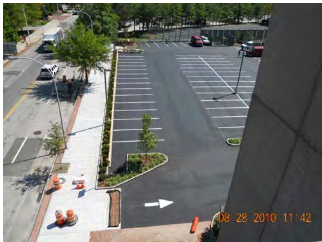
Site Restoration – Northern Area View Looking East August 28, 2010
