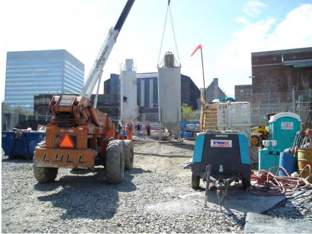
Jet Grouting – Demobilization Dismantling Batch Plant April 15, 2010
