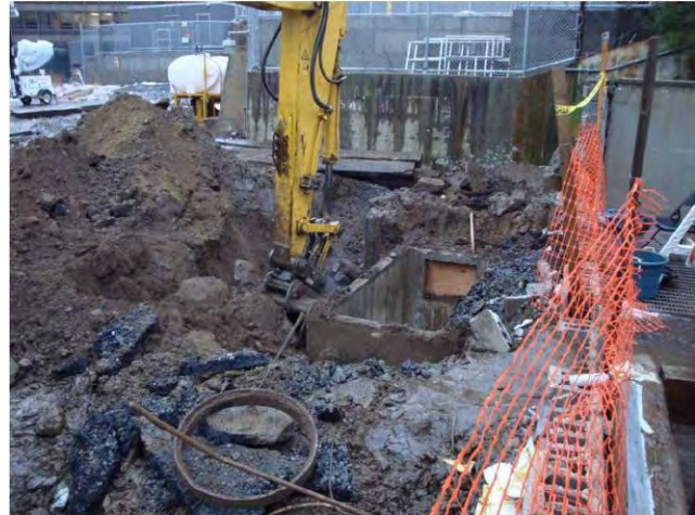
Switchyard Demo & Asbestos Abatement Excavation for Electrical Manhole #3 December 16, 2008
