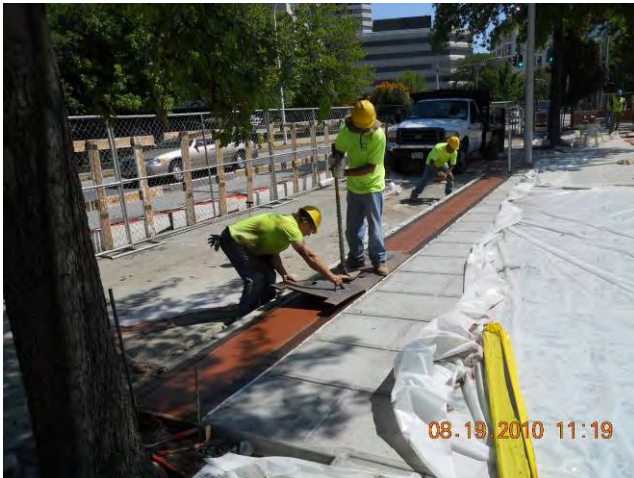
Site Restoration – Sidewalk Construction Stamping Brick Pattern into Concrete August 19, 2010
