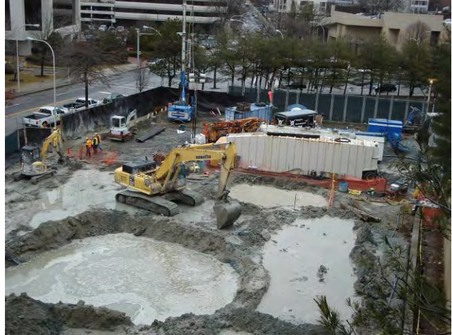
Jet Grouting – Column Installation Activities Jet Grout Spoils Sump Collection Areas February 24, 2009
