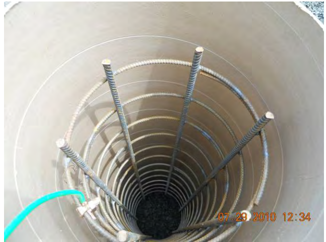
Site Restoration – Lighting Rebar Cage Placed in Light Pole Base Form July 29, 2010
