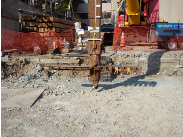
Auger ISS - Mobilization 9-foot Diameter Auger Attached to Kelly bar March 27, 2009
