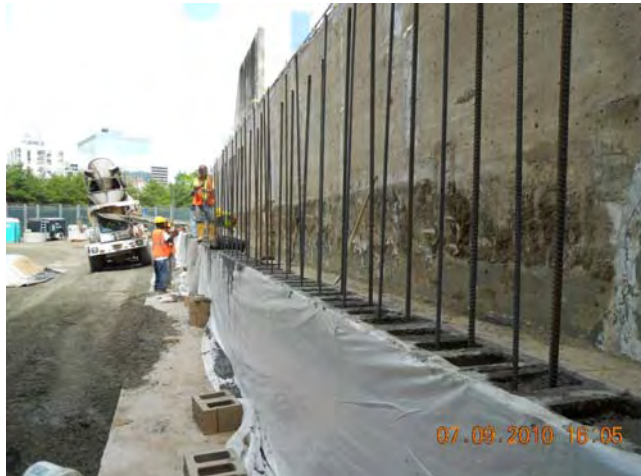
Site Restoration – Planter Wall Stucco Reconstruction Masonry Block with Reinforcing July 9, 2010
