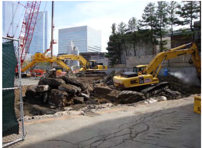
Demo of Structures for West Side Stockpiling Subsurface Structures March 27, 2009
