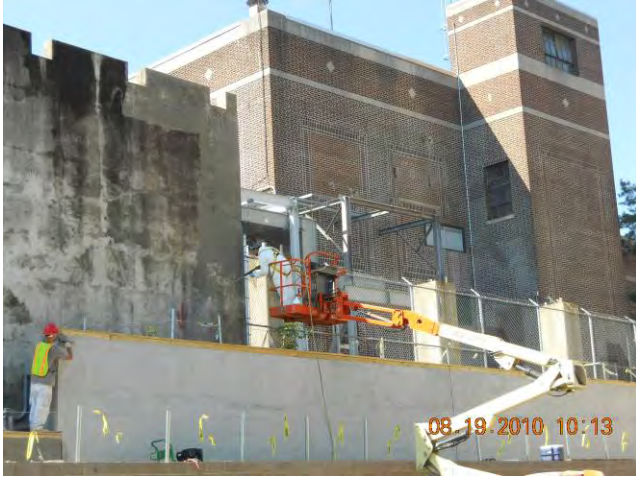
Site Restoration – Power Wash of Firewall Power Washing Firewall August 19, 2010
