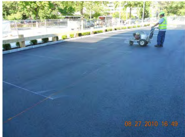
Site Restoration – Asphalt Placement Painting Parking Space Lines August 27, 2010
