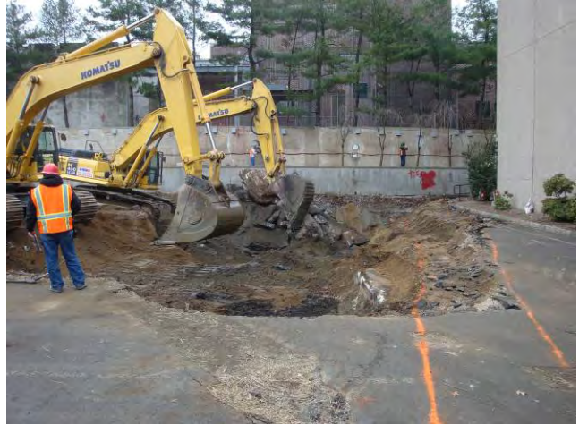
Demo of Structures for West Side Excavating Pavement and Subsurface Structures March 26, 2009
