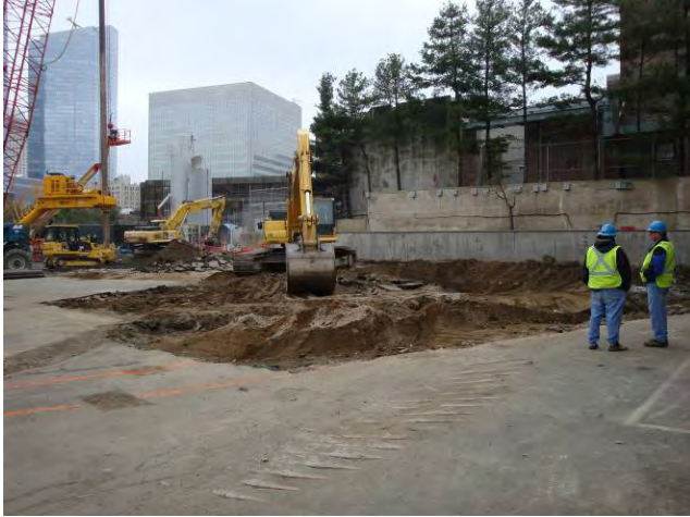
Demo of Structures for West Side Excavating Pavement March 26, 2009
