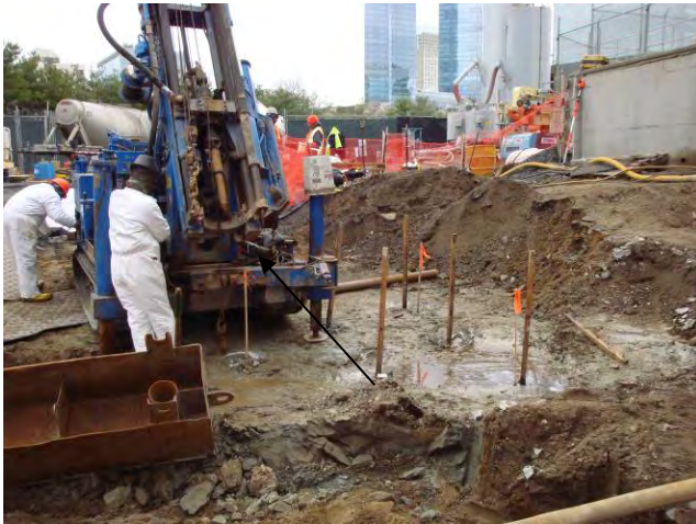
Auger ISS - Test Coring Program Drill Rig (CME-55) for Test Core Sampling April 7, 2009
