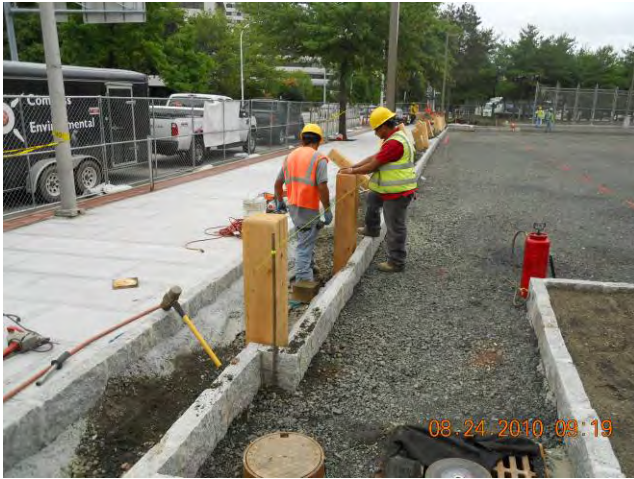
Site Restoration – Guide Rail Installing Guide Rail Posts August 24, 2010
