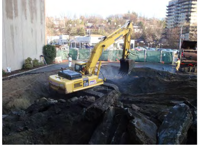
Demo of Structures for West Side Excavating Subsurface Structures March 27, 2009
