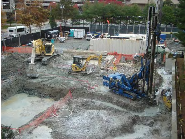
Jet Grouting – Column Installation Activities Installing Jet Grout Column SI-16 November 5, 2009
