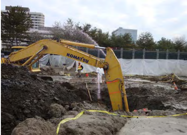
Excavator ISS – Cell Mixing Excavation Prior to Addition of Reagent for Cell EM-2 February 10, 2009
