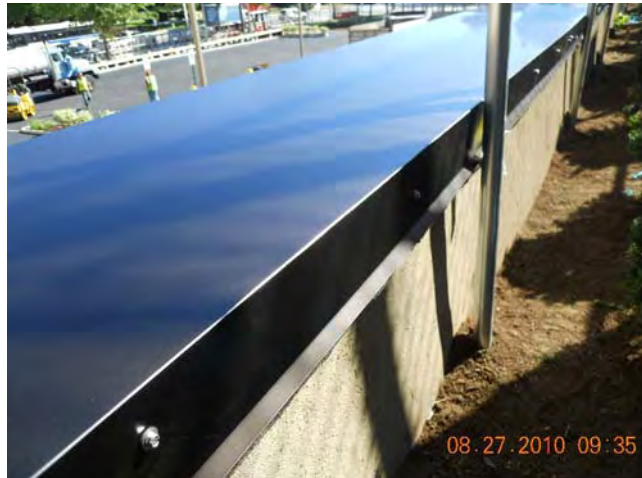
Site Restoration – Retaining Wall Installed Coping August 27, 2010
