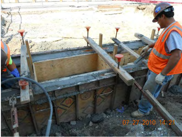
Site Restoration – Trench Drains Finishing Concrete for Trench Drain CB-2 July 27, 2010
