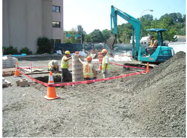
Site Restoration – Lighting Placing Light Pole Base Form in Excavation July 19, 2010
