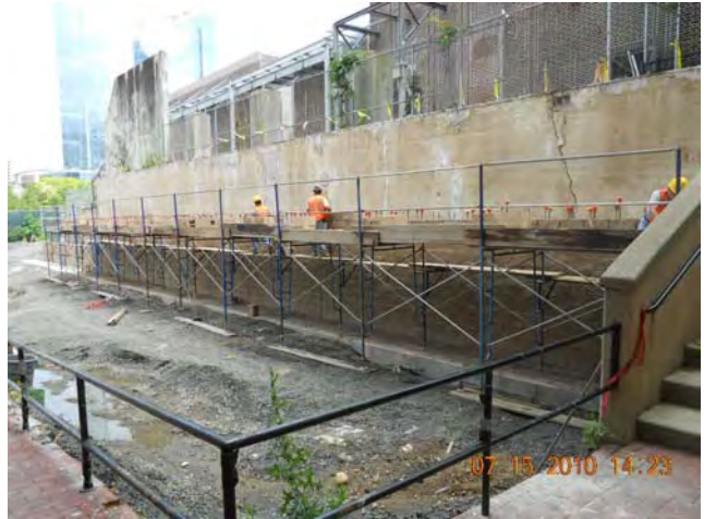
Site Restoration – Planter Wall Stucco Reconstruction Final Masonry Courses July 15, 2010
