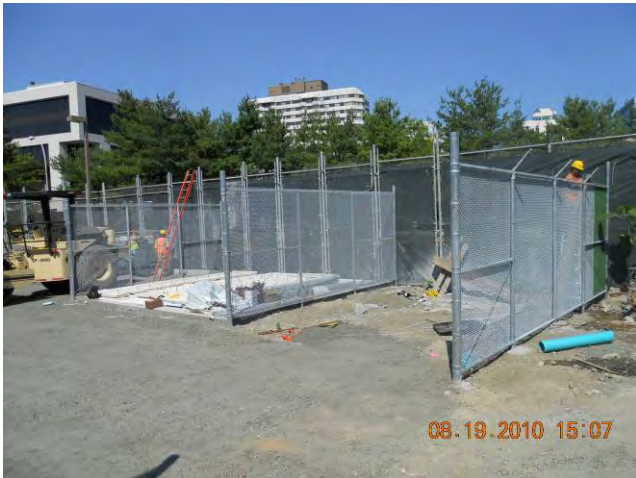
Site Restoration – Fence Installation Fence Fabric Installed onto Dumpster Pad Fence Posts August 19, 2010
