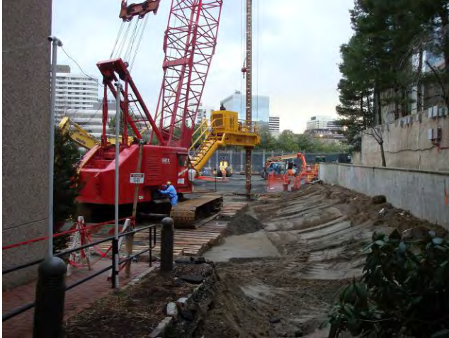
Auger ISS – Test Column Installation Auger Rig Set-up on Test Column Location M-10 March 30, 2009
