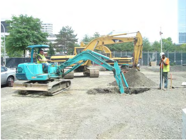
Site Restoration – Lighting Excavation for Light Pole Base Construction July 16, 2010
