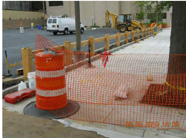
Site Restoration – Fence Installation Completed Guide Rail August 25, 2010
