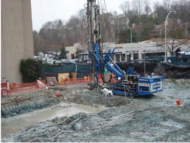
Jet Grouting – Column Installation Activities Installing Jet Grout Column WO-5 December 15, 2009
