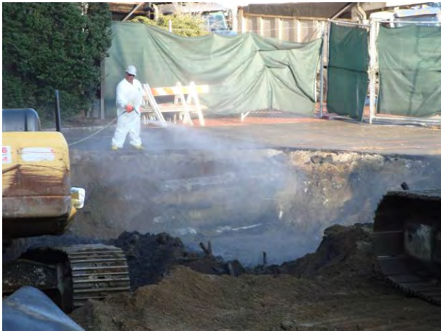
Demo of Structures for West Side BioSolve Sprayed to Reduce Odors March 27, 2009
