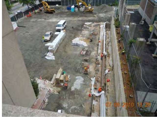
Site Restoration – Planter Wall Stucco Reconstruction Initial Masonry Courses July 8, 2010
