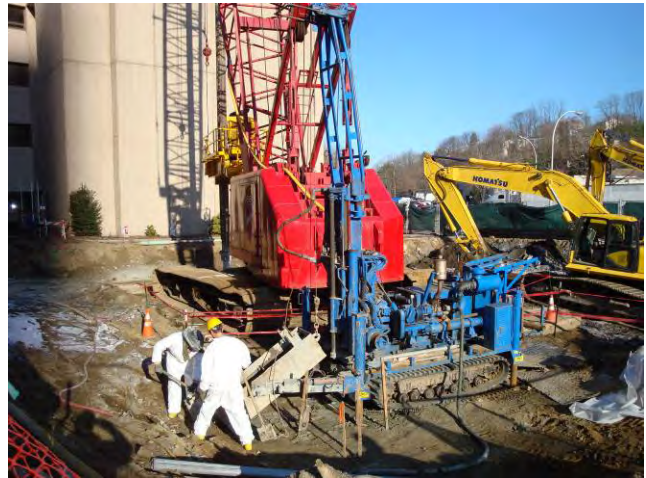
Auger ISS - Test Coring Program Drill rig (CME-55) for Test Core Sampling April 9, 2009
