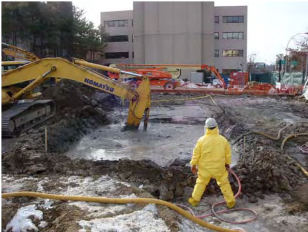
Excavator ISS – Cell Mixing Excavator Mixing Test Cell TP-2 January 27, 2009
