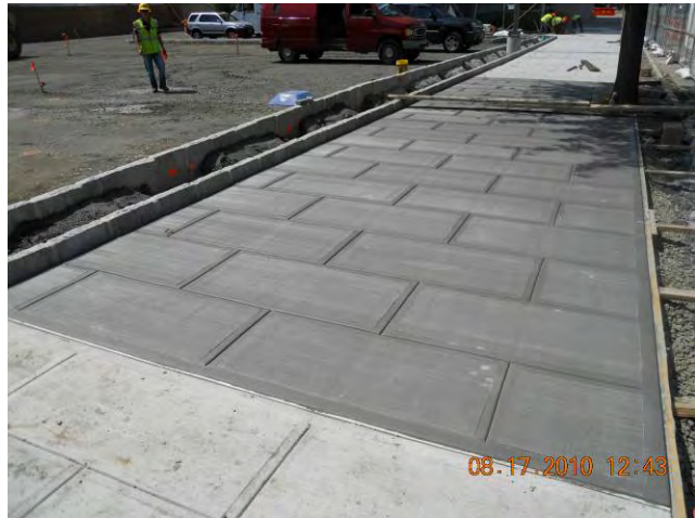
Site Restoration – Sidewalk Construction Finished Sidewalk Section August 17, 2010
