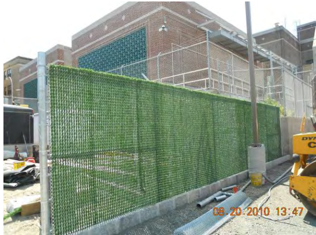
Site Restoration – Fence Installation Privacy Screen Installed over Fence Fabric August 20, 2010
