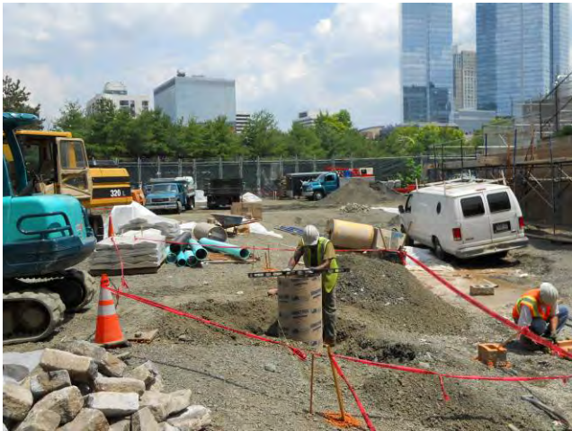
Site Restoration – Lighting Leveling Light Pole Base Form July 29, 2010
