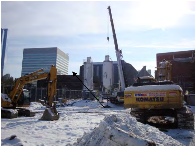
ISS - Mobilization Crane Placing Portland Silo January 20, 2009
