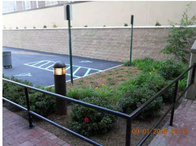
Site Restoration – Plantings Completed Plantings in Alcove Area September 1, 2010
