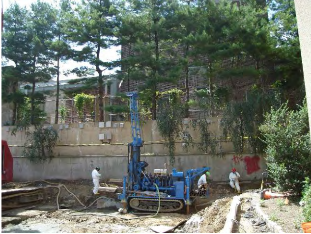
Jet Grouting – Test Cores Collecting ISS Core from Test Column JG-Test-6 July 10, 2009
