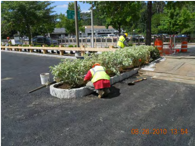
Site Restoration – Plantings Plantings Near East Entrance Drive August 26, 2010
