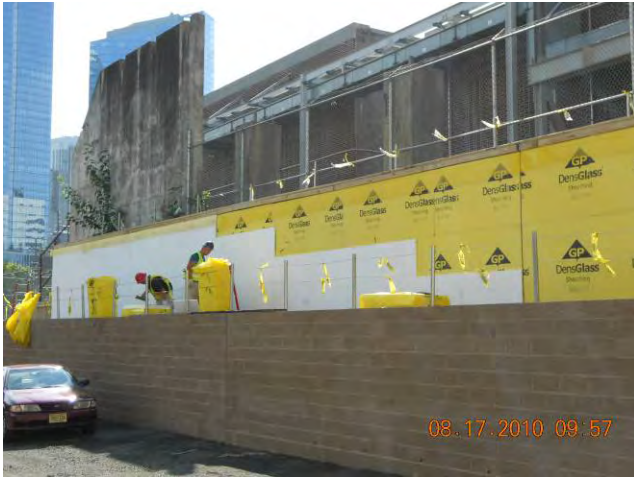
Site Restoration – Retaining Wall Insulation Board Placed over Dens Glass August 17, 2010
