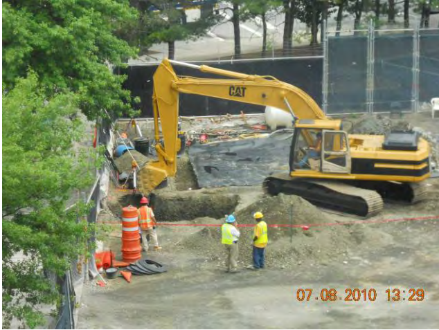
Site Restoration – Hydrodynamic Separators Excavating for Hydrodynamic Separator CB-2 July 8, 2010
