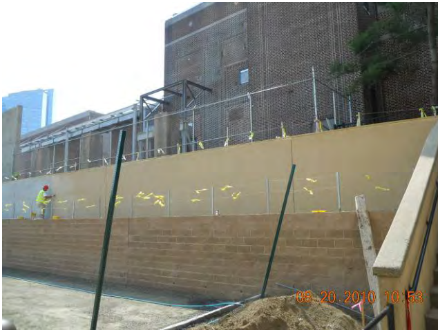
Site Restoration – Retaining Wall Application of Final Stucco Finish August 20, 2010
