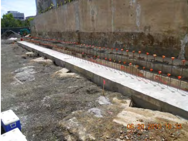
Site Restoration – Planter Wall Stucco Reconstruction Concrete Footing June 28, 2010
