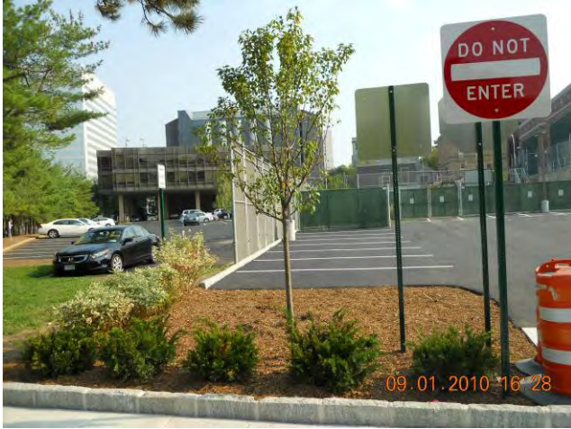
Site Restoration – Plantings Completed Plantings at Northeast Corner September 1, 2010
