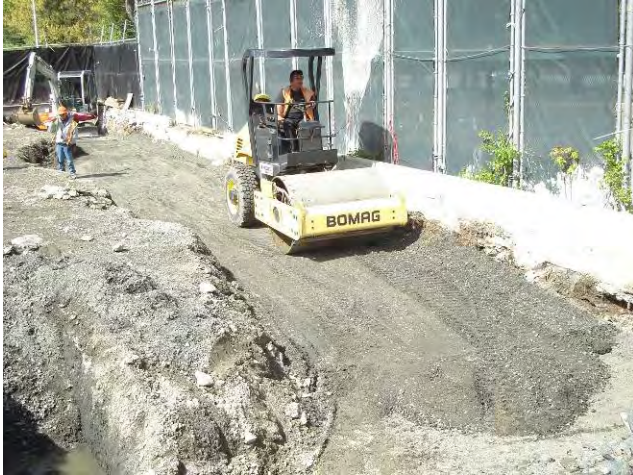
Site Restoration – Backfill Compacting Backfill Along East Perimeter of Site April 27, 2010
