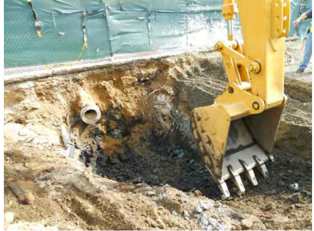
Site Restoration – Hydrodynamic Separators Excavation for Hydrodynamic Separator CB-2 July 8, 2010
