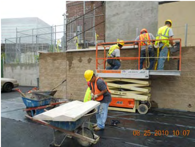
Site Restoration – Planter Wall Stucco Reconstruction Concrete Cap Installation August 25, 2010
