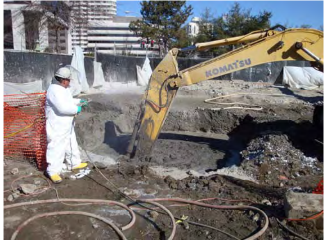
Excavator ISS – Cell Mixing Excavator Mixing Test Cell EM-9 February 24, 2009
