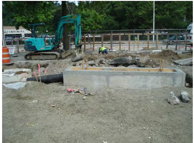
Site Restoration – Trench Drains Concrete Forms Removed from Trench Drain CB-2 August 11, 2010
