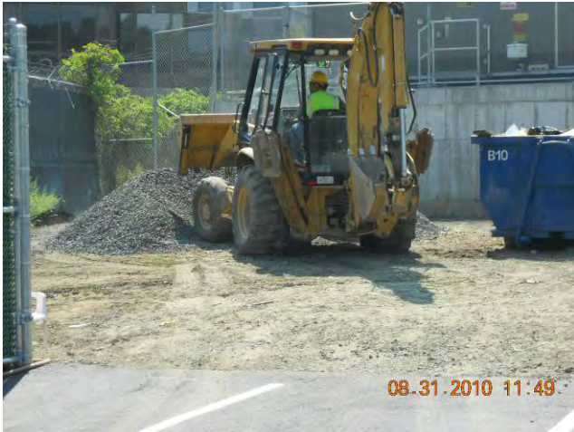
Site Restoration – Substation area (ISS Staging Area) Spreading Crushed Stone Layer August 31, 2010
