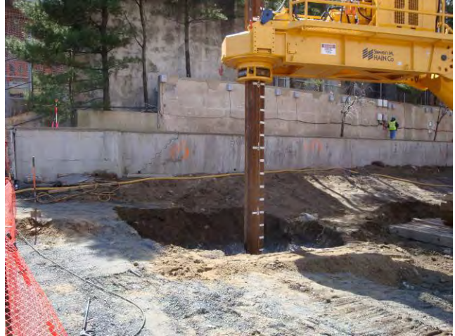
Auger ISS – Test Column Installation Auger Rig Mixing Test Column M-10 March 30, 2009
