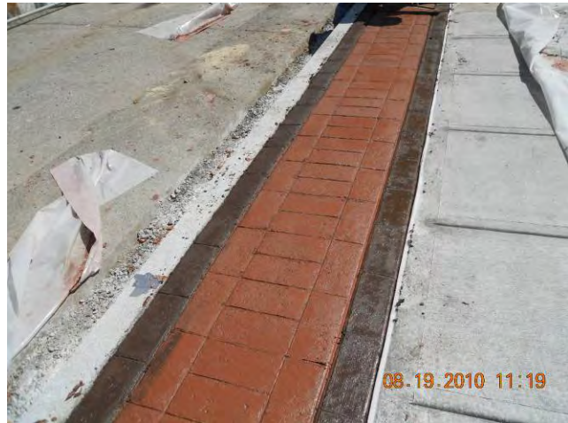
Site Restoration – Sidewalk Construction Completed Stamped Concrete August 19, 2010
