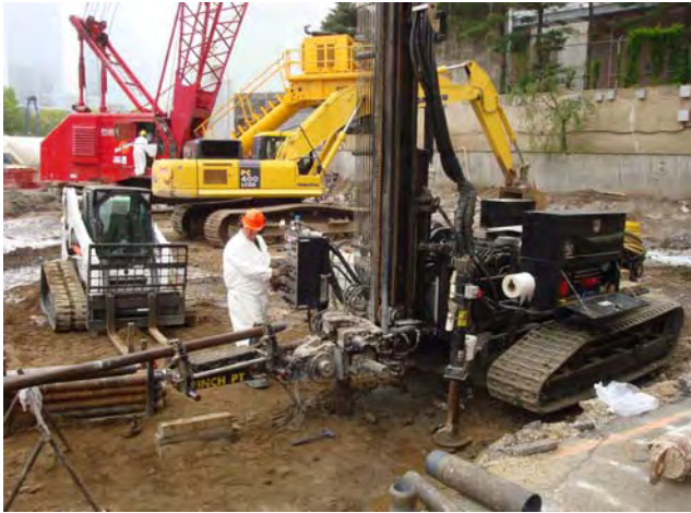
Excavator ISS – Delineation Borings Rotasonic Drilling May 16, 2009
