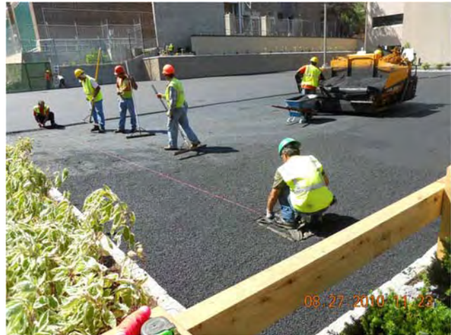
Site Restoration – Asphalt Placement Placement of Top Course and Checking Grade August 27, 2010
