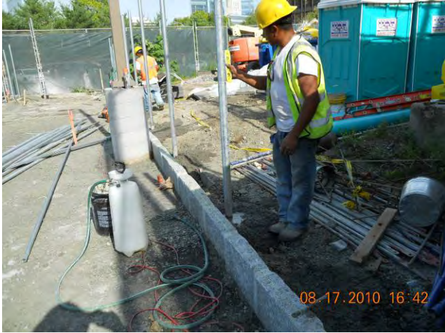
Site Restoration – Fence Installation Installing Fence Posts into Concrete along South Perimeter August 17, 2010
