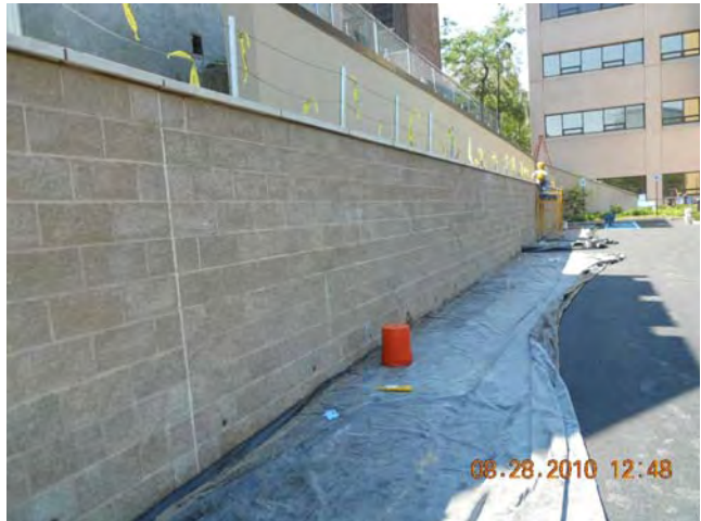
Site Restoration – Planter Wall Stucco Reconstruction Completed Planter Wall August 28, 2010
