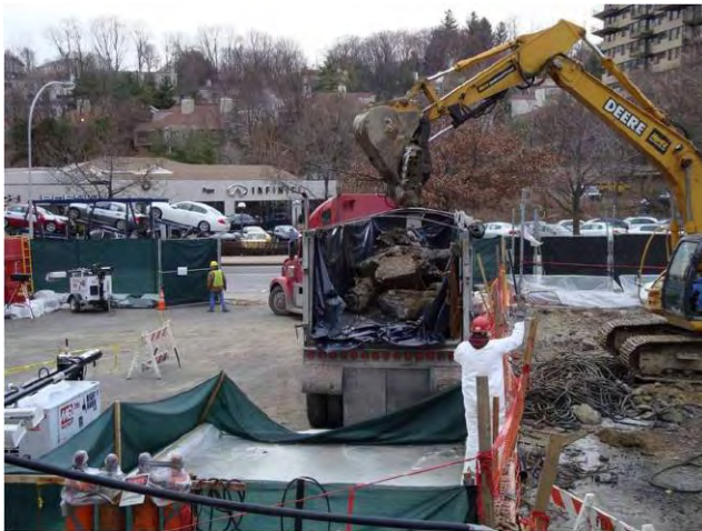
Switchyard Demo & Asbestos Abatement Loading C&D Material for Off-site Disposal December 9, 2008
