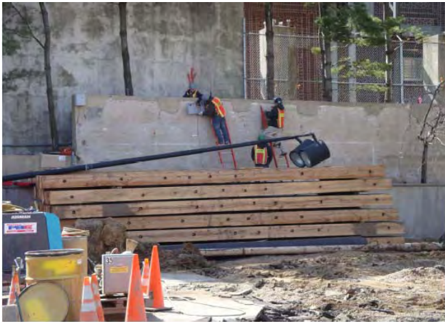
Instrumentation & Monitoring Installation of Tiltmeters March 25, 2009
