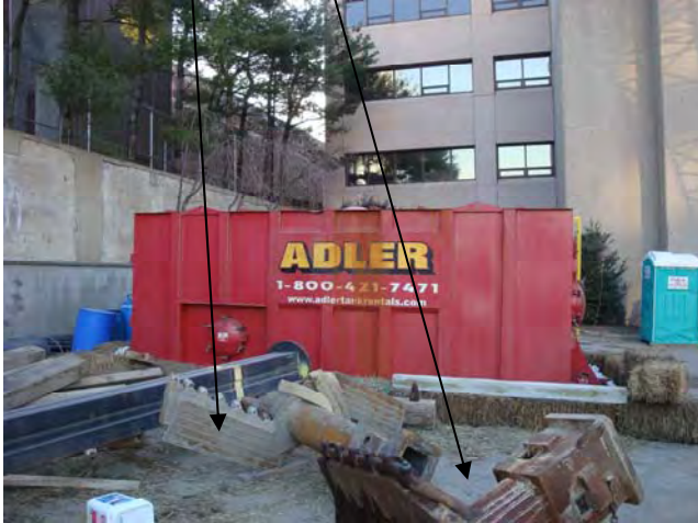
Auger ISS – Various Auger Sizes 9-foot and 8-foot Diameter Augers February 25, 2009
