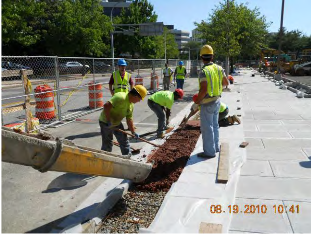
Site Restoration – Sidewalk Construction Concrete Pour for Stamped Concrete August 19, 2010
