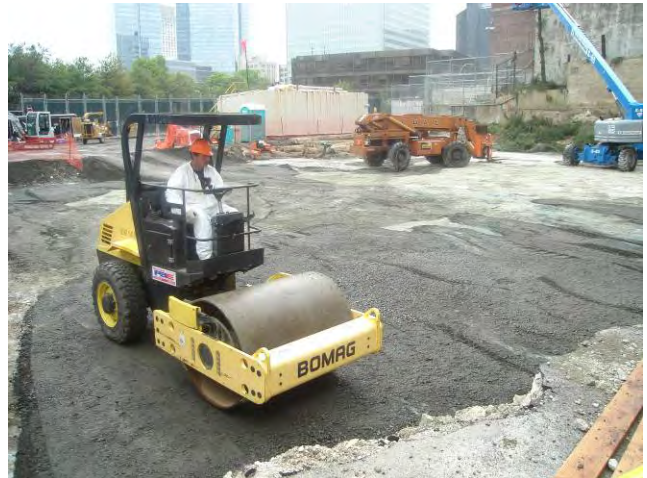
Site Restoration –Backfill Compacting Backfill in Northwest Corner of Site May 15, 2010
