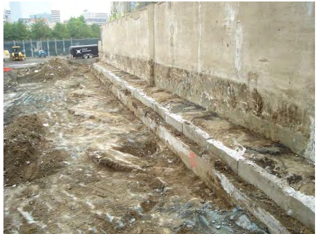
Site Restoration – Retaining Wall Forms removed from Cellular Concrete Pour June 14, 2010
