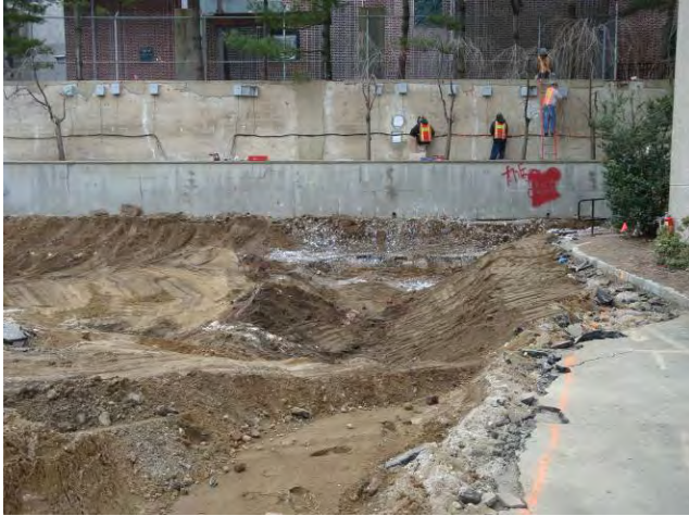
Demo of Structures for West Side Excavated Pavement and Substructures March 26, 2009
