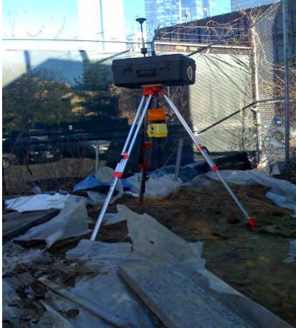
Instrumentation & Monitoring CAMP Station February 13, 2009
