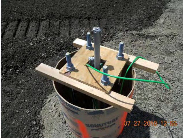
Site Restoration – Lighting Anchor Bolts and Conduits Placed in Light Pole Base Form July 27, 2010
