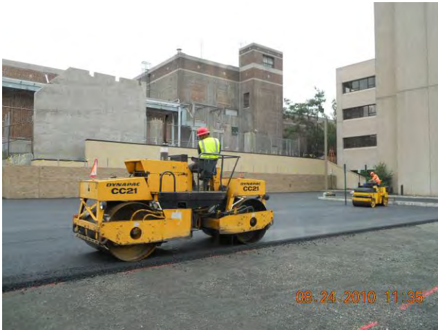
Site Restoration – Asphalt Placement Compacting Asphalt Base Course August 24, 2010
