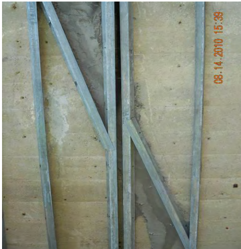
Site Restoration – Retaining Wall Stucco Installation Z-stud Installation Over Crack #11 August 14, 2010
