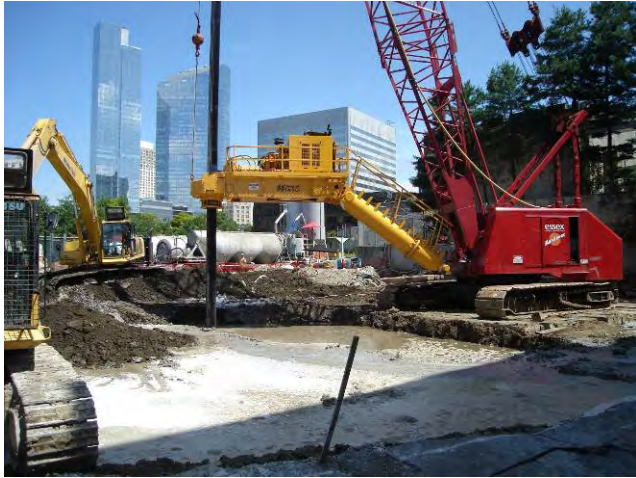
Auger ISS – Drilling Activities Auger Rig Mixing Column 8G5 July 9, 2009
