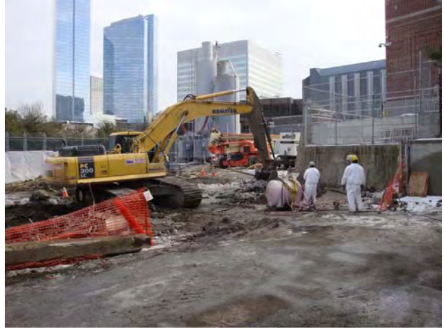
Excavator ISS – Cell Mixing Excavator Mixing Cell P-13 February 7, 2009
