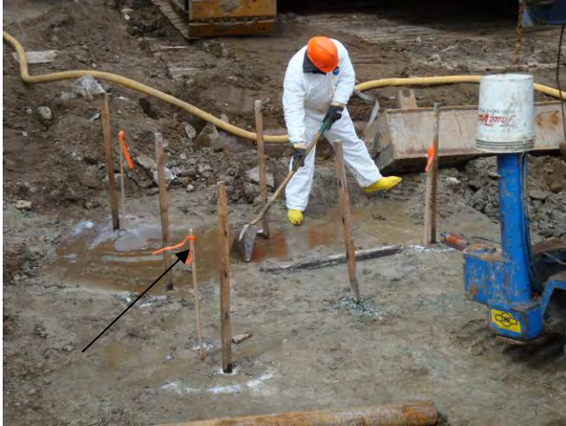
Auger ISS - Test Coring Program Test Core Drill Locations Staked Out April 7, 2009
