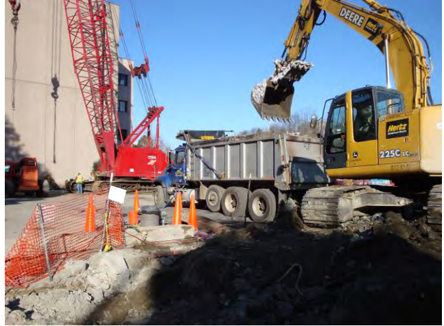
Excavator ISS – Lowering top elevation of ISS Loading ISS Material for Off-site Disposal March 6, 2009
