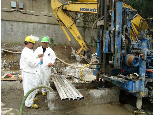
Hot Spot Delineation Borings Preparing to Collect Sample at Location DB-9 April 29, 2009
