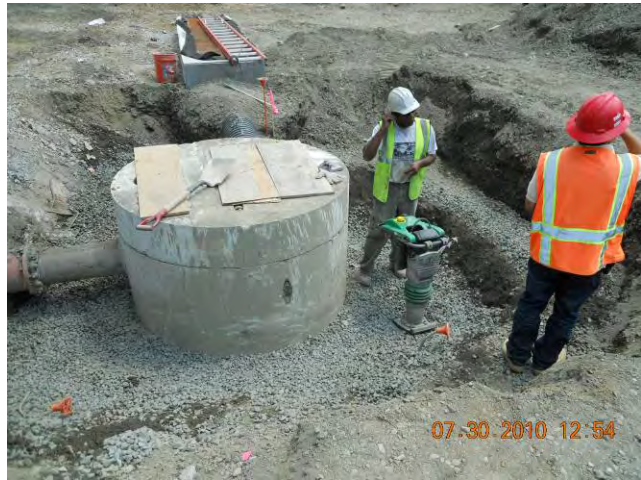
Site Restoration – Hydrodynamic Separator Connections Made to CB-2 Separator July 30, 2010
