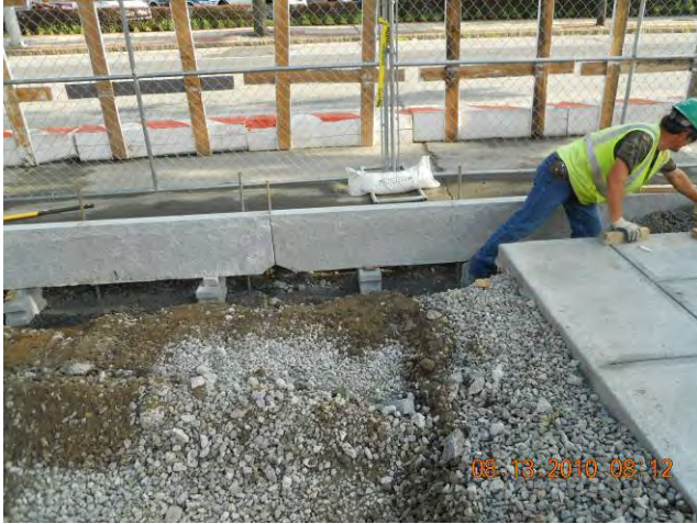
Site Restoration – Curbing New street Curbing prior to Concrete Pour August 13, 2010
