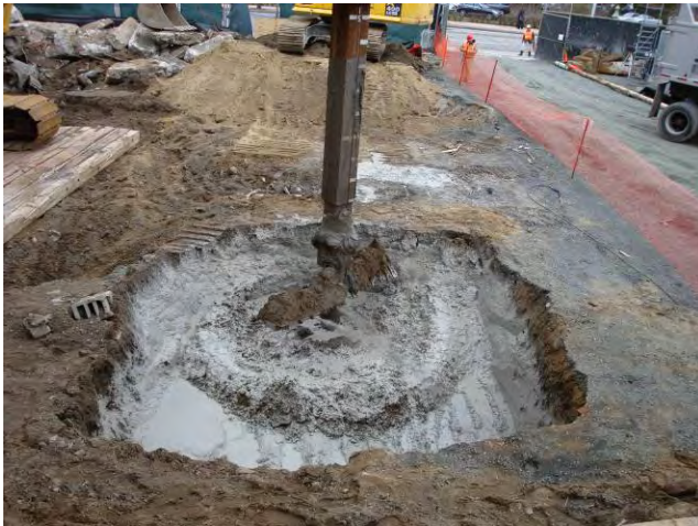
Auger ISS – Test Column Installation Pulling Auger Out of Installed Test Column M-10 March 30, 2009
