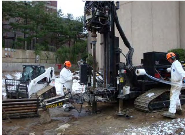
Excavator ISS – Delineation Borings Rotasonic Drilling May 16, 2009
