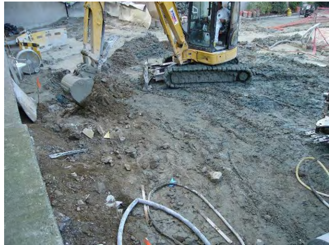
Jet Grouting – Spoils Collection and Load Out Excavating Jet Grout Spoils October 22, 2009
