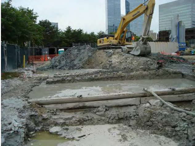
Jet Grouting – Spoils Collection and Load Out Jet Grout Spoils sump Collection Area September 22, 2009
