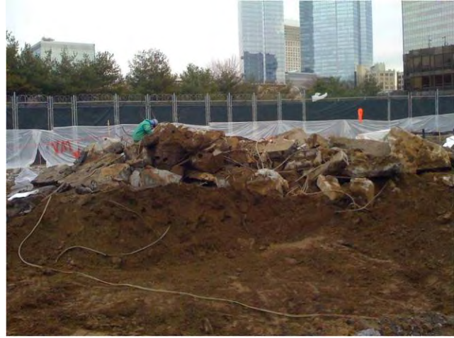
Switchyard Demo & Asbestos Abatement Stockpile of C&D Material December 6, 2008
