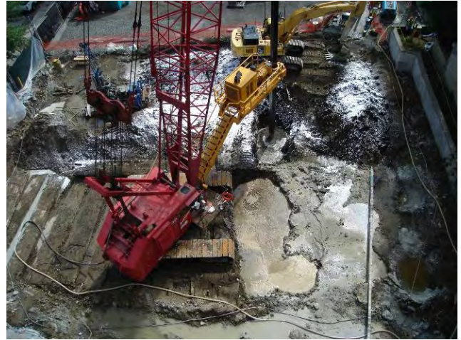
Auger ISS – Drilling Activities Auger Rig Mixing Column 8L4 July 24, 2009
