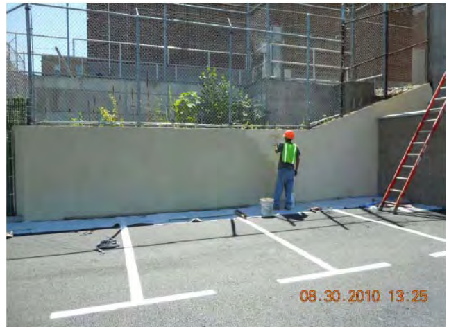
Site Restoration – Lower Substation Wall Second Application of Thorocoat August 30, 2010
