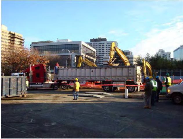
Switchyard Demo & Asbestos Abatement Loading C&D Material for Off-site disposal December 5, 2008
