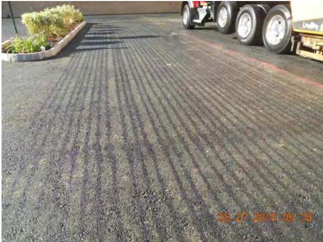
Site Restoration – Asphalt Placement Placement of Tack Coat August 28, 2010
