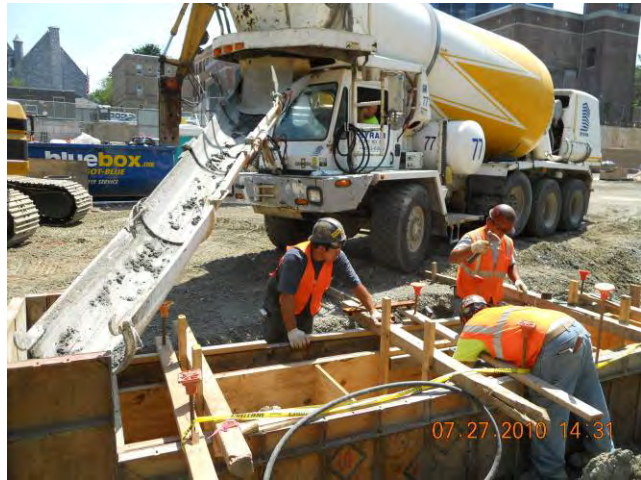
Site Restoration – Trench Drains Concrete pour for Trench Drain CB-2 July 27, 2010
