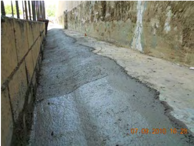
Site Restoration – Planter Wall Stucco Reconstruction Concrete Wash Behind Planter Wall July 9, 2010
