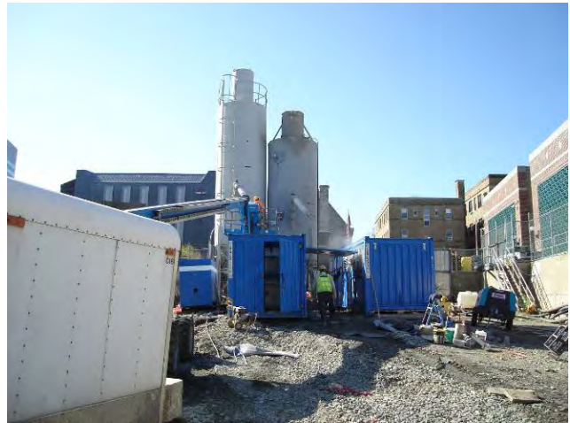
Jet Grouting – Column Installation Activities Jet grout Batch Plant Area April 14, 2010
