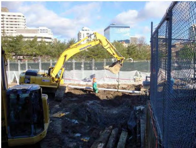
Switchyard Demo & Asbestos Abatement Removal of Subsurface Pipe December 12, 2008
