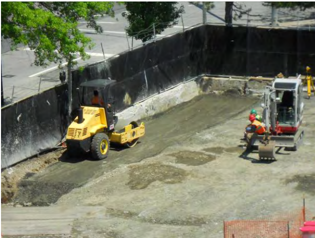
Site Restoration –Backfill Compacting Backfill Along North Perimeter of Site May 5, 2010
