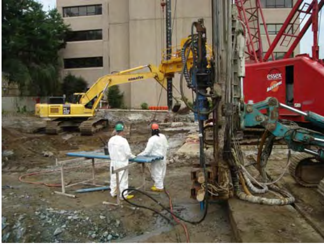
Jet Grouting – Test Column Installation Installation of Jet grout Test Column JG-1 June 26, 2009
