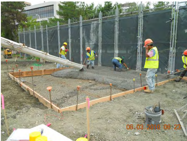
Site Restoration – Dumpster pad construction Concrete Pour for Dumpster Pad August 3, 2010
