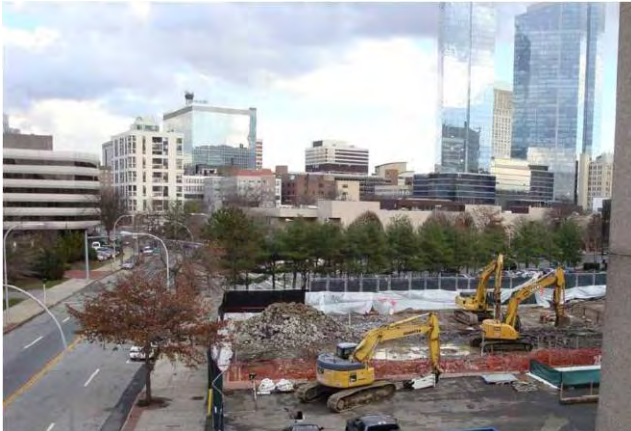
Switchyard Demo & Asbestos Abatement Overhead View of Switchyard Demolition December 1, 2008
