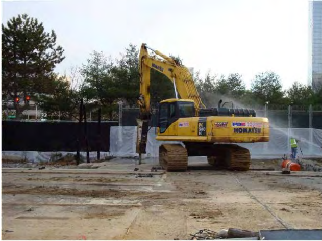
Switchyard Demo & Asbestos Abatement Initial Demo with Hydraulic Hammer November 21, 2008
