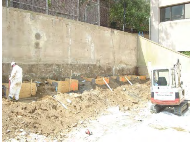
Site Restoration – Voids under Retaining Wall Footing Placing Forms to Fill in Voids June 3, 2010
