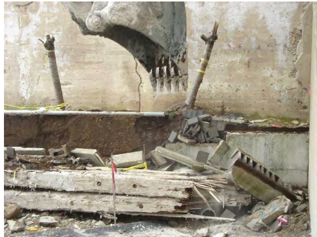
Site Restoration – Planter Wall Demolition Demolishing West Portion of Planter Wall April 6, 2010
