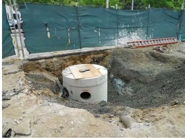
Site Restoration – Hydrodynamic Separator Hydrodynamic Separator CB-1 July 13, 2010
