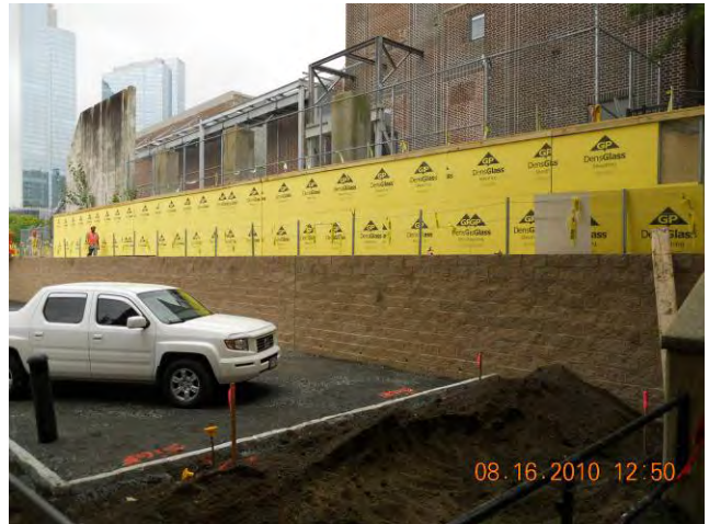
Site Restoration – Retaining Wall Stucco Installation Dens Glass Sheeting Installation August 16, 2010
