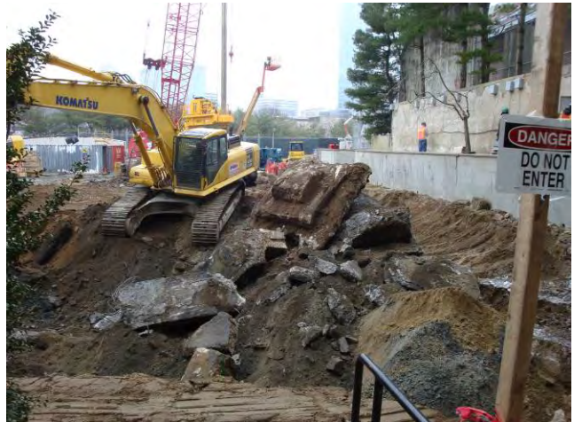
Demo of Structures for West Side Excavated Subsurface Structures March 26, 2009
