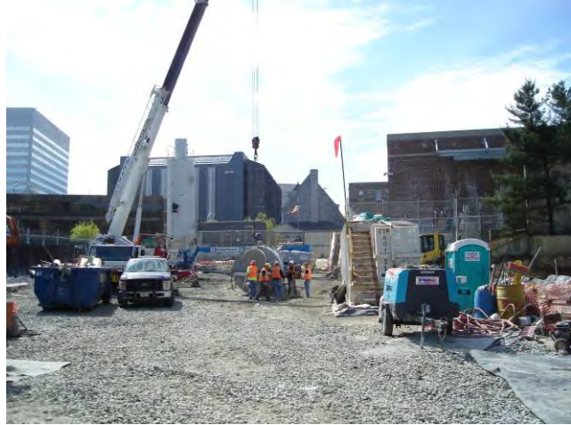
Jet Grouting – Demobilization Dismantling Batch Plant April 15, 2010
