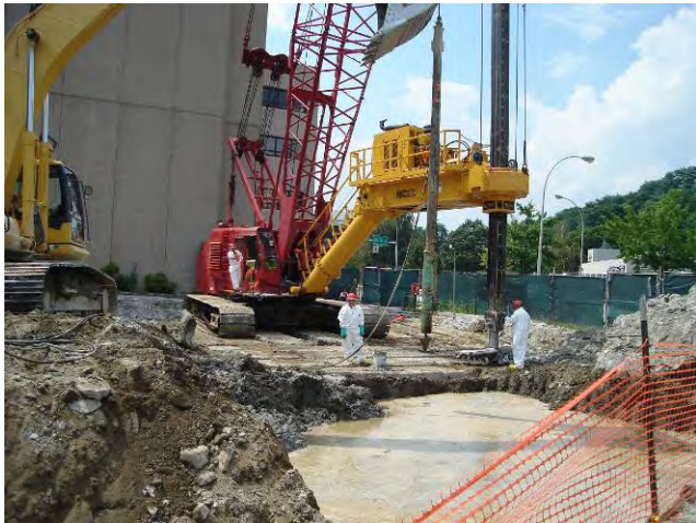
Auger ISS – Sampling Collecting Grout Sample for Column 8x4 July 28, 2009
