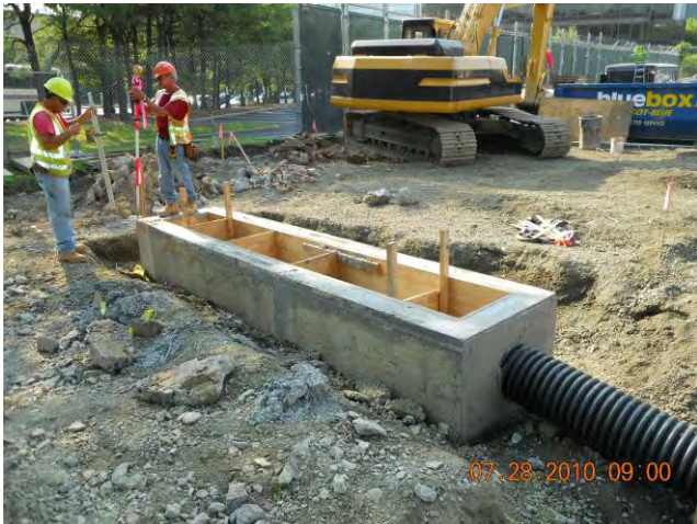
Site Restoration – Trench Drains Concrete Forms Removed from Trench Drain CB-2 July 28, 2010
