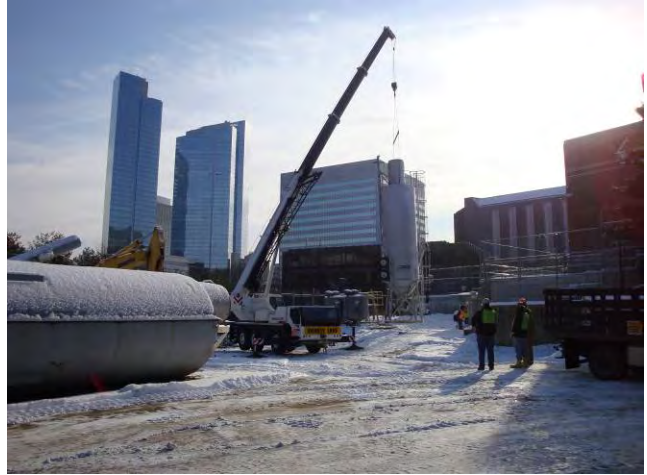
ISS - Mobilization Crane Placing Slag Silo January 20, 2009
