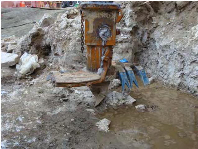
Auger ISS – Various Auger Sizes 4-foot Diameter Auger May 28, 2009
