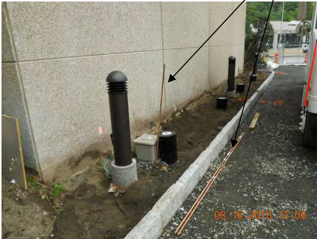
Site Restoration – Lighting Light bollards and Wall Wash Lights and Grounding Rods August 16, 2010
