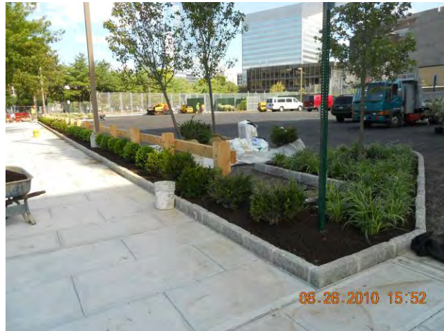
Site Restoration – Plantings Plantings along Water Street Sidewalk August 28, 2010
