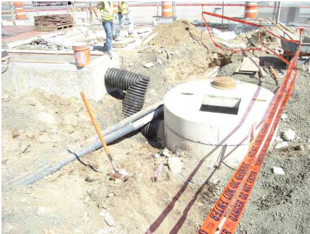
Site Restoration – Hydrodynamic Separator Connection from CB-1 Trench Drain to Separator July 21, 2010
