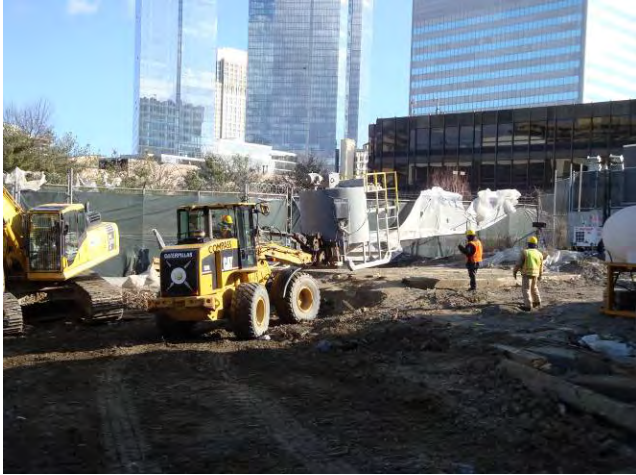
ISS - Mobilization Placing Reagent Mixing Tub January 9, 2009
