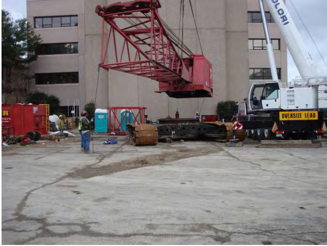
Auger ISS - Mobilization Crane Assembly February 12, 2009
