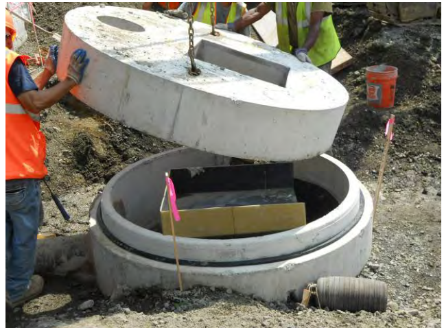
Site Restoration – Hydrodynamic Separators Placing Top of Hydrodynamic Separator CB-1 July 13, 2010
