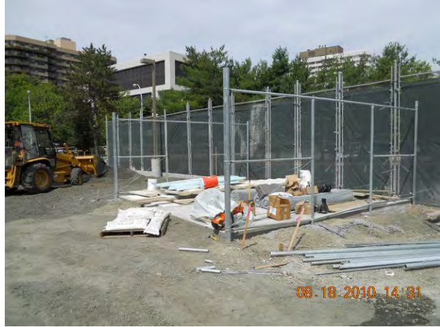
Site Restoration – Fence Installation Fence Post Installation for Dumpster Pad August 18, 2010
