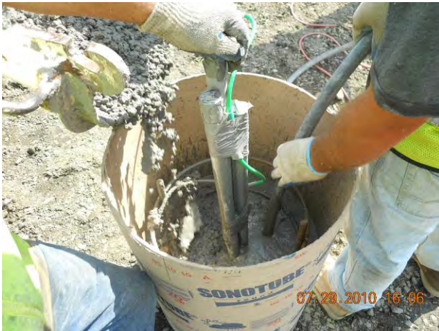
Site Restoration – Lighting Concrete Pour for Light Pole Base July 28, 2010
