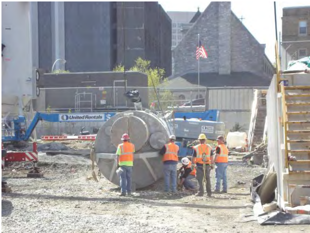
Jet Grouting – Demobilization Laying Down Reagent Silo April 15, 2010
