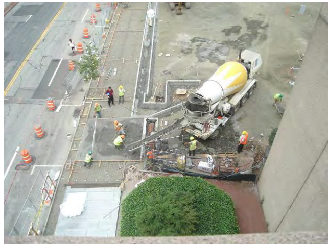
Site Restoration – Entrance Drive Construction Concrete Pour for West Entrance Drive August 10, 2010
