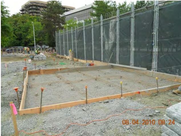
Site Restoration – Dumpster pad construction Forms and Rebar for Dumpster Pad August 4, 2010
