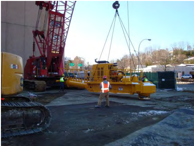
Auger ISS - Mobilization Mounting Drilling Platform to Crane March 3, 2009
