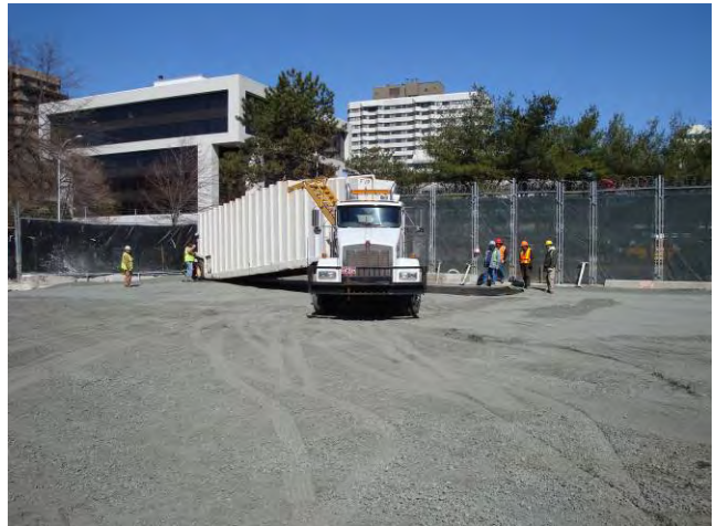
Backfill Placement & Compaction (East Side) Loading Baker Tank on Completed Backfill March 24, 2009
