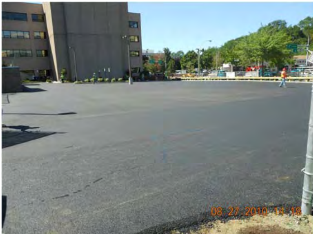
Site Restoration – Asphalt Placement Completed Top Course August 27, 2010
