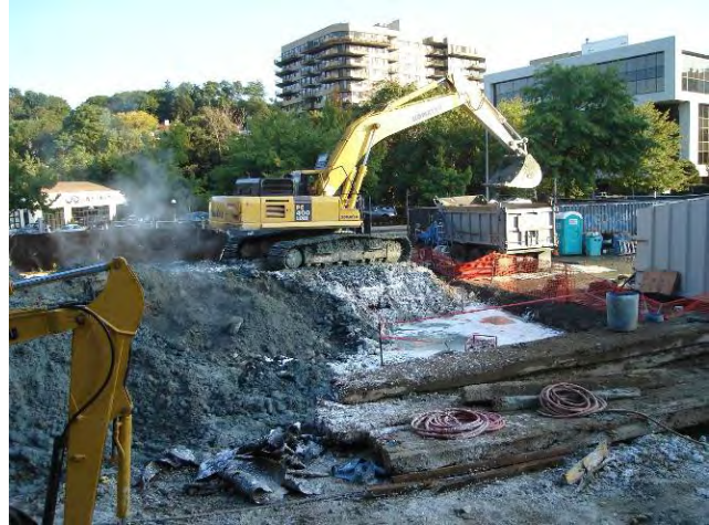
Jet Grouting – Spoils Collection and Load Out Loading Jet Grout Spoils for Off-site Disposal September 29, 2009
