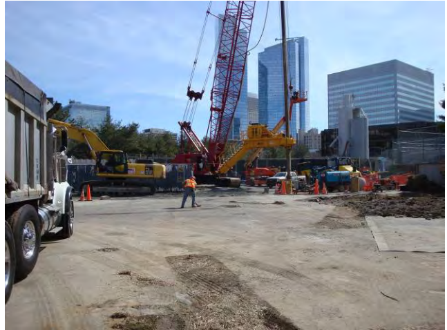
Auger ISS - Mobilization Completed Assembly of Crane and Drilling Platform March 27, 2009
