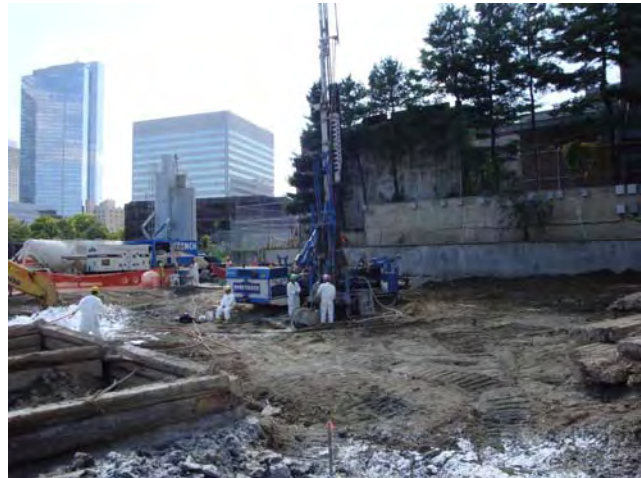
Jet Grouting - Mobilization Setting Up Jet Grout Production Rig August 17, 2009
