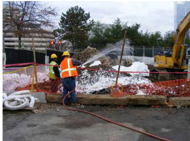
Switchyard Demo & Asbestos Abatement Applying Rusmar Foam for Odor Control December 15, 2008
