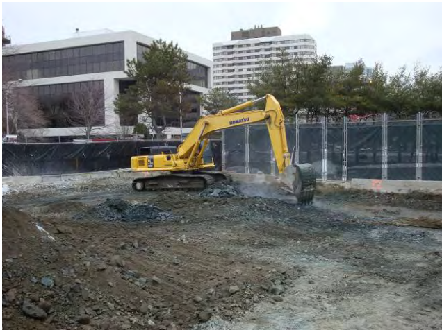
Excavator ISS – Lowering top elevation of ISS Scraping Down Top of ISS Monolith March 6, 2009
