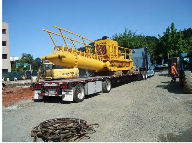
Auger ISS – Demobilization Drilling Platform Loaded onto Truck August 8, 2009
