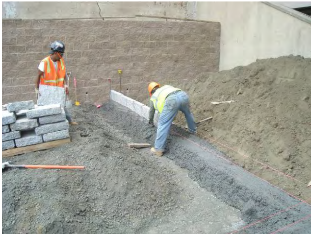
Site Restoration – Curbing Placing granite Block Curb in Southwest corner August 5, 2010
