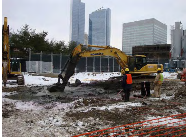
Excavator ISS – Test Cell Mixing Excavator Mixing Test Cell TP-1 January 22, 2009
