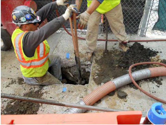
Sidewalk Borings Hand clearance for SW-5 May 11, 2010
