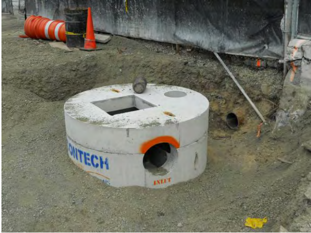
Site Restoration – Hydrodynamic Separator Hydrodynamic Separator CB-2 July 13, 2010
