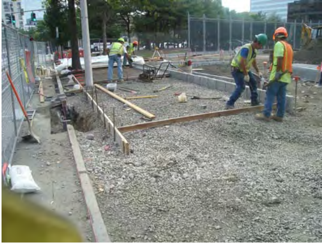
Site Restoration – Sidewalk Construction Concrete forms for Sidewalk Sections August 6, 2010
