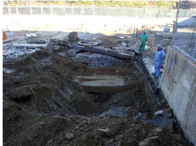
Switchyard Demo & Asbestos Abatement Excavation of Switchyard Foundation December 3, 2008
