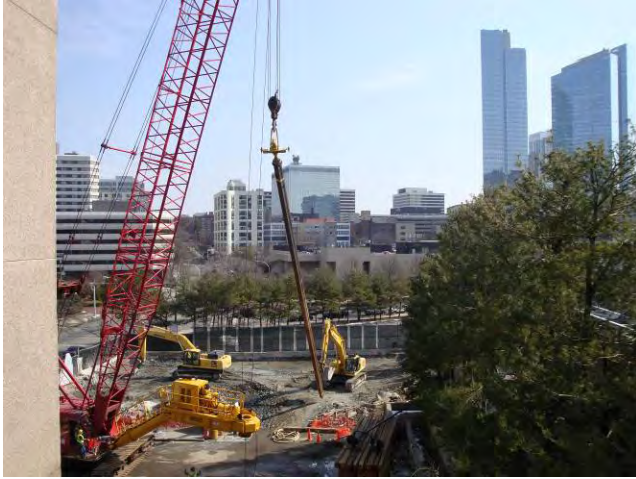
Auger ISS - Mobilization Attaching Kelly Bar to Drilling Platform March 26, 2009
