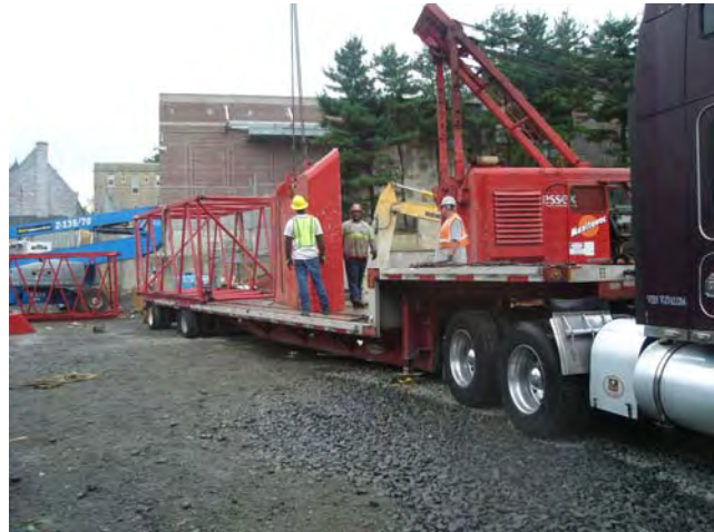
Auger ISS - Demobilization Dismantling of Crane August 12, 2009
