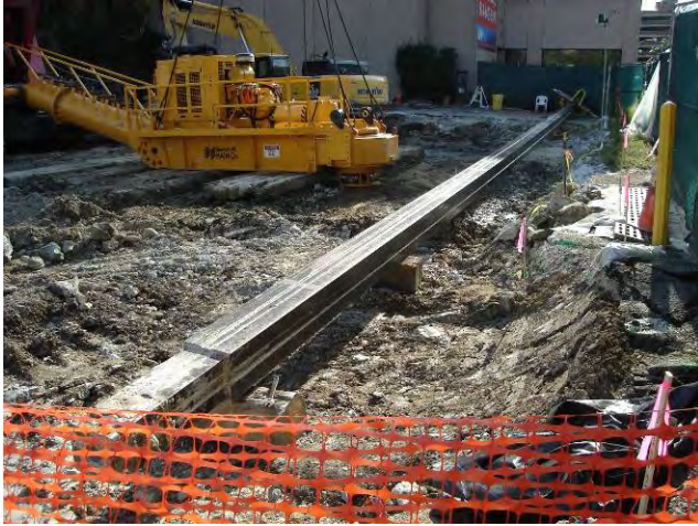
Auger ISS – Demobilization Disassembled Drilling Platform & Kelly bar August 8, 2009
