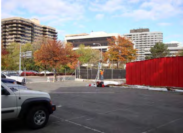
Pre-Remediation Site Conditions Removal of Previous Fencing October 29, 2008
