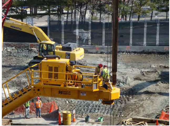
Auger ISS - Mobilization Attaching Kelly Bar to Drilling Platform March 27, 2009
