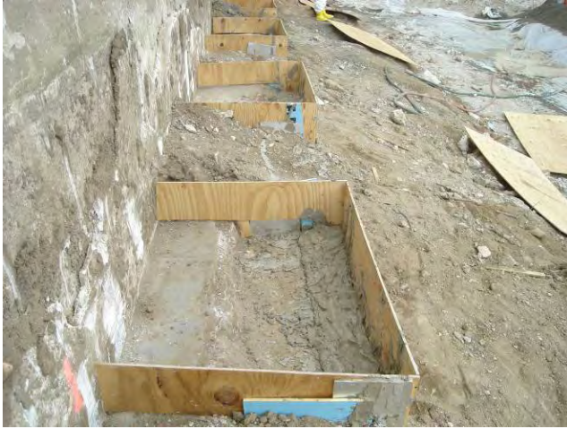
Site Restoration – Retaining Wall Forms Filled with Cellular Concrete June 7, 2010
