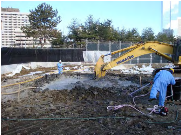
Excavator ISS – Test Cell Mixing Excavator Mixing Test Cell TP-1 (remix) January 26, 2009
