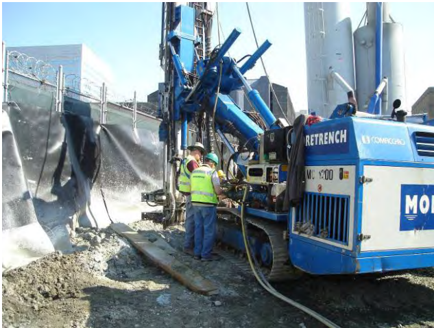
Jet Grouting – Column Installation Activities Installing Jet Grout Column EI-21 April 5, 2010
