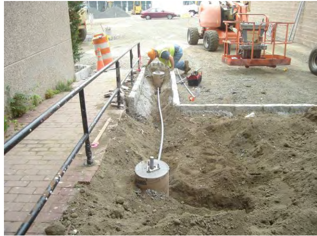
Site Restoration – Lighting Conduit run Between Light Bollard Bases August 16, 2010
