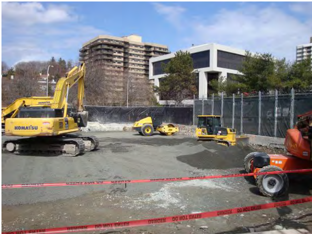
Backfill Placement & Compaction (East Side) Compacting Item #4 Backfill Material March 24, 2009
