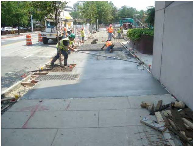
Site Restoration – Sidewalk Construction Concrete Finishing for Sidewalk Section August 17, 2010
