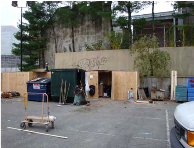
Pre-Remediation Site Conditions South Side of Parking Lot November 2, 2008
