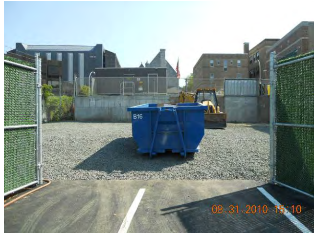
Site Restoration – Substation area (ISS Staging Area) Crushed Stone Layer Placed in Substation Area August 31, 2010
