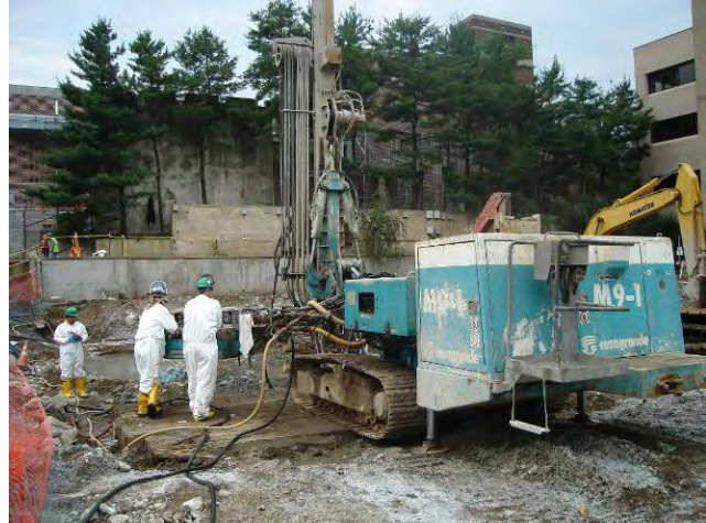
Jet Grouting - Mobilization Test Column Jet Grout Rig Set-up for Test Column June 29, 2009
