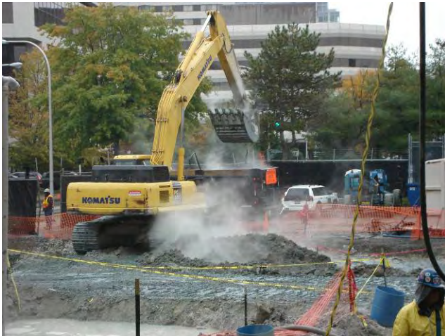
Jet Grouting – Spoils Collection and Load Out Loading Jet Grout Spoils for Off-site Disposal October 15, 2009
