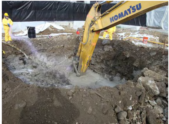
Excavator ISS – Test Cell Mixing Excavator Mixing Test Cell TP-2 January 27, 2009
