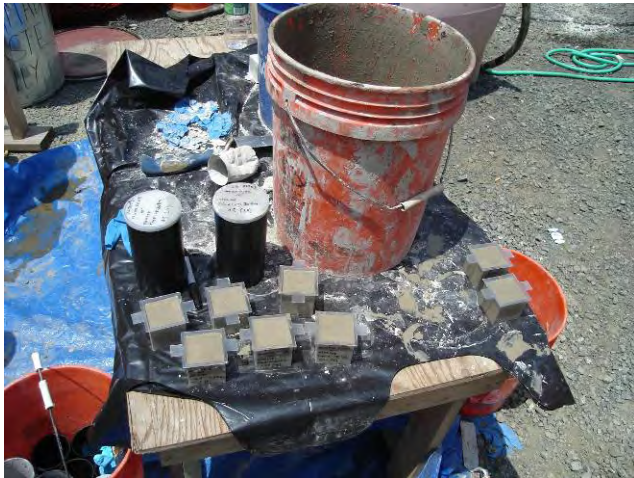
Jet Grouting – Sampling Grout Cylinders and Grout Cubes July 29, 2009
