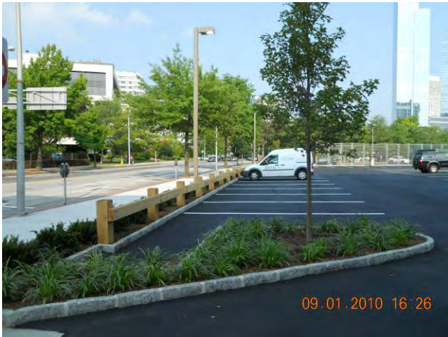
Site Restoration – Plantings Completed Plantings Along 12 Water Street Sidewalk September 1, 2010
