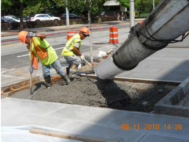
Site Restoration – Sidewalk Construction Concrete Pour for Sidewalk Section August 11, 2010
