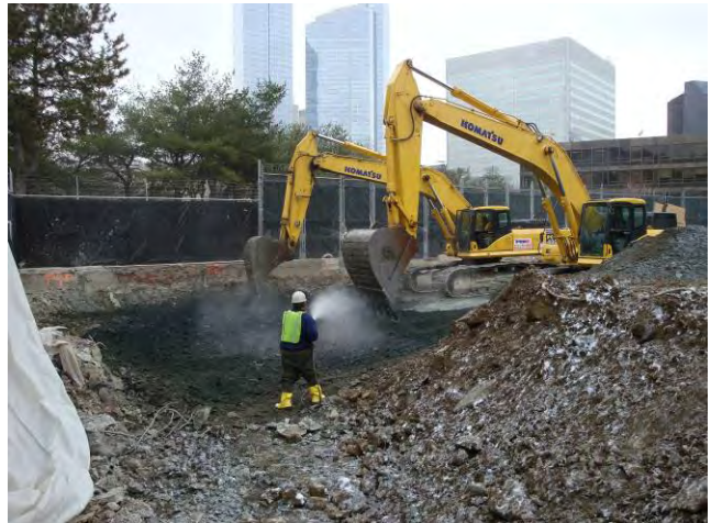
Excavator ISS – Lowering top elevation of ISS Scraping Down Top of ISS Monolith March 11, 2009
