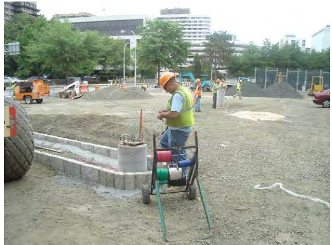
Site Restoration – Lighting Wiring Electrical Connections at Light Pole Base August 21, 2010
