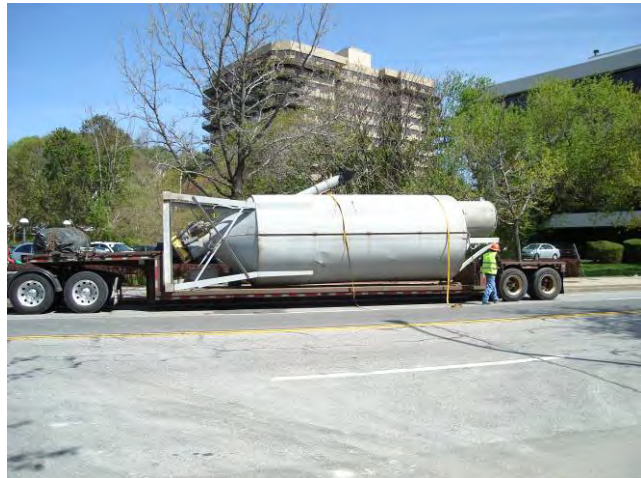
Jet Grouting – Demobilization Reagent Silo Loaded onto Truck April 15, 2010
