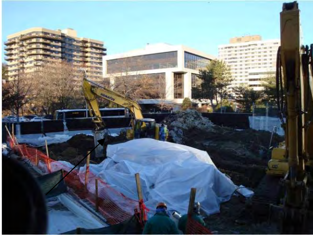
Switchyard Demo & Asbestos Abatement Removal of ACM Duct Banks December 13, 2008
