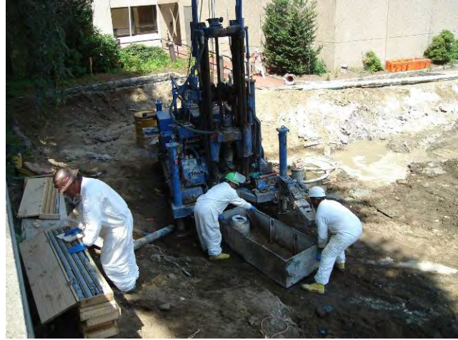
Jet Grouting – Test Cores Observing ISS Core from Test Column JG-Test-6 July 11, 2009
