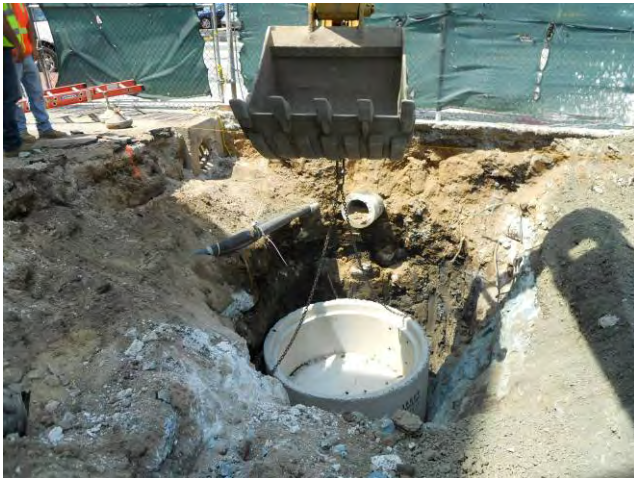
Site Restoration – Hydrodynamic Separators Lowering Base of Hydrodynamic Separator CB-2 July 8, 2010
