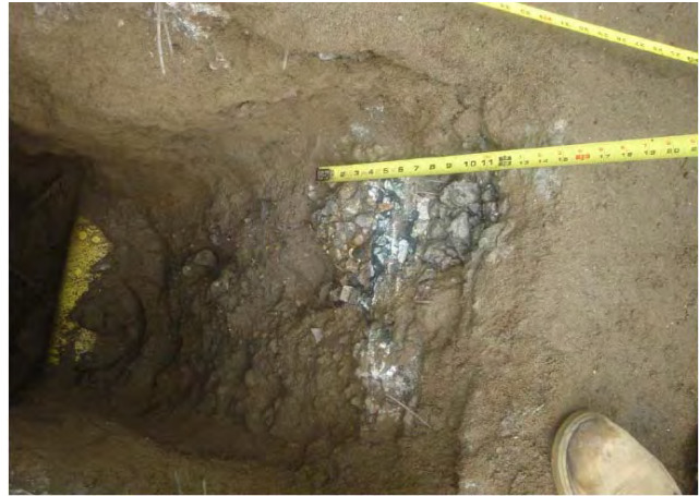
Sidewalk Borings Grout Observed in Sidewalk Sub-base in Hand Clearance for SW-4 May 12, 2010
