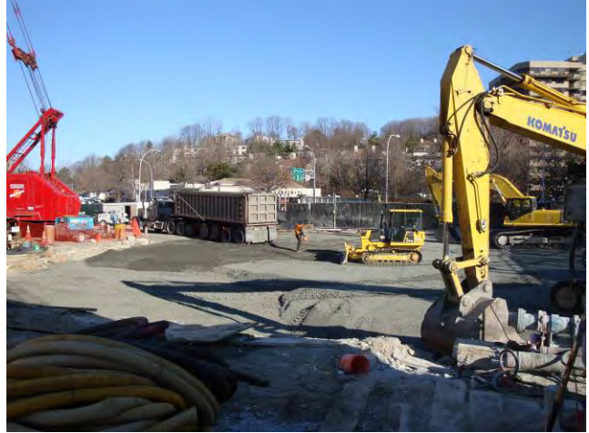
Backfill Placement & Compaction (East Side) Spreading Item #4 Backfill Material March 24, 2009
