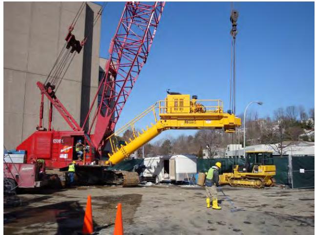
Auger ISS - Mobilization Mounting Drilling Platform to Crane March 4, 2009
