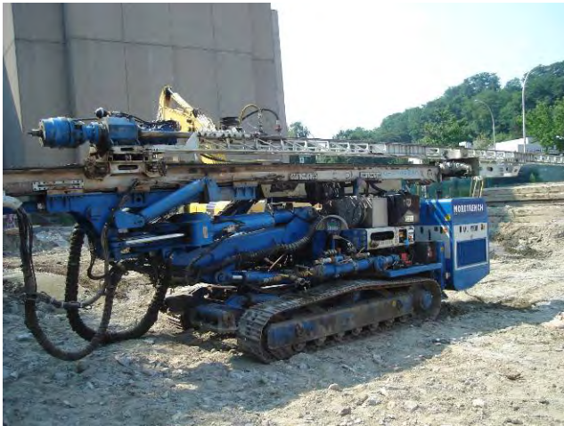
Jet Grouting - Mobilization Production Jet grout Rig Arrived On-site August 17, 2009
