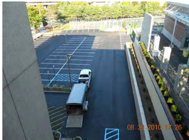
Site Restoration – Southern Area View Looking East August 30, 2010
