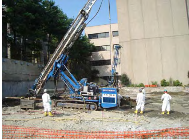
Jet Grouting – Column Installation Activities Jet grout production Rig (Amco Vega Comacchio MC 1200) August 18, 2009
