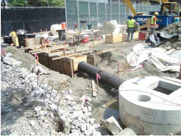
Site Restoration – Trench Drains Forms for Trench Drain CB-2 July 22, 2010
