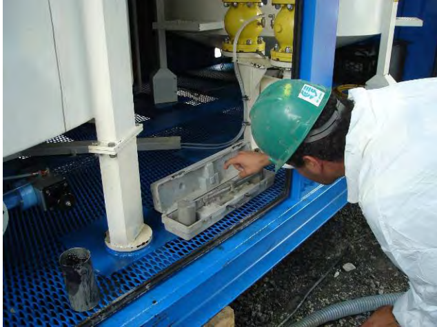
Jet Grouting – Sampling Measuring Grout Density with Mud Balance July 26, 2009
