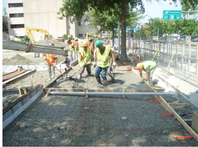
Site Restoration – Entrance Drive Construction Concrete Pour for East Entrance Drive August 5, 2010
