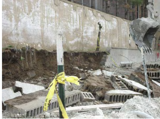
Site Restoration – Planter Wall Demolition Demolishing Central Portion of Planter Wall April 6, 2010
