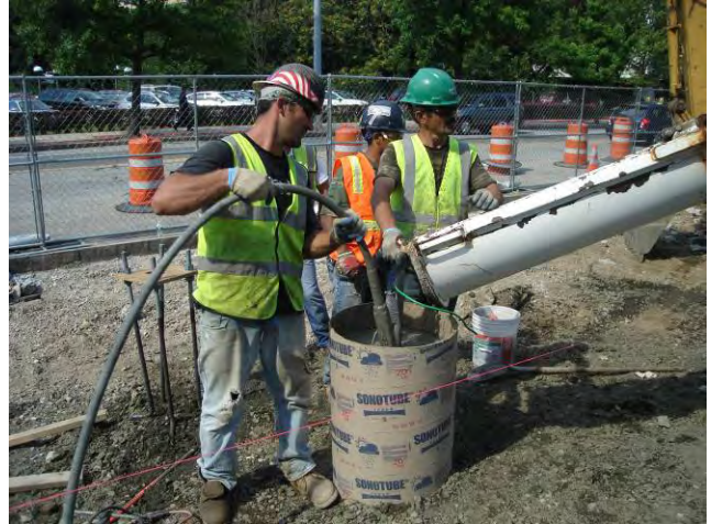
Site Restoration – Lighting Concrete Pour for Light Pole Base July 29, 2010
