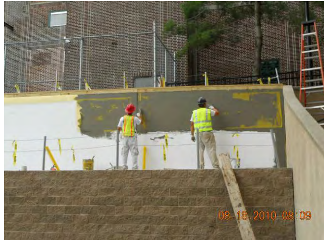
Site Restoration – Retaining Wall Application of Final Stucco Finish August 18, 2010
