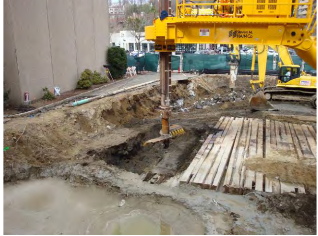
Auger ISS – Drilling Activities Auger Rig Setup on Column Location M-3 April 7, 2009
