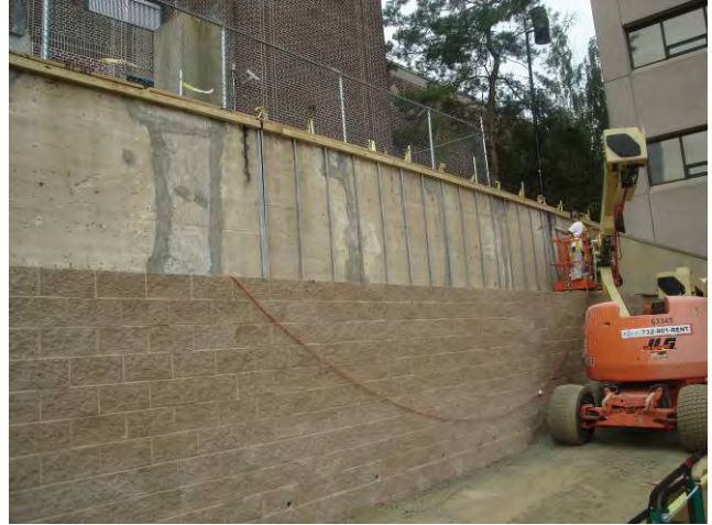
Site Restoration – Retaining Wall Stucco Installation Z-stud Installation Over Crack #4 August 14, 2010
