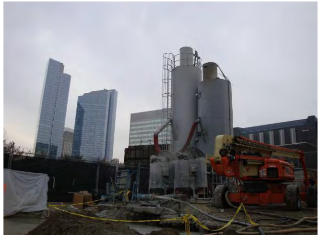
ISS - Mobilization Batch Plant Setup Complete January 27, 2009
