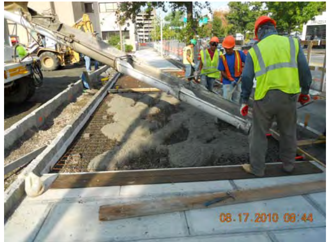
Site Restoration – Sidewalk Construction Concrete Pour for Sidewalk Section August 17, 2010
