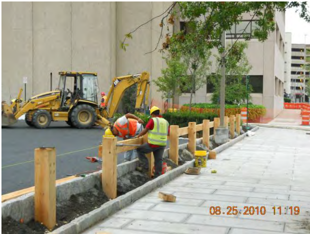
Site Restoration – Fence Installation Installing Rail Portion of Guide Rail August 25, 2010
