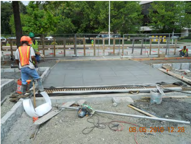
Site Restoration – Entrance Drive Construction Complete Pour for East Entrance Drive August 5, 2010
