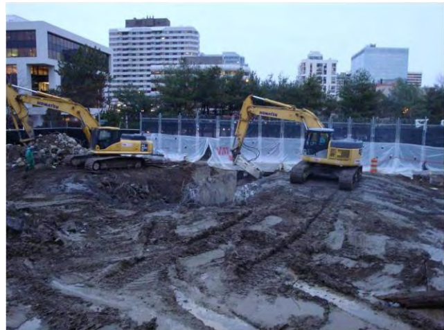
Switchyard Demo & Asbestos Abatement Removal of Switchyard Foundation Elements December 16, 2008
