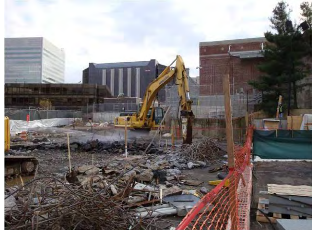
Switchyard Demo & Asbestos Abatement Demo of Surface Concrete Layer November 26, 2008
