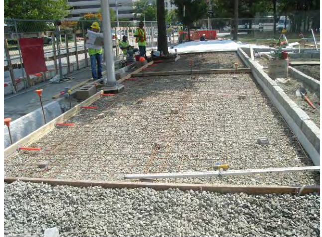
Site Restoration – Sidewalk Construction Concrete Forms and Rebar for Sidewalk Sections August 6, 2010
