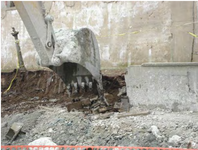
Site Restoration – Planter Wall Demolition Demolishing West Central Portion of Planter Wall April 6, 2010
