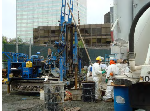
Excavator ISS – Delineation Borings Collecting ISS Core Samples May 14, 2009
