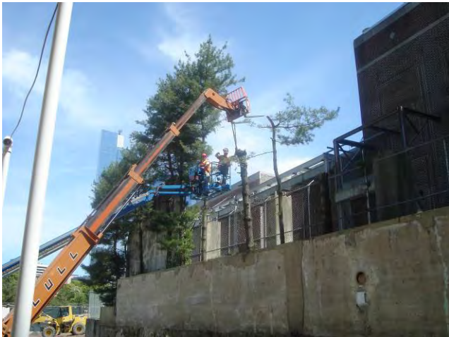
Site Restoration – Tree Removal along Retaining Wall Removing Trees Along Substation Retaining Wall May 13, 2010
