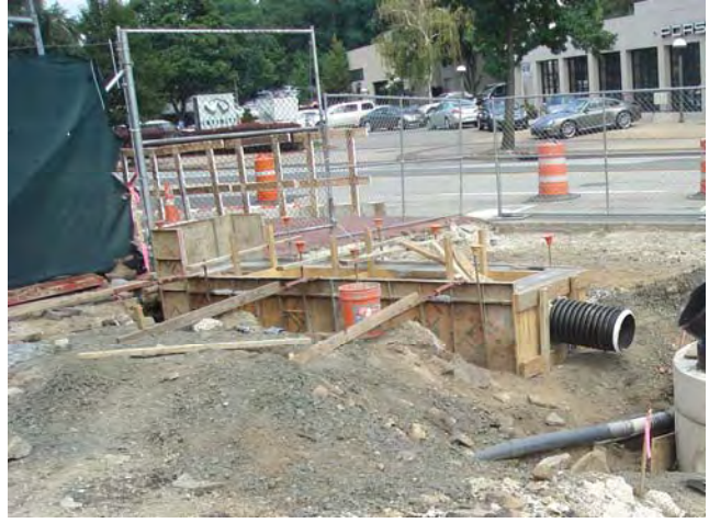
Site Restoration – Trench Drains Concrete Poured for Trench Drain CB-1 July 28, 2010
