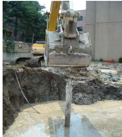
Auger ISS – Sampling Collecting Grout Sample for Column 8x4 July 28, 2009
