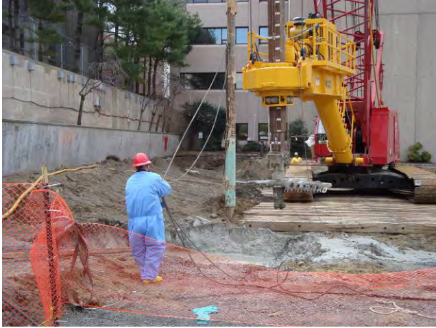
Auger ISS – Sampling Collecting Grout Sample for Test Column M-10 March 30, 2009
