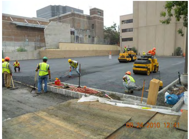
Site Restoration – Asphalt Placement Completing Asphalt Base Course Placement & Compaction August 24, 2010
