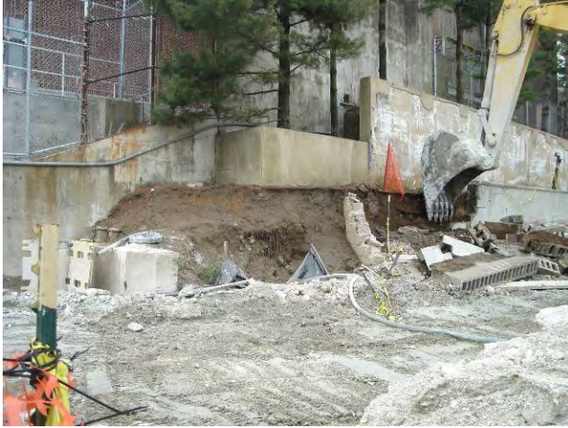
Site Restoration – Planter Wall Demolition Demolishing East Portion of Planter Wall April 6, 2010
