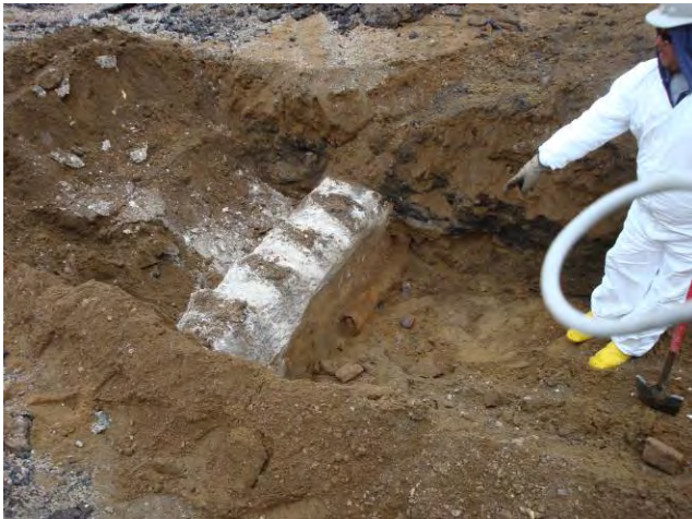
Demo of Structures for West Side Remnant Foundation to be Excavated March 26, 2009
