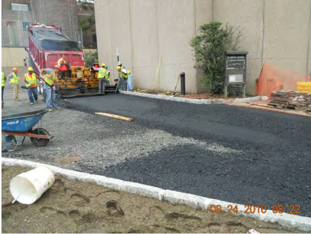
Site Restoration – Asphalt Placement Placing Asphalt Base Course along Western Perimeter August 24, 2010
