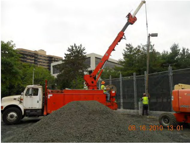
Site Restoration – Lighting Placing Light Pole on Light Pole Base August 16, 2010
