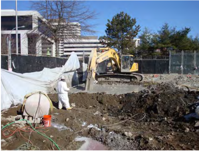
Excavator ISS – Cell Mixing Excavator Mixing Cell P-2 February 21, 2009
