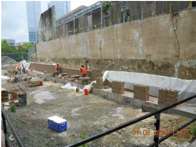
Site Restoration – Planter Wall Stucco Reconstruction Masonry Block July 8, 2010
