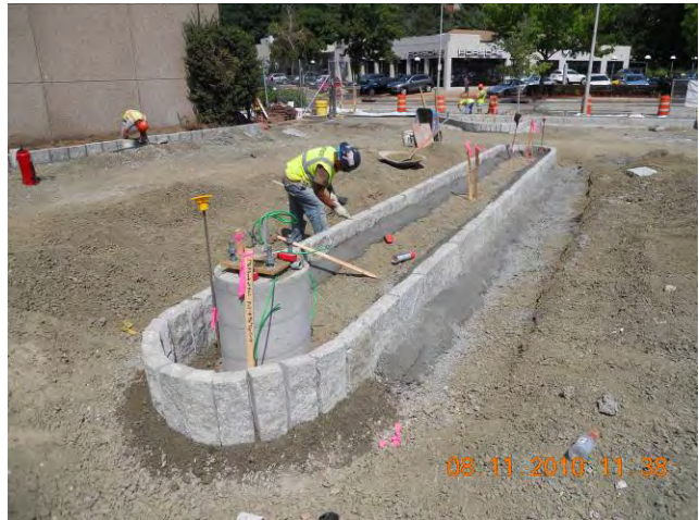
Site Restoration – Curbing Finishing Curb Blocks for Central Planter Area August 11, 2010
