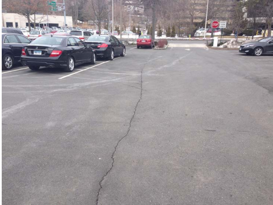
Photo 3: East Side of Water Street Parking Lot (facing North)
