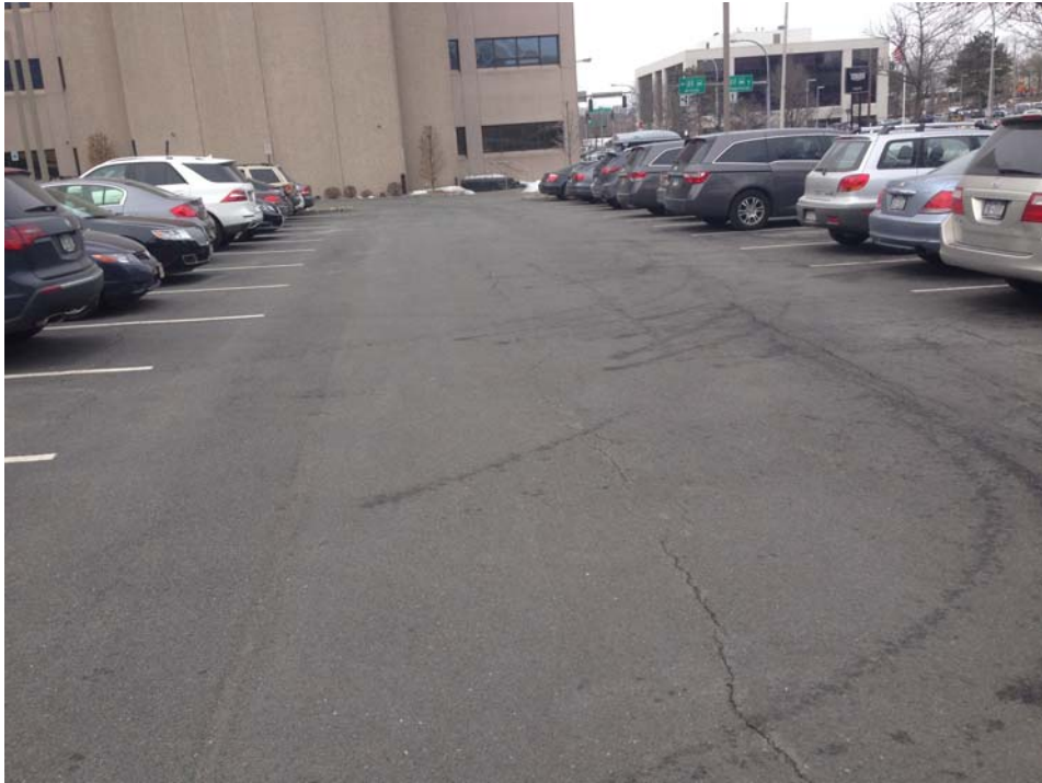
Photo 6: Smith Street Parking Lot (facing West)
