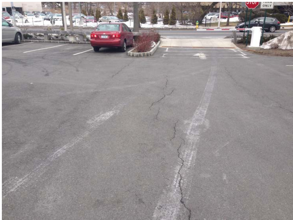
Photo 4: Water Street Parking Lot (facing North)
