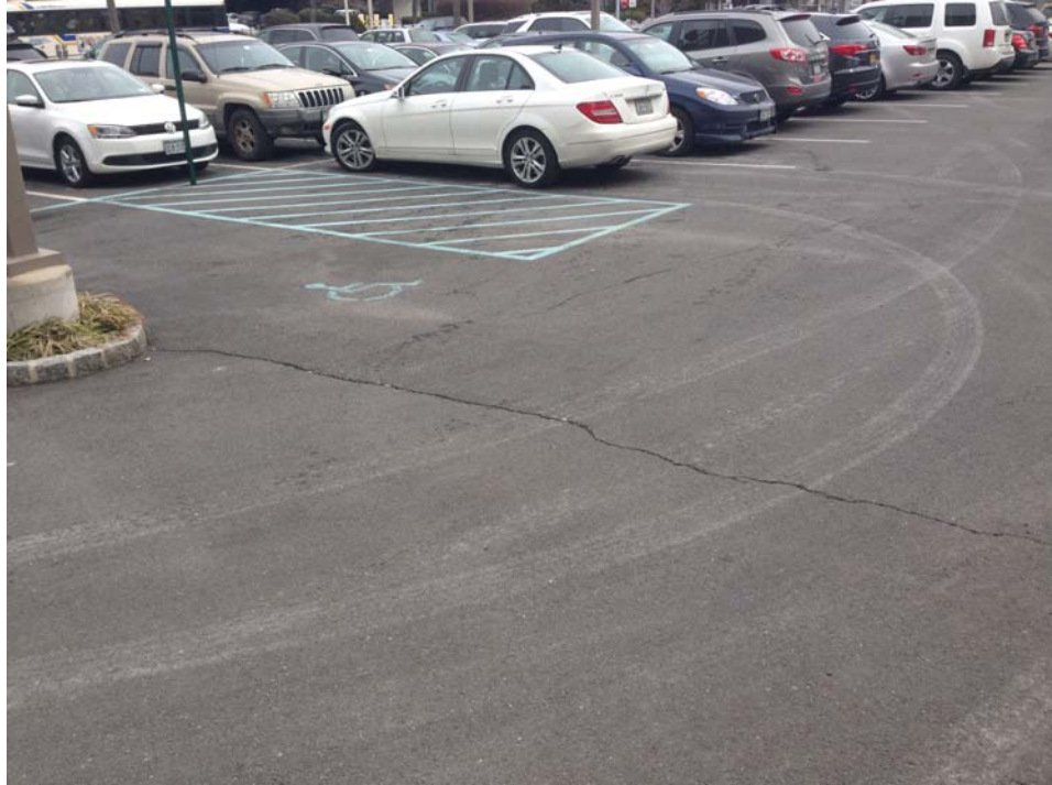
Photo 1: Water Street Parking Lot (facing Northeast)
