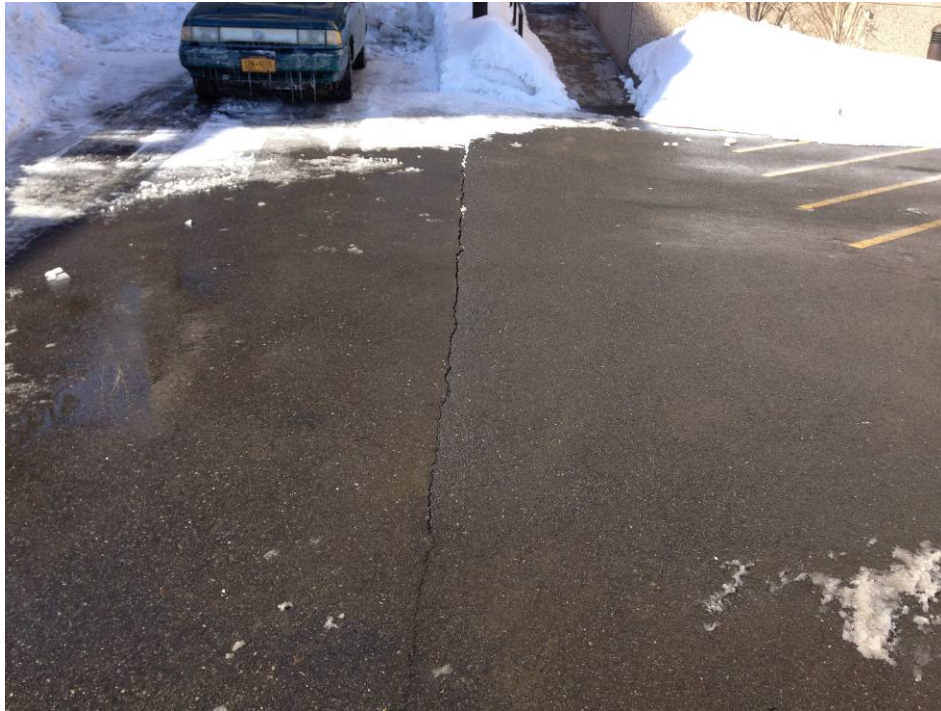
Photo 7: West Side of Water Street Parking Lot (facing West)
