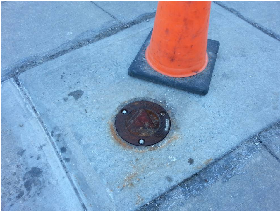
Photo 9: MW-18 Well Cover Replaced on 3/12/15
