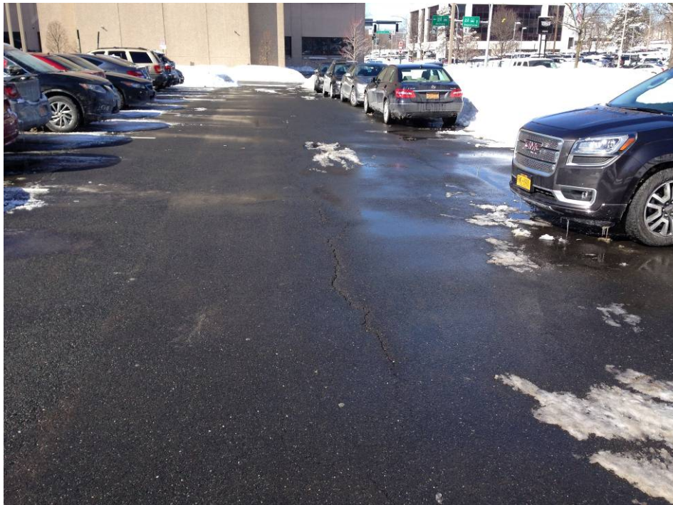
Photo 4: Water Street Parking Lot (facing West)
