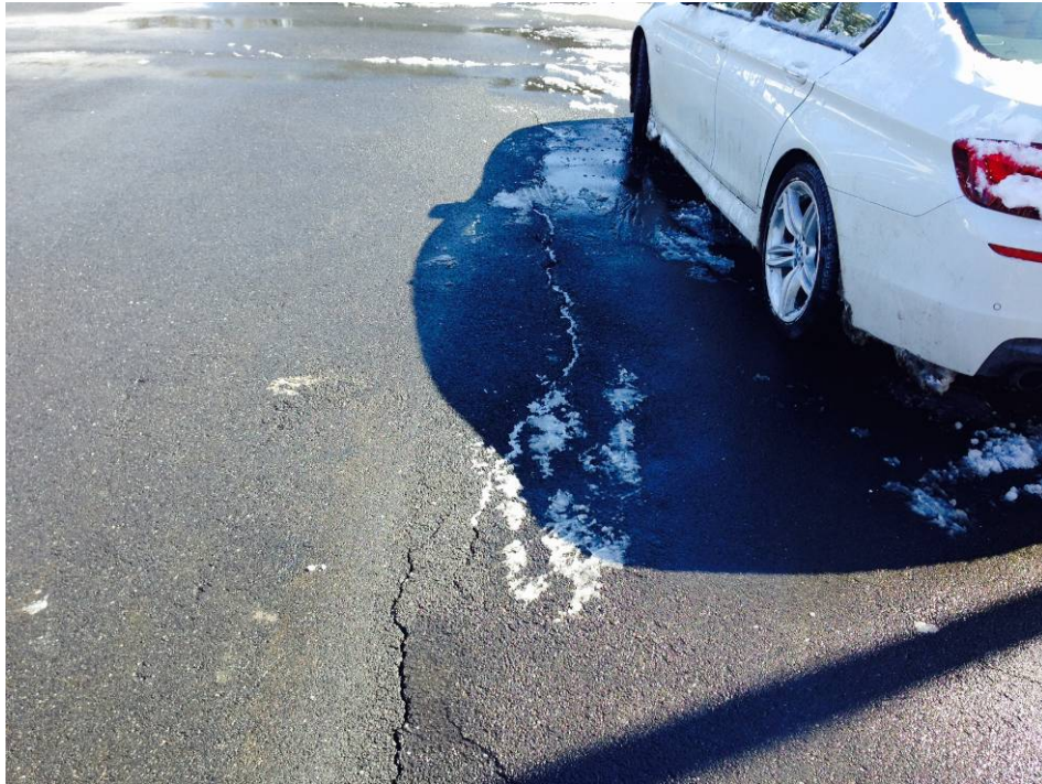
Photo 5: Water Street Parking Lot (facing North)
