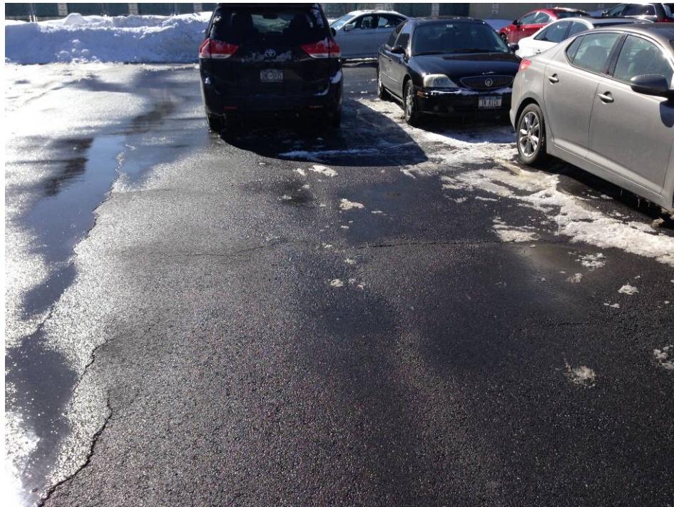
Photo 6: Water Street Parking Lot (facing South)
