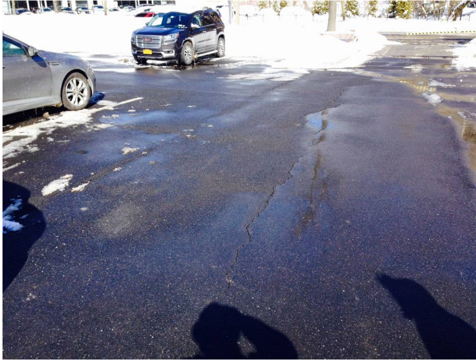
Photo 1: East Side of Water Street Parking Lot (facing North)
