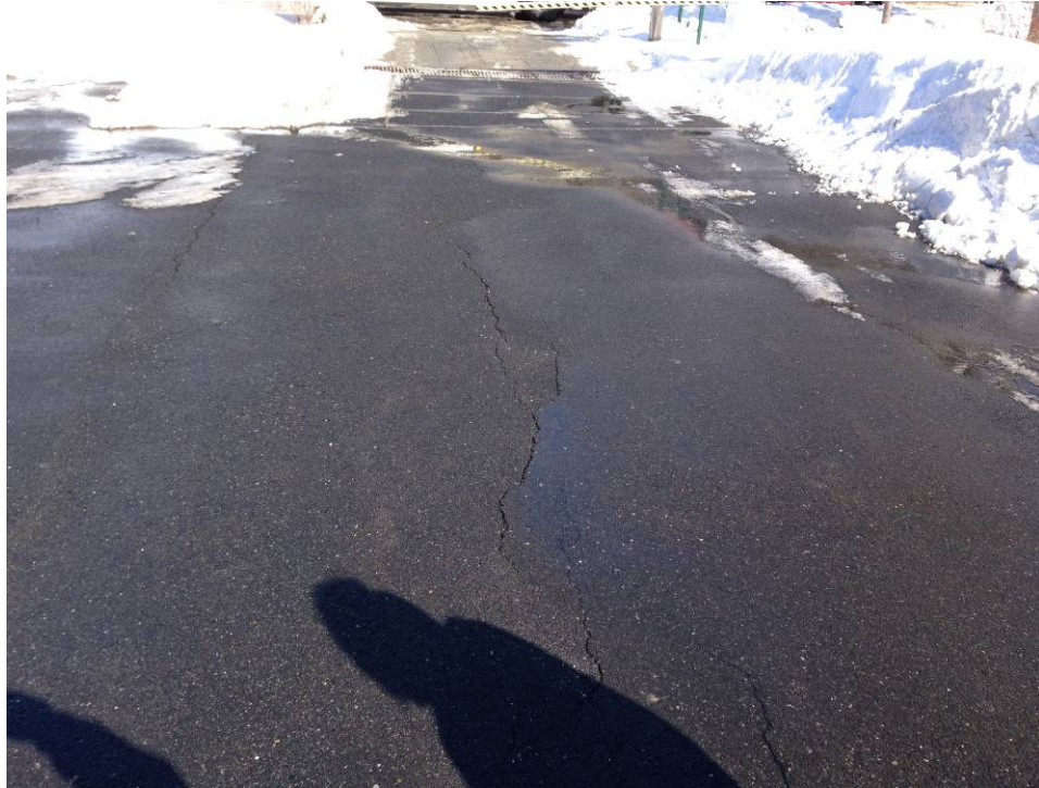
Photo 3: Water Street Parking Lot (facing North)
