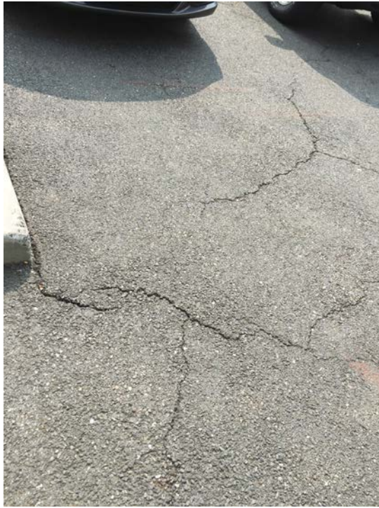
Photo 3: Substation Parking Lot (facing East)
