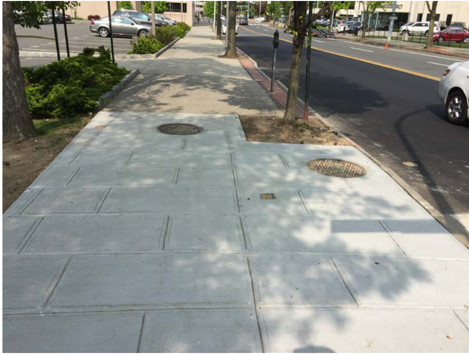
Photo 17: Newly Poured Sidewalk Along Water Street Parking (facing West)
