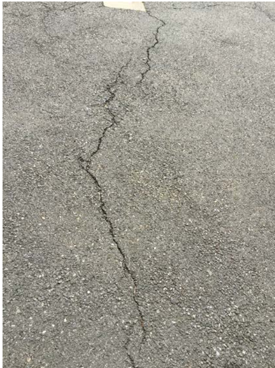
Photo 2: Substation Parking Lot (facing South)
