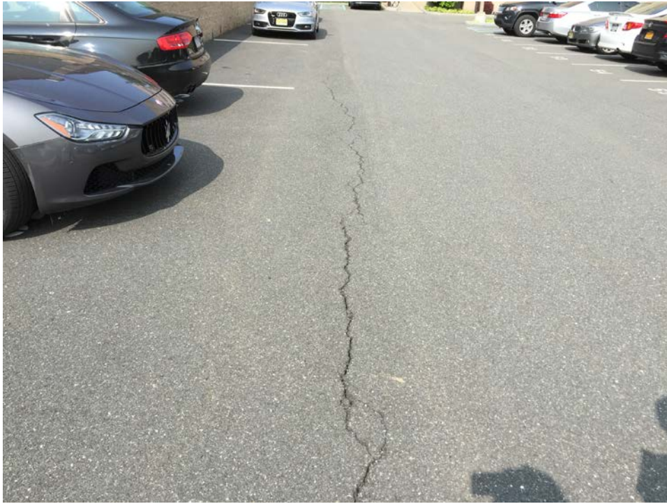
Photo 11: Water Street Parking Lot (facing West)
