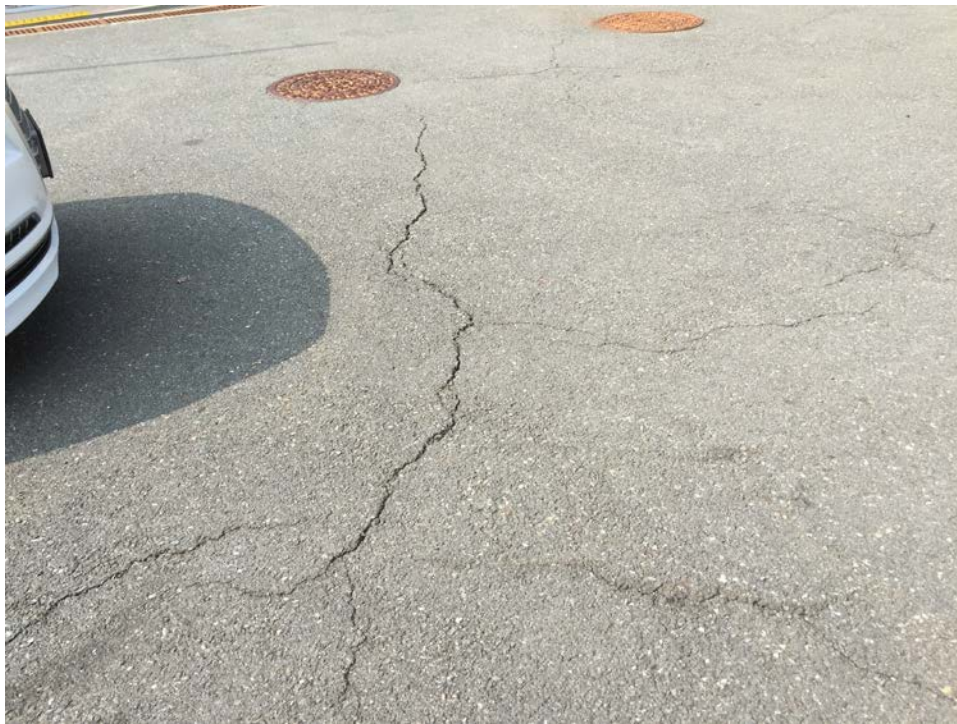
Photo 4: Substation Parking Lot (facing South)
