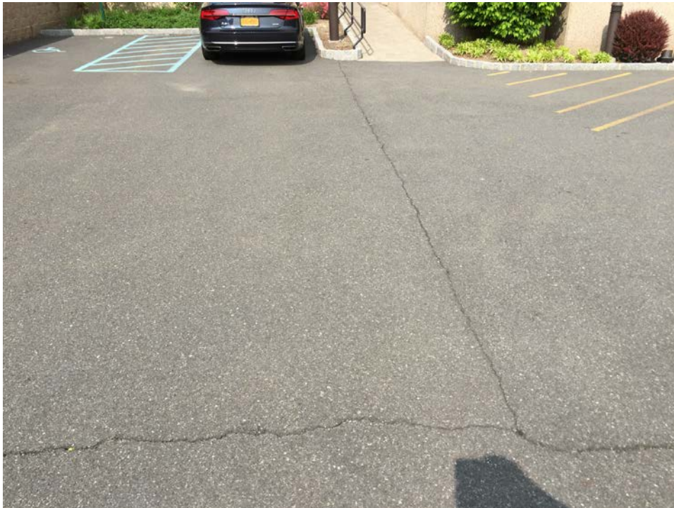
Photo 12: Water Street Parking Lot (facing West)
