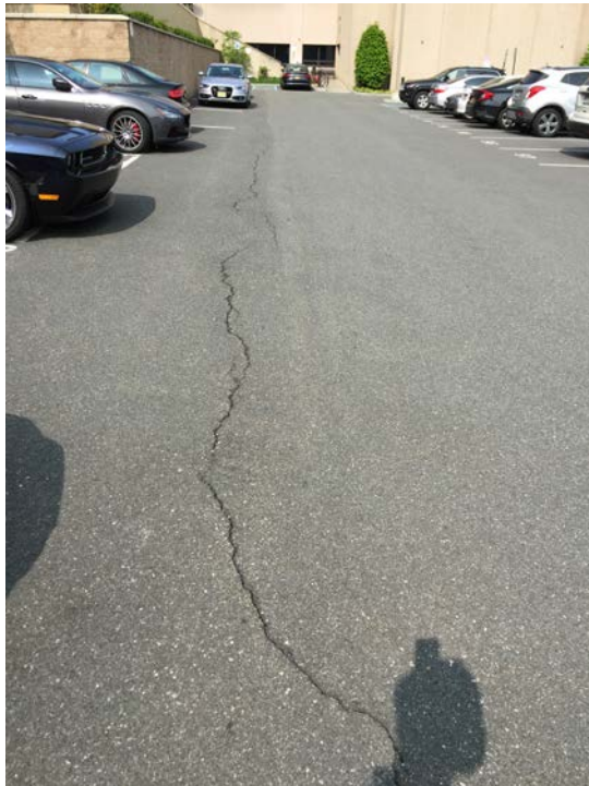
Photo 10: Water Street Parking Lot (facing West)
