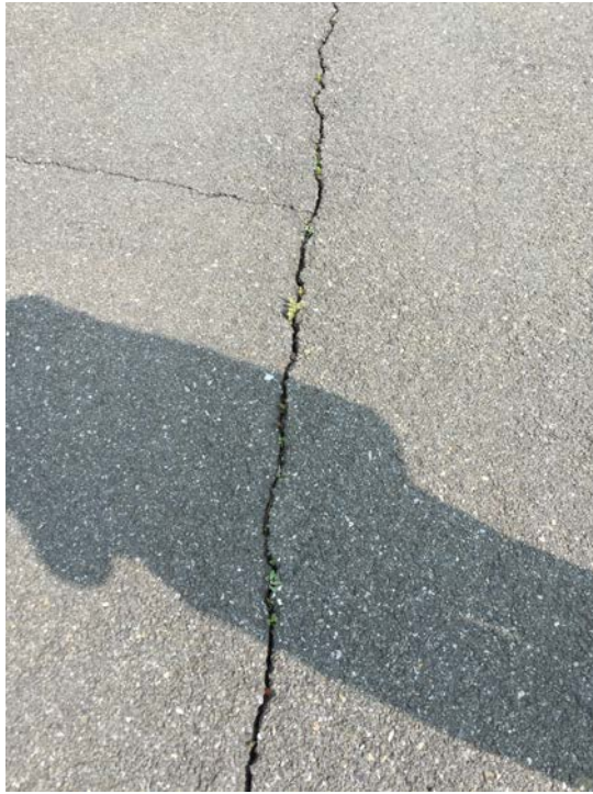
Photo 9: Water Street Parking Lot (facing North)
