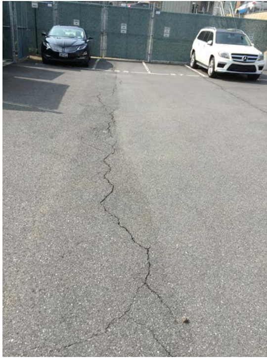
Photo 7: Water Street Parking Lot (facing South)
