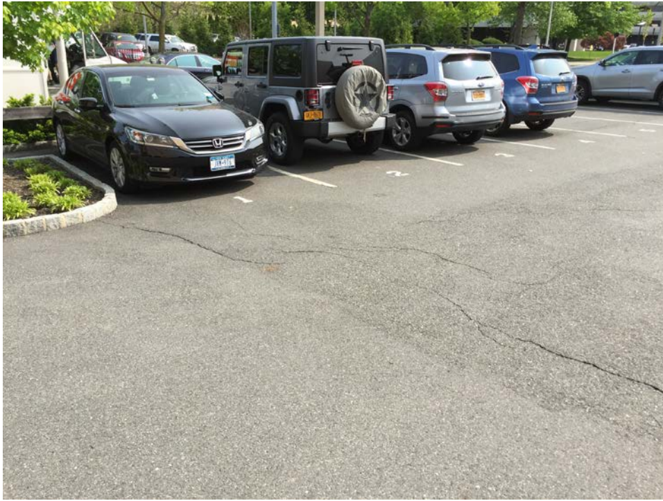
Photo 15: Water Street Parking Lot (facing Northeast)
