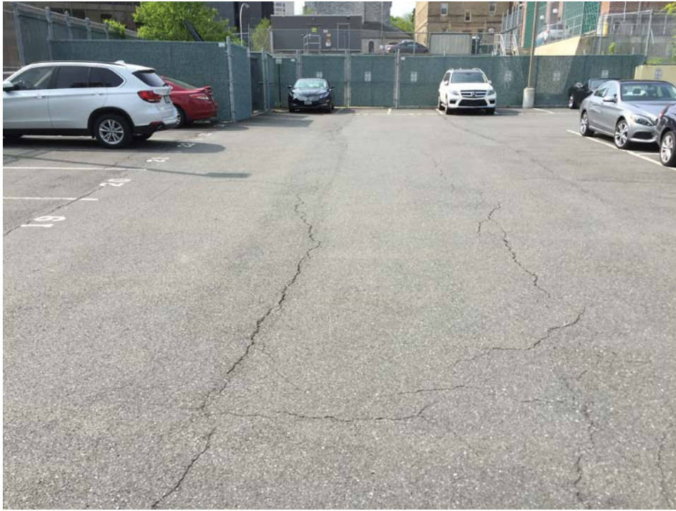
Photo 5: Water Street Parking Lot (facing South)
