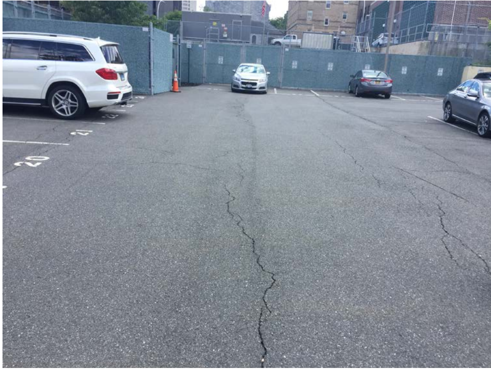
Photo 7: Water Street Parking Lot (facing South)
