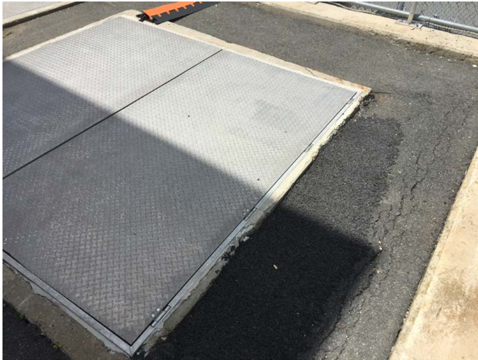
Photo 1: Substation Parking Lot filled in depression along equipment vault (facing North)
