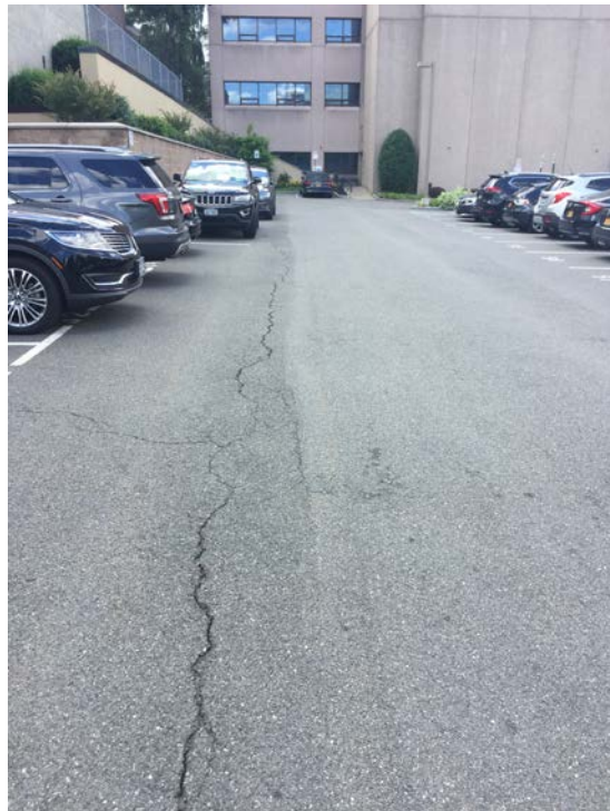
Photo 8: Water Street Parking Lot (facing West)
