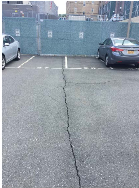
Photo 5: Water Street Parking Lot (facing South)
