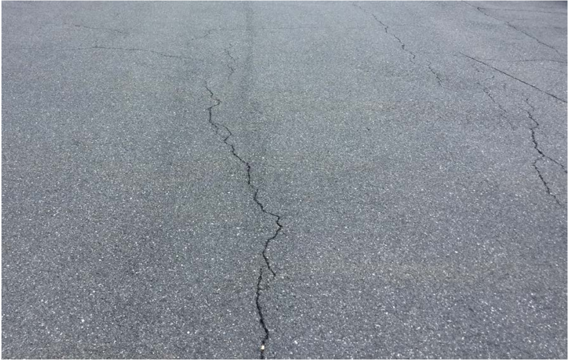
Photo 3: Substation Parking Lot (facing South)
