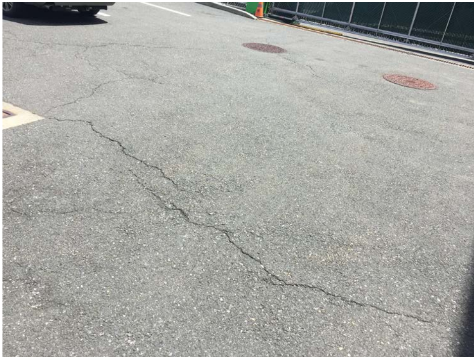
Photo 4: Substation Parking Lot (facing South)
