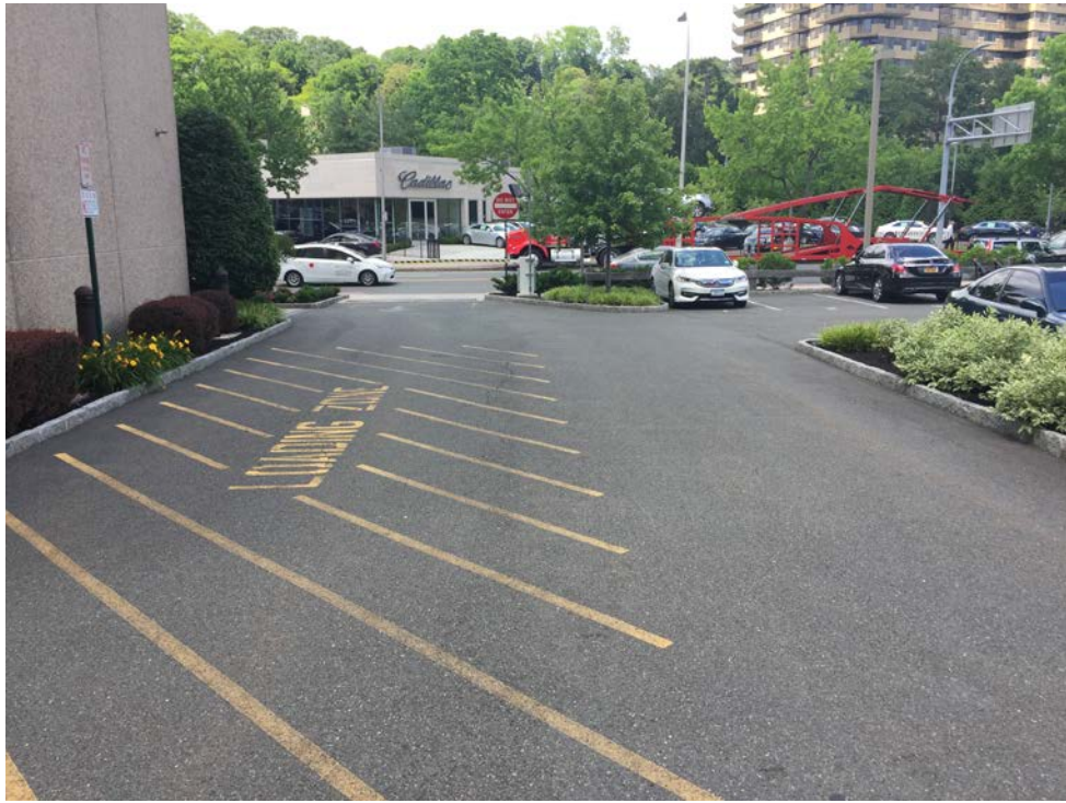
Photo 11: Water Street Parking Lot (facing North)
