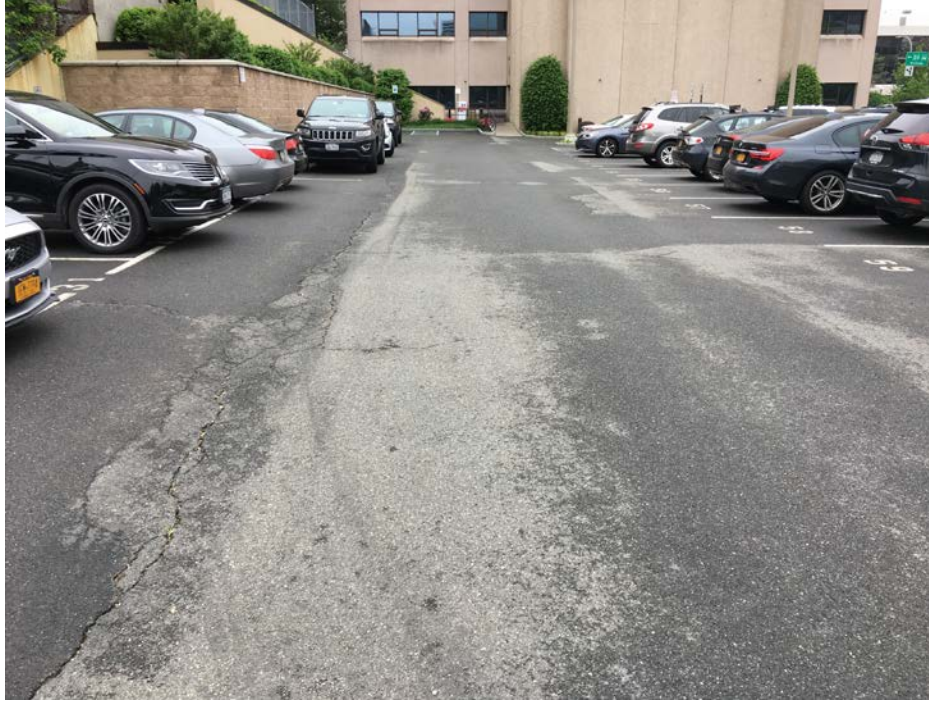
Photo 9: Water Street Parking Lot (facing West)
