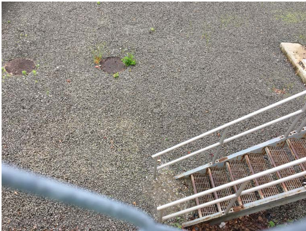
Photo 2: Sink hole no longer in gravel cover area near Transformer Vault No. 3 (facing East)
