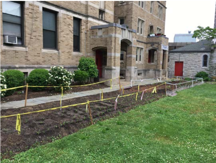
Photo 14: Newly installed flower/vegetable bed in St John’s Courtyard (facing Northeast)
