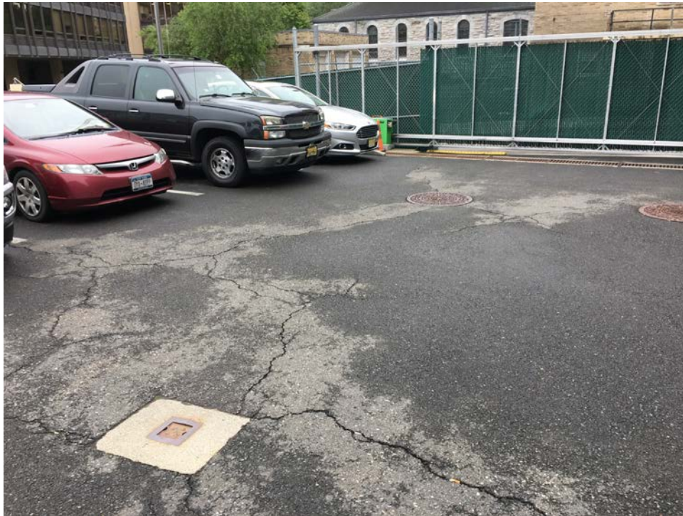
Photo 4: Substation Parking Lot (facing South)
