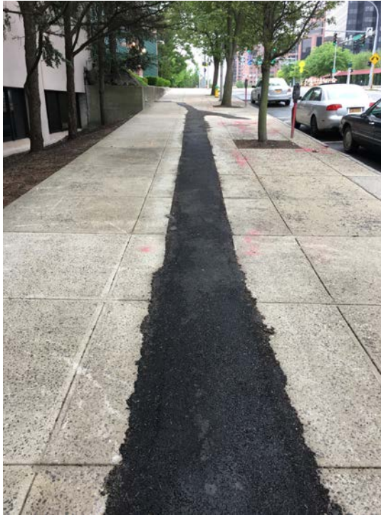
Photo 16: Telecommunications Repair Trenching along North Lexington Avenue (facing South)
