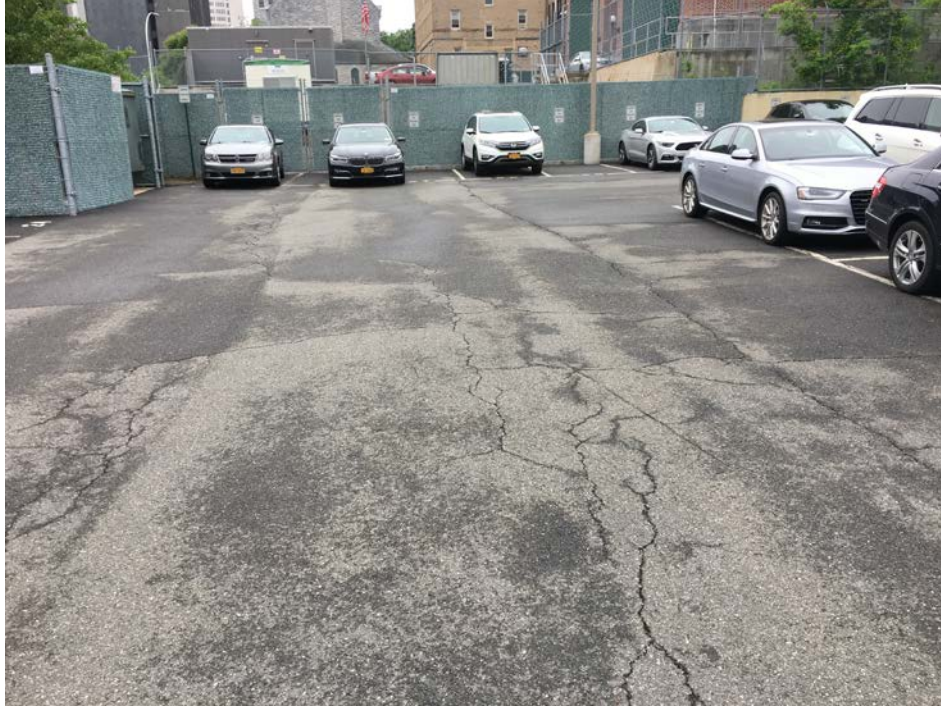
Photo 7: Water Street Parking Lot (facing South)
