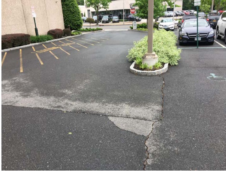
Photo 11: Water Street Parking Lot (facing North)
