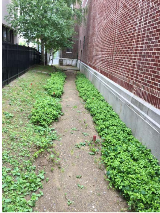
Photo 15: Location of Trenching for Telecommunications Repair Work (facing East)
