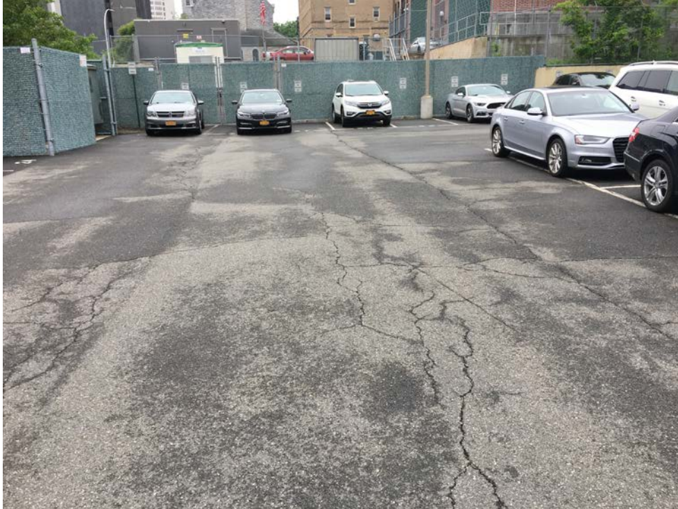
Photo 5: Water Street Parking Lot (facing South)
