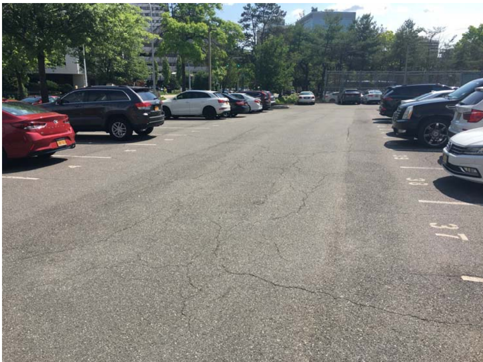
Photo 10: Water Street Parking Lot (facing East)
