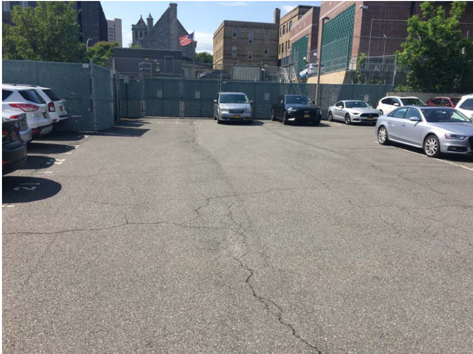
Photo 5: Water Street Parking Lot (facing South)
