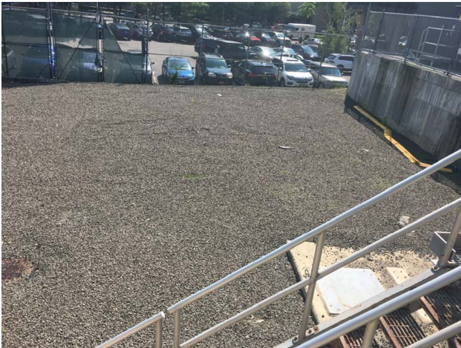
Photo 2: Gravel cover area near Transformer Vault No. 3 (facing East)
