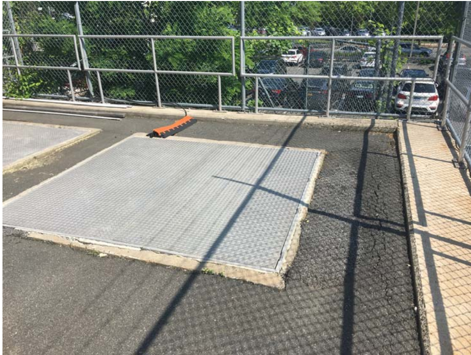
Photo 1: Alley between Transformer Vaults No. 3 and 4 (facing North)
