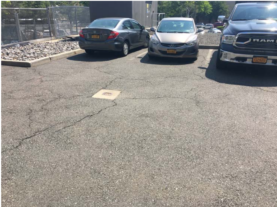
Photo 4: Substation Parking Lot (facing Northeast)
