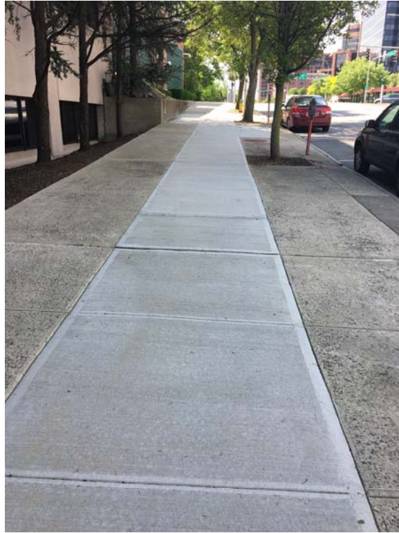
Photo 15: Trenching Sidewalk Repair along North Lexington Avenue (facing South)
