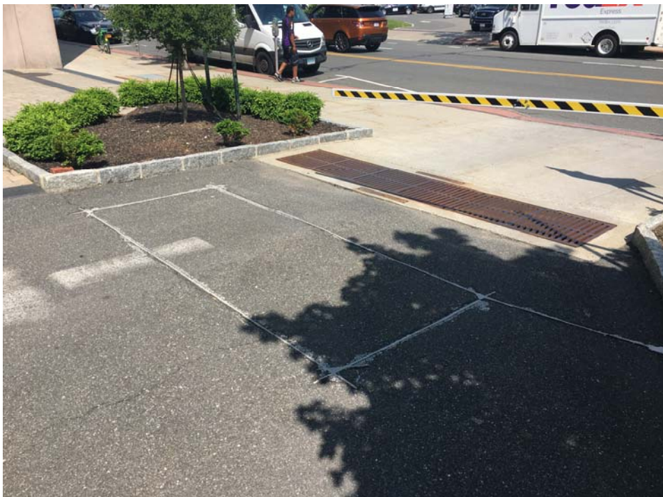
Photo 12: Water Street Parking Lot (facing Northwest)
