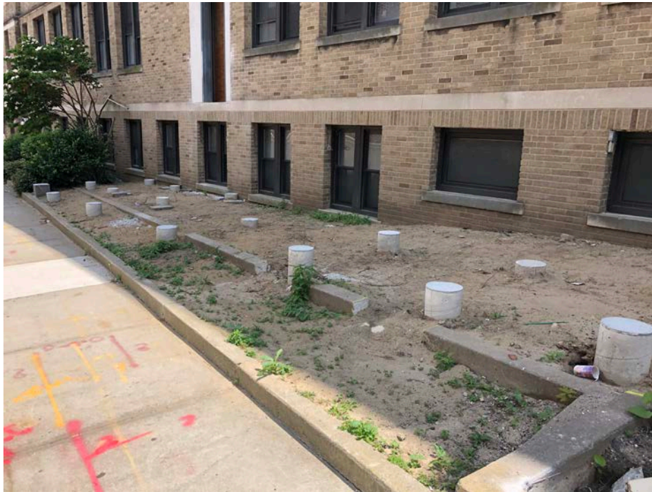
Photo 16: Construction of Handicapped Access Ramp at St. John's
