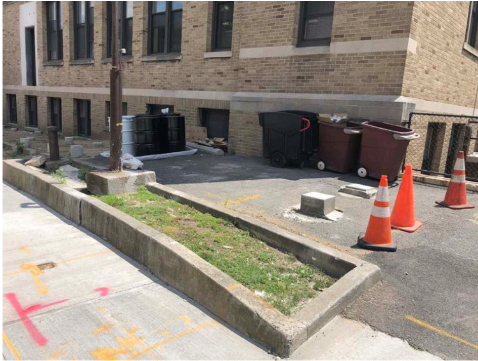
Photo 15: Construction of Handicapped Access Ramp at St. John's
