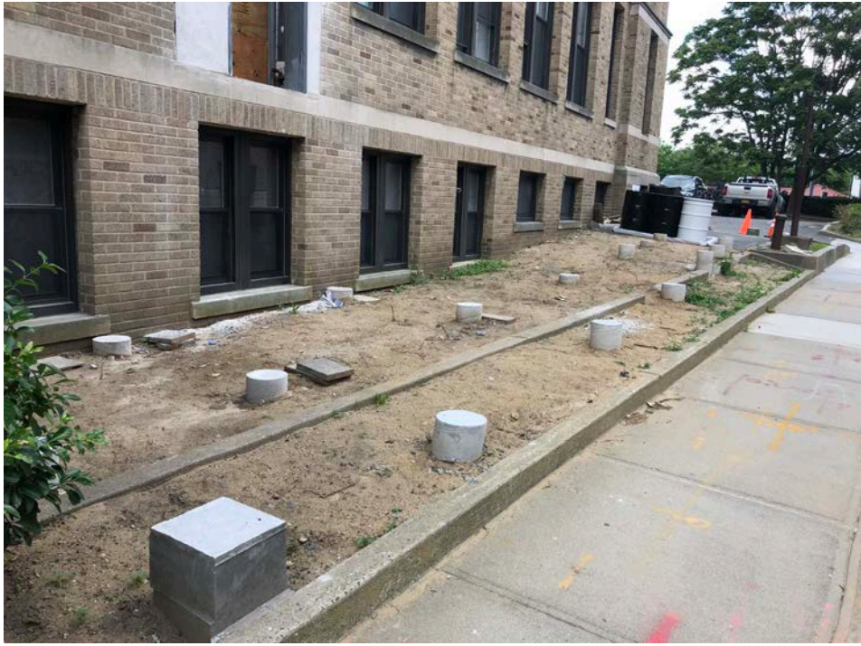
Photo 17: Construction of Handicapped Access Ramp at St. John's
