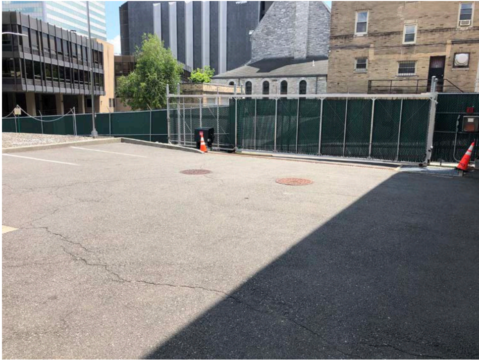
Photo 3: Substation Parking Lot (facing South)
