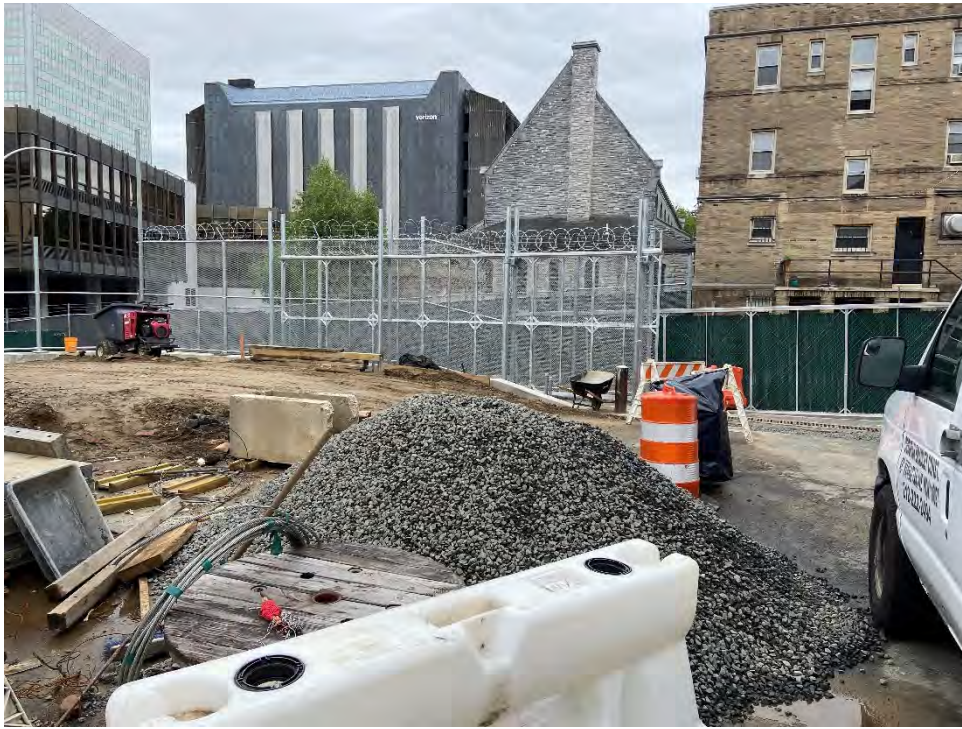
Photo 3: Substation Parking Lot (facing Southeast)
