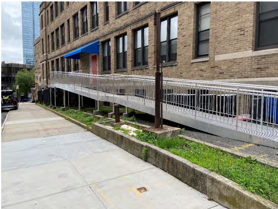
Photo 16: Newly Constructed Handicapped Access Ramp at St. John's
