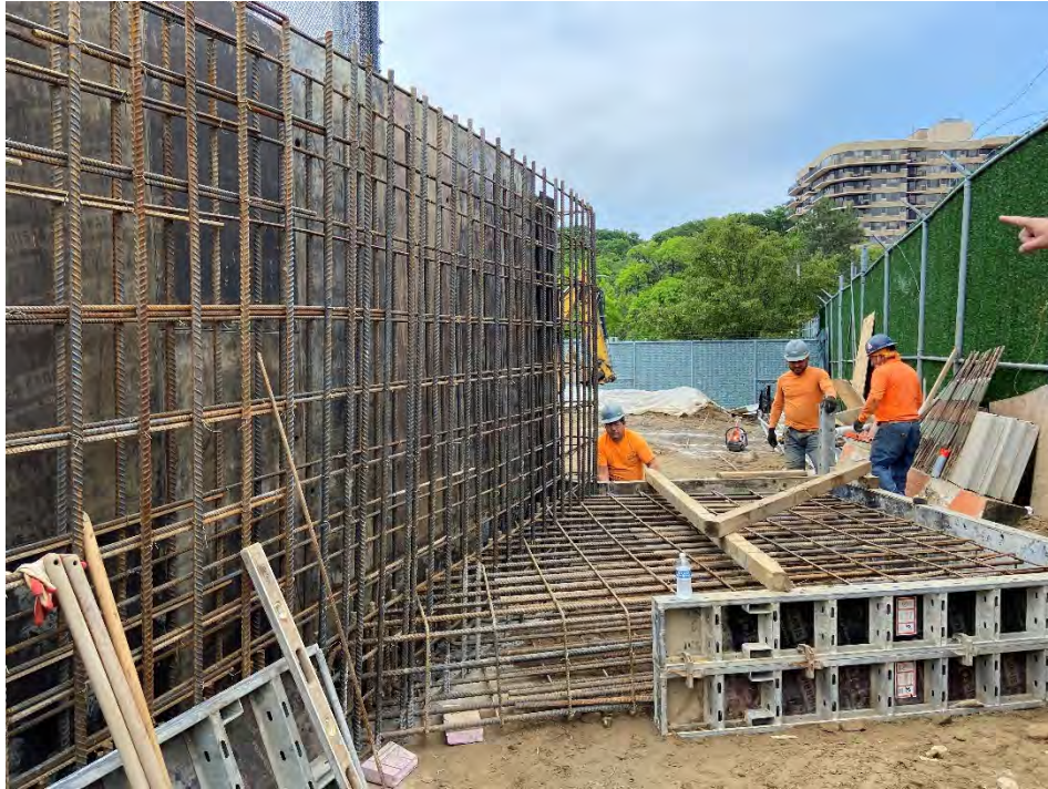
Photo 9: Concrete Wall Reinforcement (looking North)
