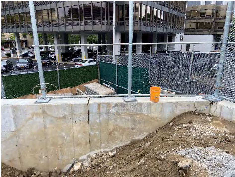
Photo 7: Newly Constructed Retaining Wall (looking Southeast)
