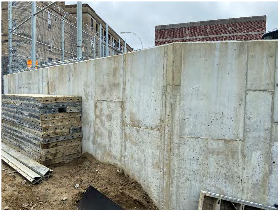
Photo 10: Front of Newly Constructed Retaining Wall (looking Southwest)
