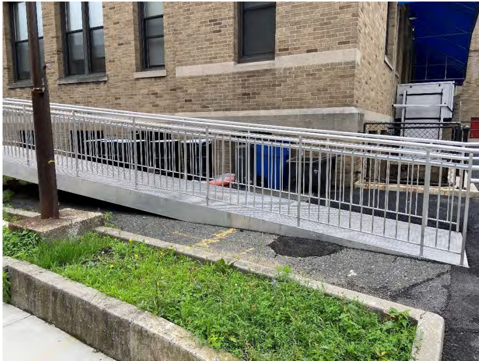
Photo 15: Newly Constructed Handicapped Access Ramp at St. John's
