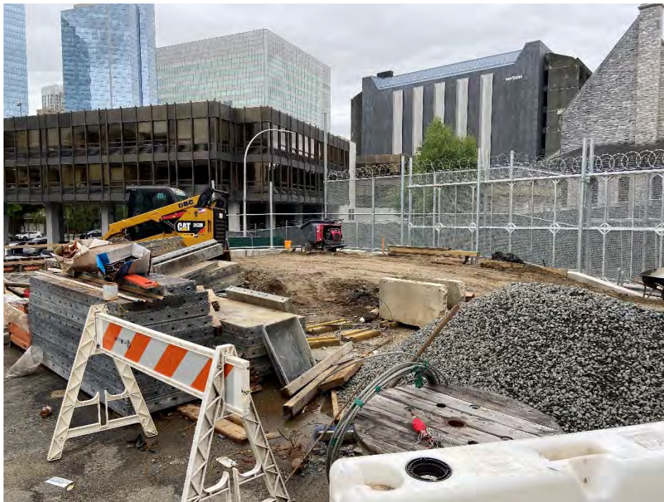
Photo 4: Substation Parking Lot (facing Southeast)
