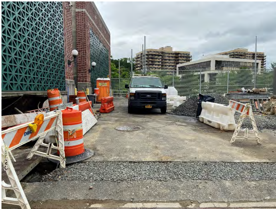
Photo 6: Substation Parking Area (Looking North)
