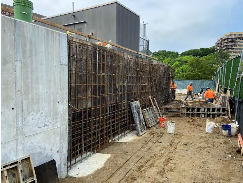
Photo 11: Front of Newly Constructed Retaining Wall (looking North)
