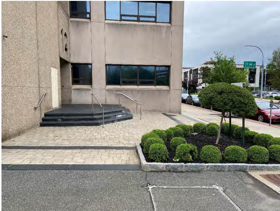
Photo 11: Water Street Parking Lot (facing Northwest)
