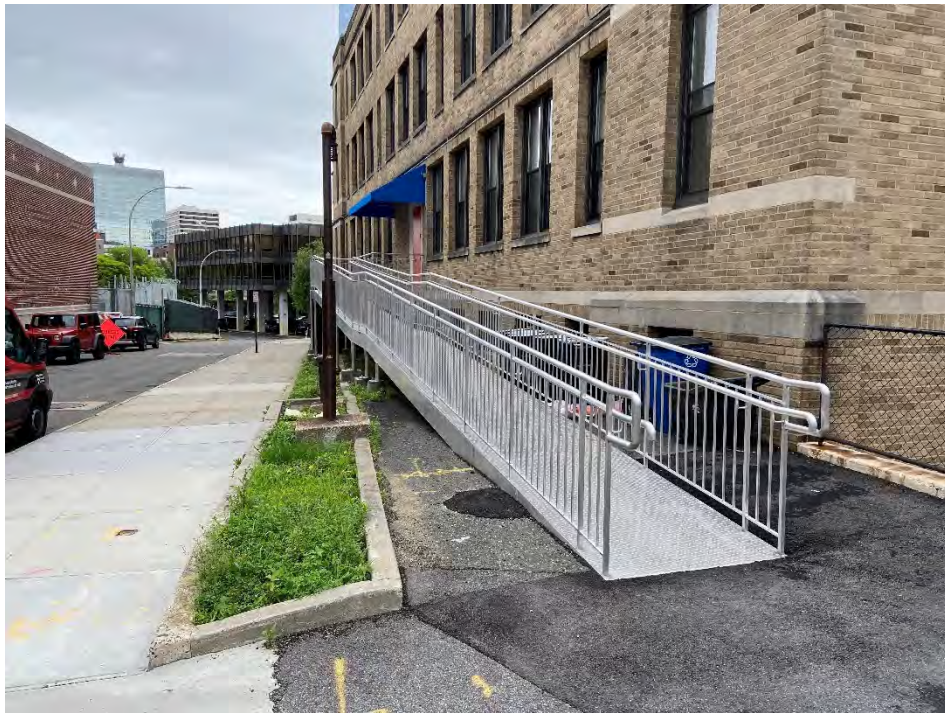
Photo 14: Newly Constructed Handicapped Access Ramp at St. John's
