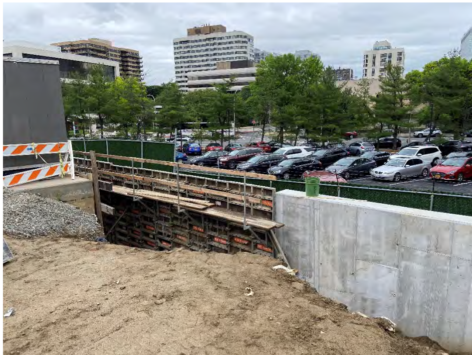
Photo 8: Concrete Forms for Retaining Wall (Looking Northeast)
