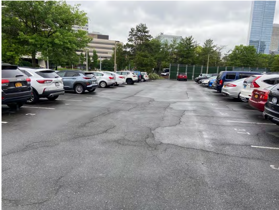
Photo 9: Water Street Parking Lot (facing East)
