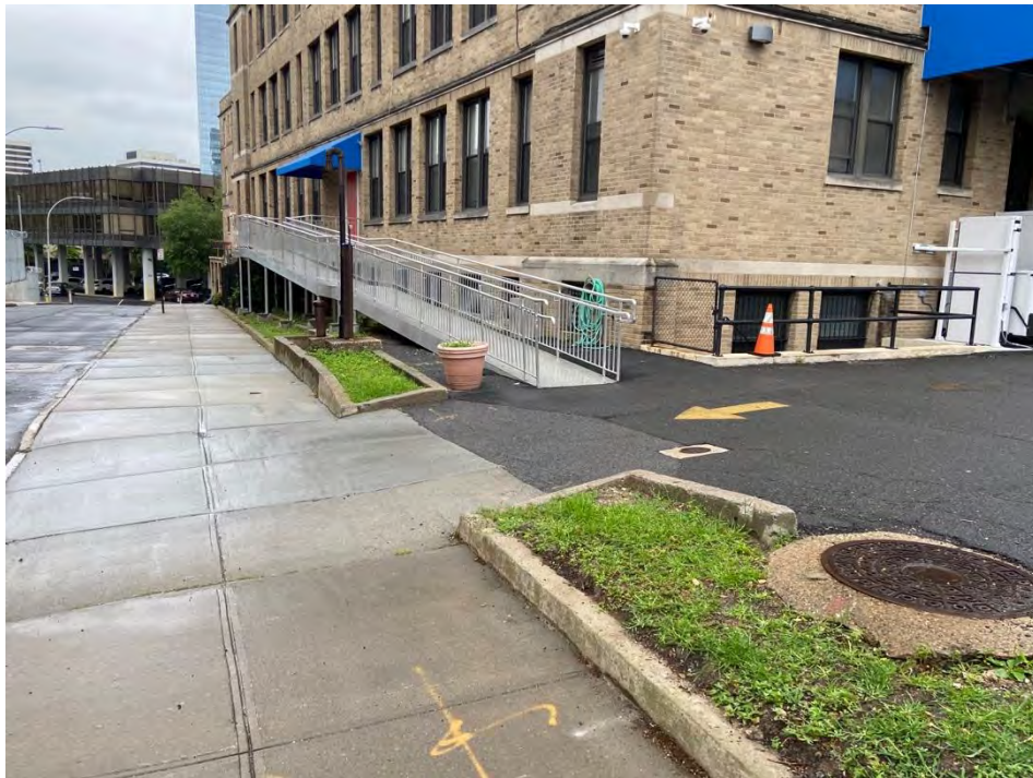
Photo 14: Handicapped Access Ramp adjacent to St John's School Building
