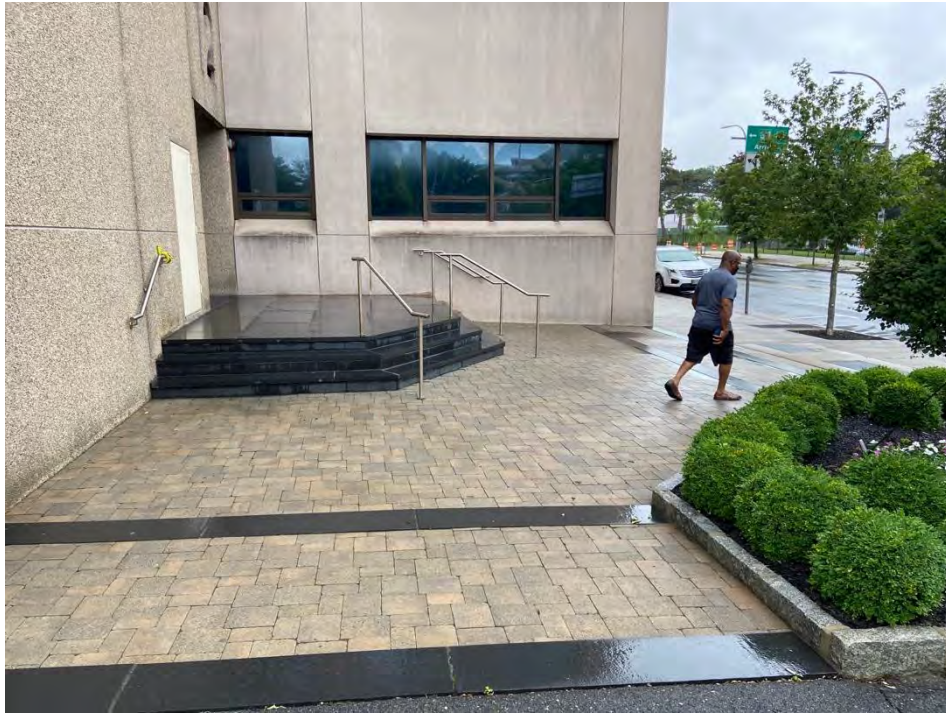
Photo 11: Water Street entrance (facing Northwest)
