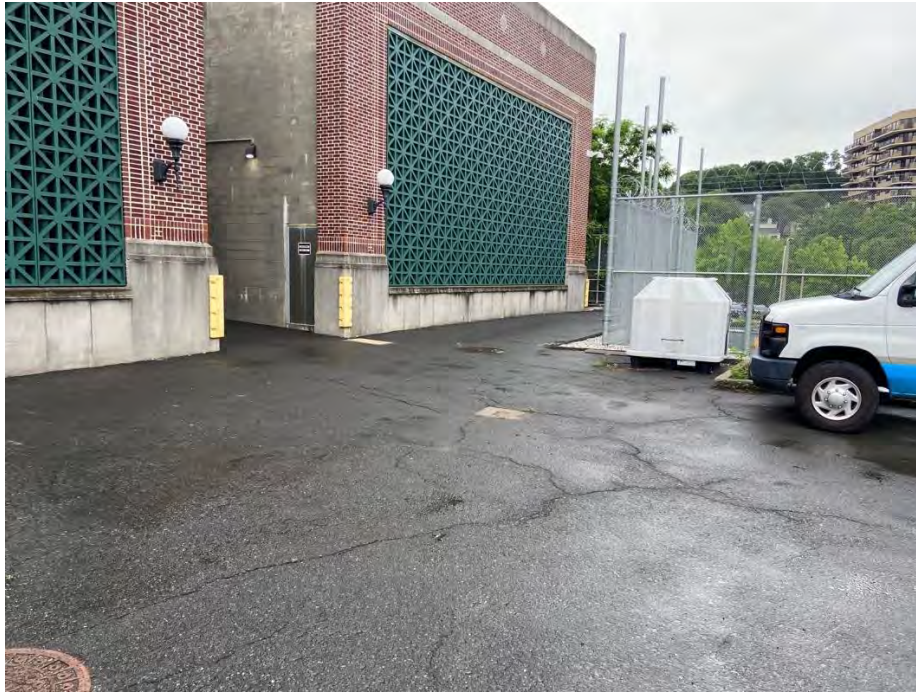
Photo 1: Alley between Transformer Vaults No. 3 and 4 (facing Northwest)
