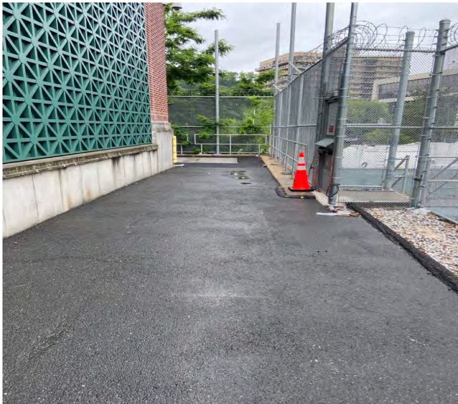
Photo 2: Driveway east of Transformer Vaults No. 3 and 4 (facing North)
