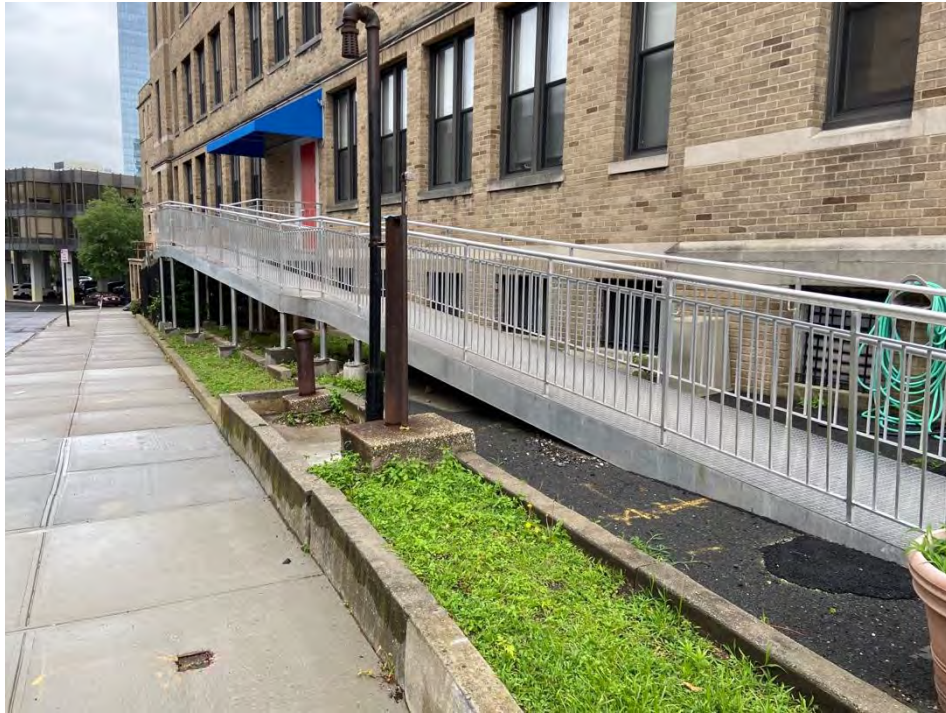
Photo 15: Handicapped Access Ramp adjacent to St John's School Building
