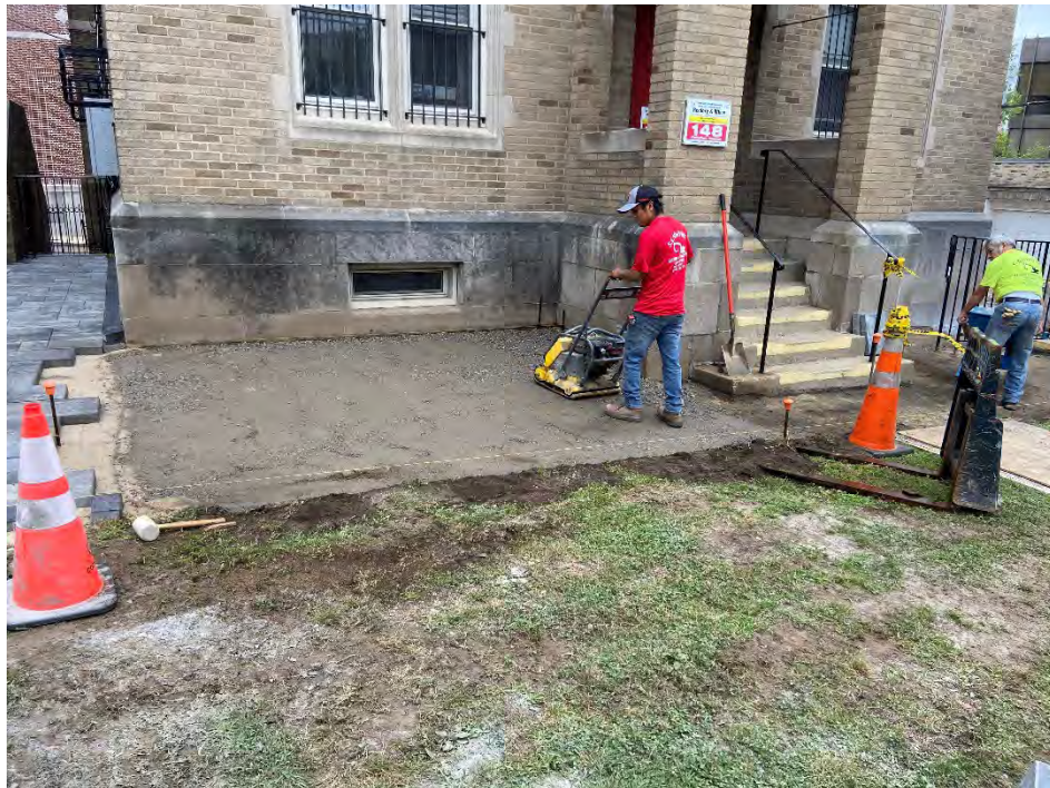
Photo 18: Surficial paver work conducted in the St John's Courtyard (facing Northeast)
