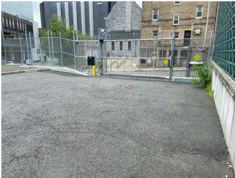
Photo 2: Parking area east of Transformer Vaults No. 3 and 4 (facing South)
