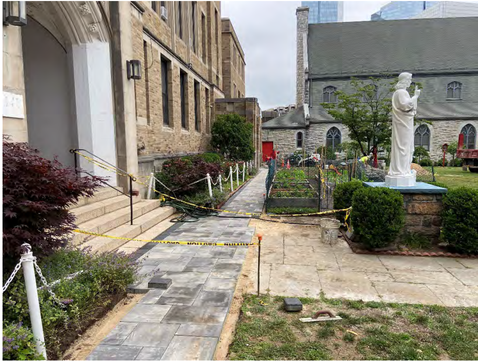
Photo 17: Surficial paver work conducted in the St John's Courtyard (facing East)
