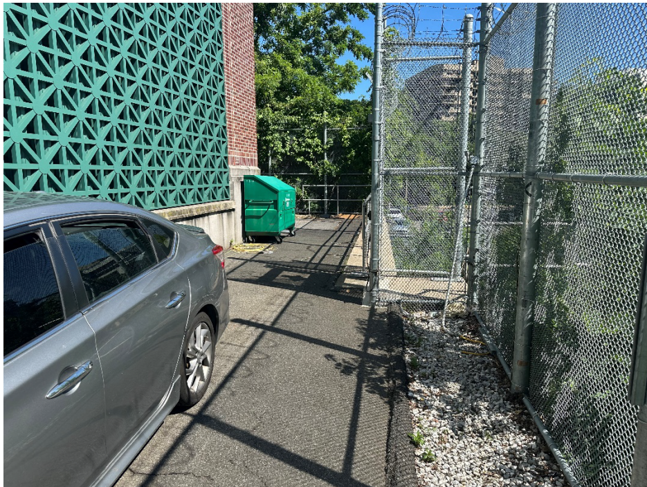
Photo 4: Driveway east of Transformer Vaults No. 3 and 4 (facing North)
