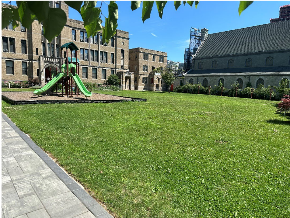
Photo 19: Surficial paver work completed in the St John's Courtyard (facing North)
