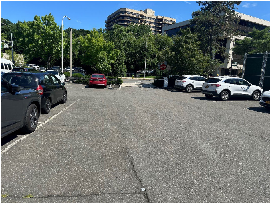
Photo 13: Water Street Parking Lot (facing North)
