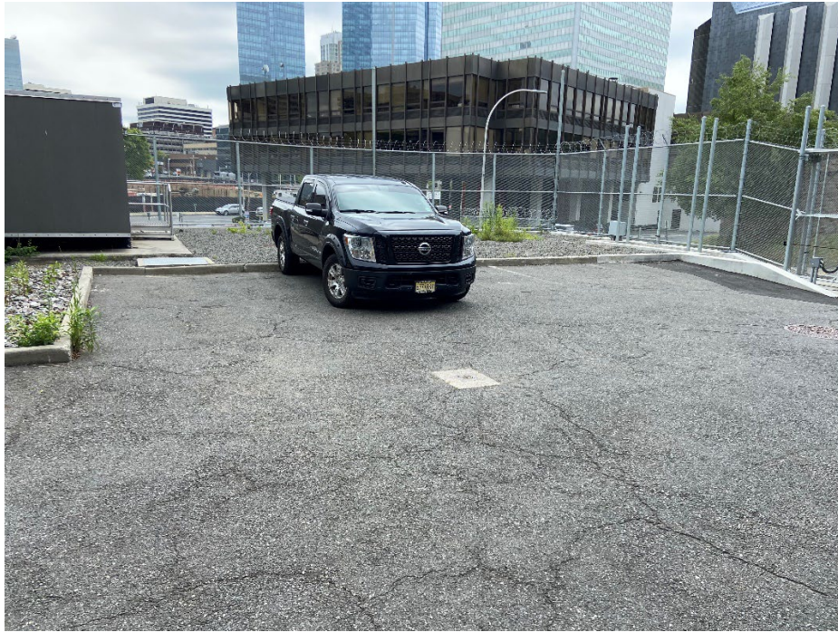
Photo 3: Parking area east of Transformer Vaults No. 3 and 4 (facing East)
