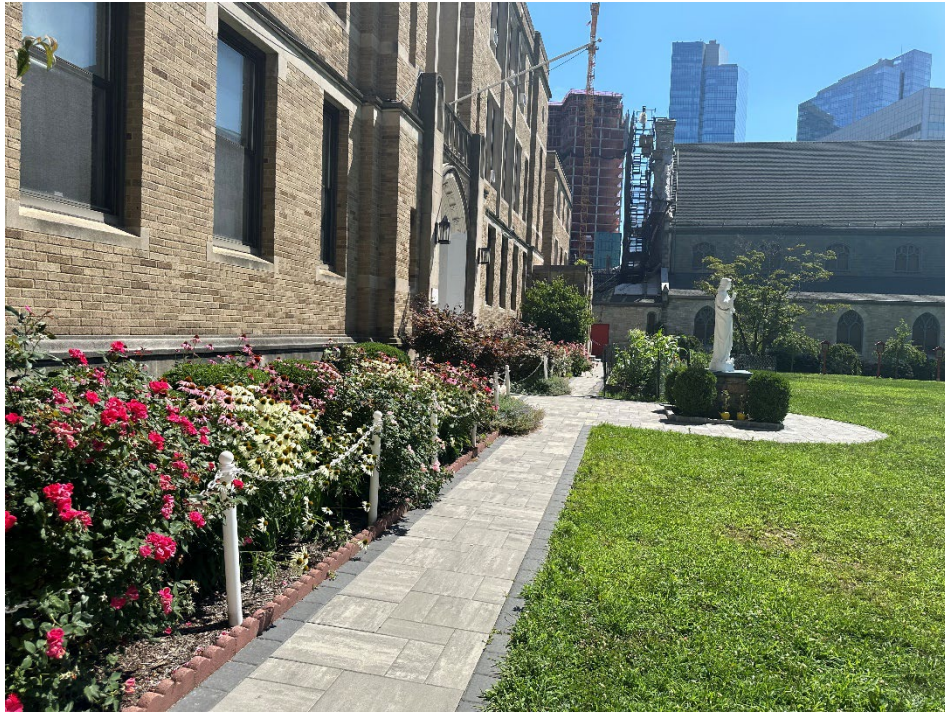
Photo 17: Surficial paver work completed in the St John's Courtyard (facing East)
