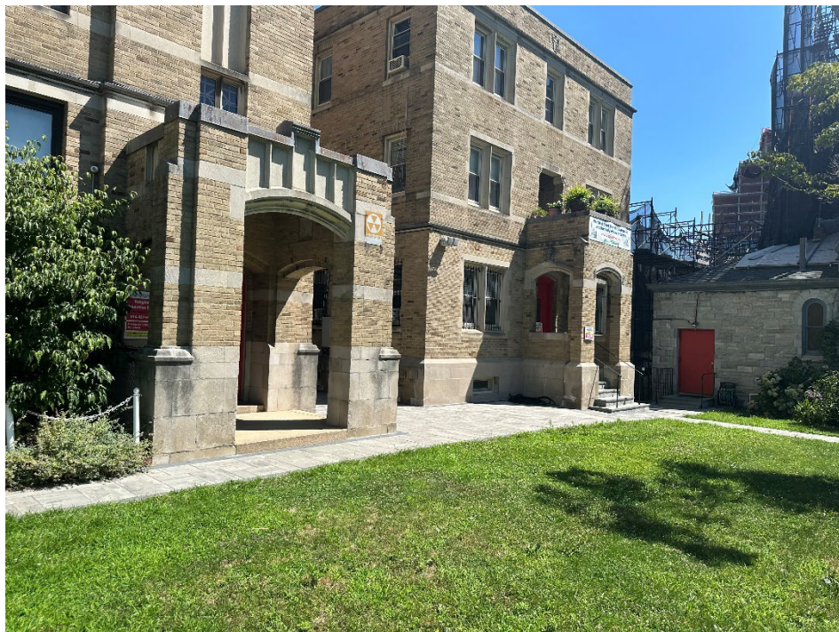
Photo 18: Surficial paver work completed in the St John's Courtyard (facing Northeast)
