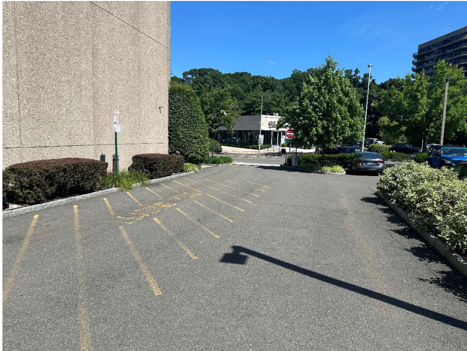
Photo 15: Water Street Parking Lot entrance (facing North)
