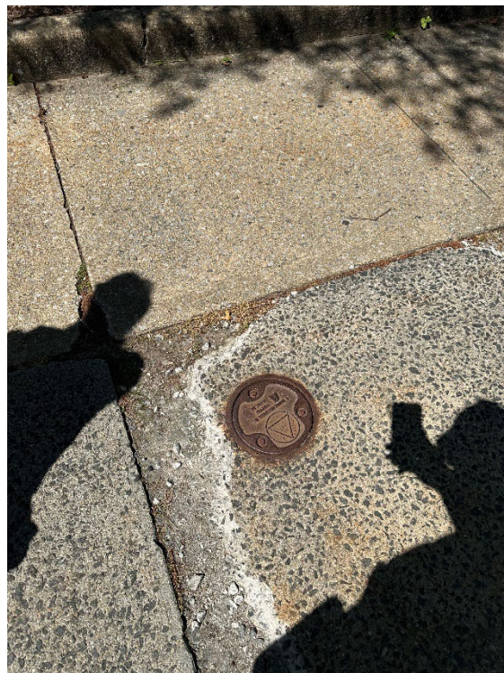
Photo 8: Monitoring Well (MW-7) on western sidewalk of of Dr. Martin Luther King Jr. Blvd
