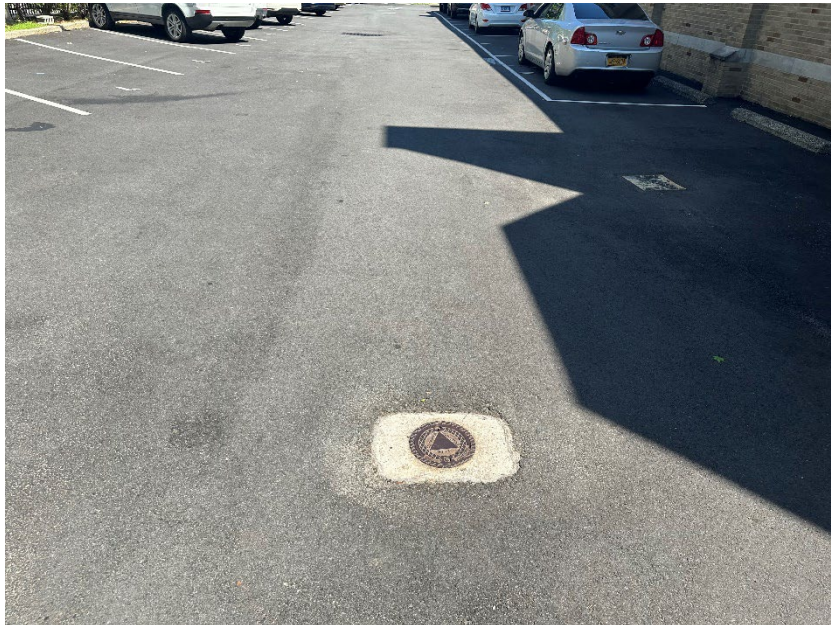
Photo 20: Western St. Johns driveway/parking lot (facing North)
