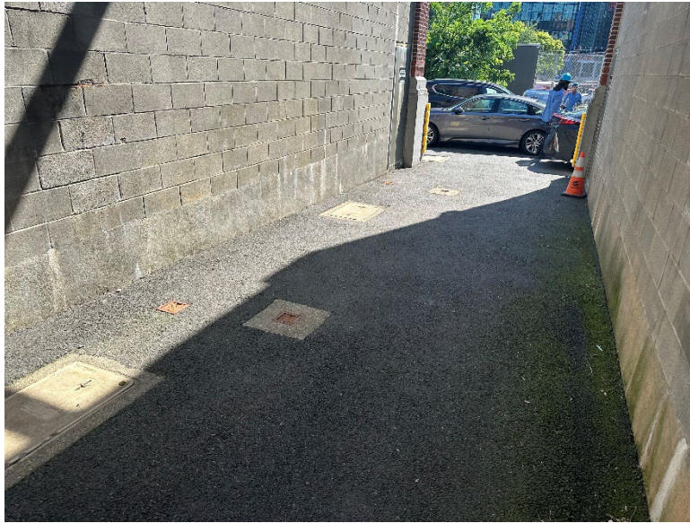
Photo 1: Alley between Transformer Vaults No. 3 and 4 (facing East)
