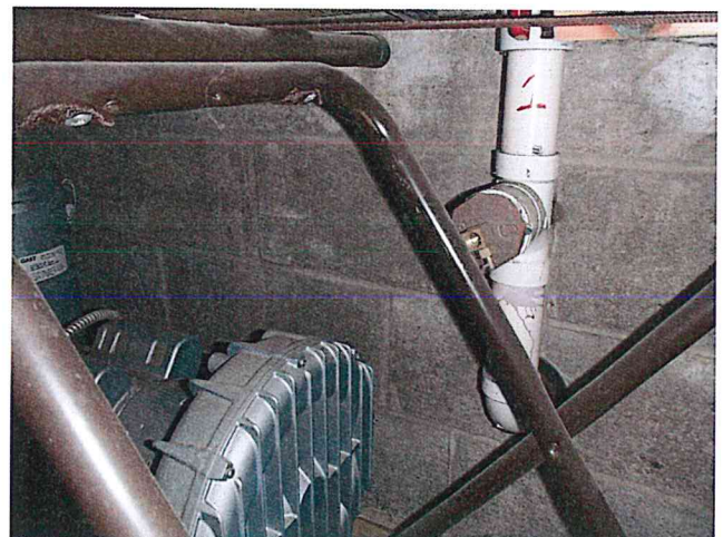
Photo 6: View of the suction point for VES-2.
