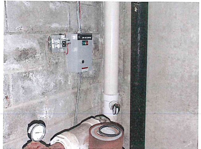
Photo 2: View of the PVC pipe that vents exhaust from VES-1 to the roof.
