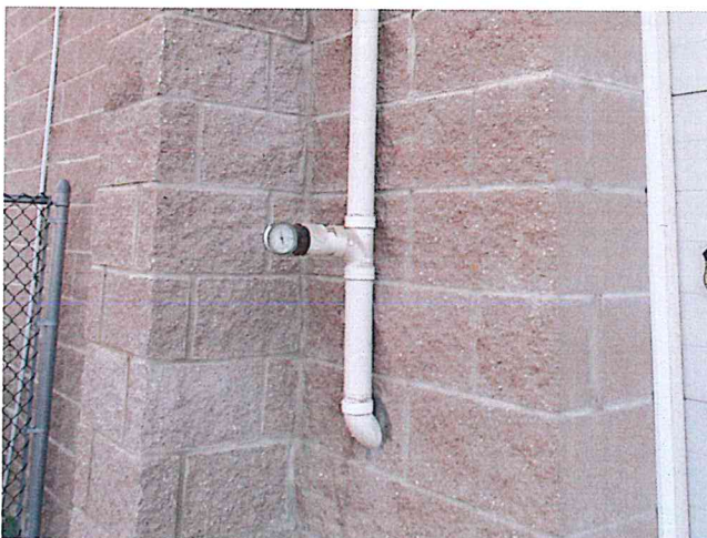
Photo 5: View of the PVC pipe that vents exhaust from VES-2 to the roof.
