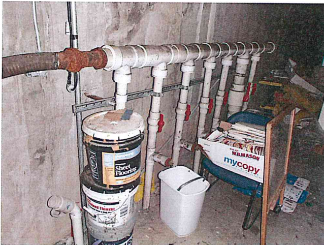
Photo 3: View of the suction points for VES-1.
