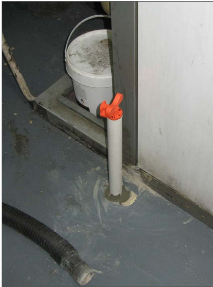
Photo 1. Vapor Extraction Point installed in Concrete Slab with sealing orange J-cap.
