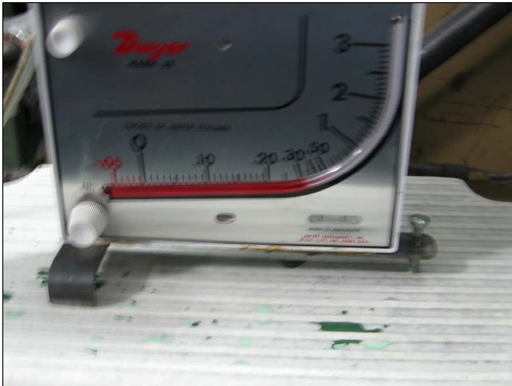
Photo 9. Vacuum gauge measuring -0.31 inches water at XP1 during pilot test.
