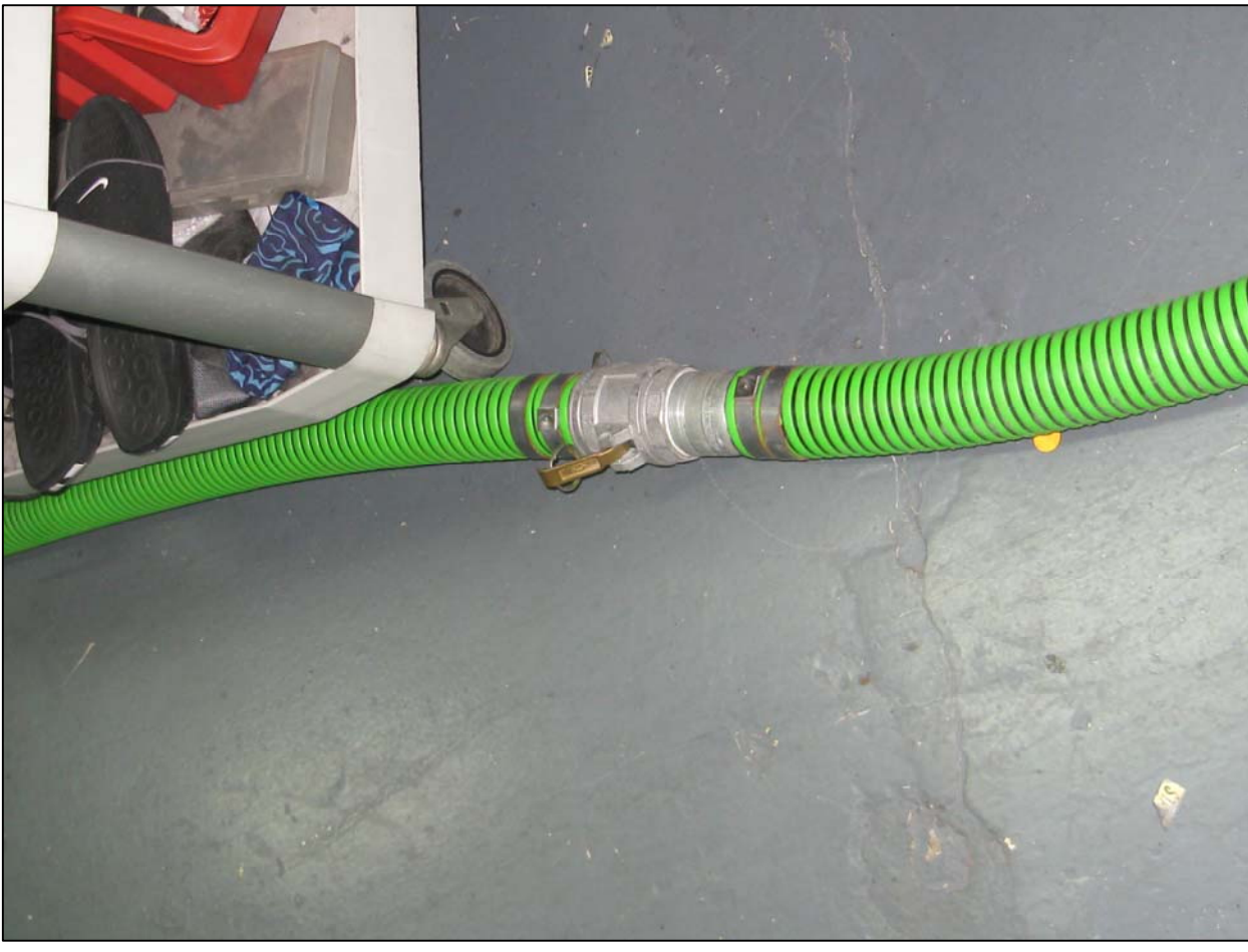
Photo 4. Hose for connection from shop vac to extraction point XP2.
