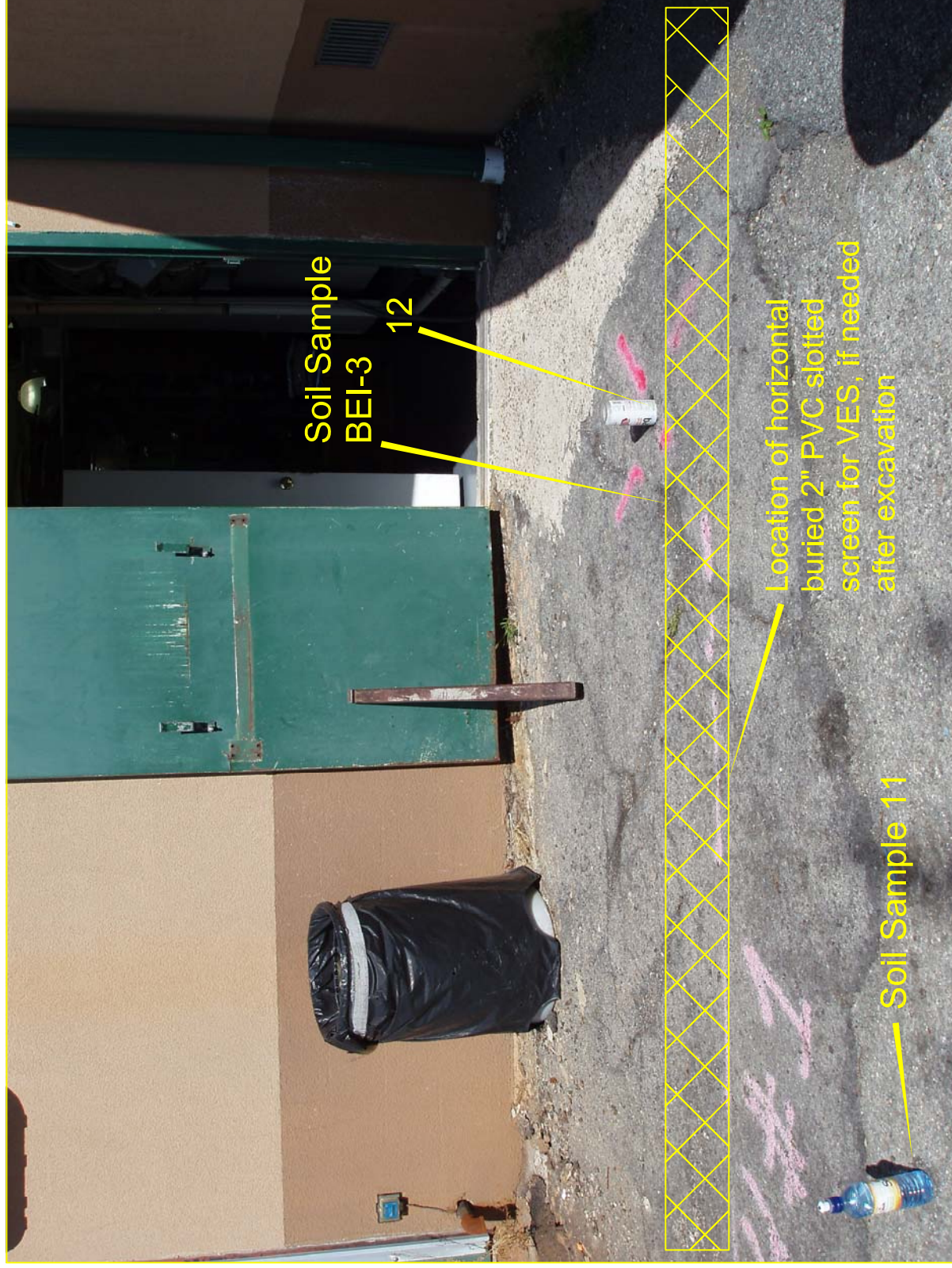
Figure 8. Area of excavation by back door to remove PCE-contamination at Sample #12S Vapor Extraction System at American Cleaners at 360 Route 211 East, Middletown, NY 10940 NYSDEC DER VCP V-00461-3, September 2012
