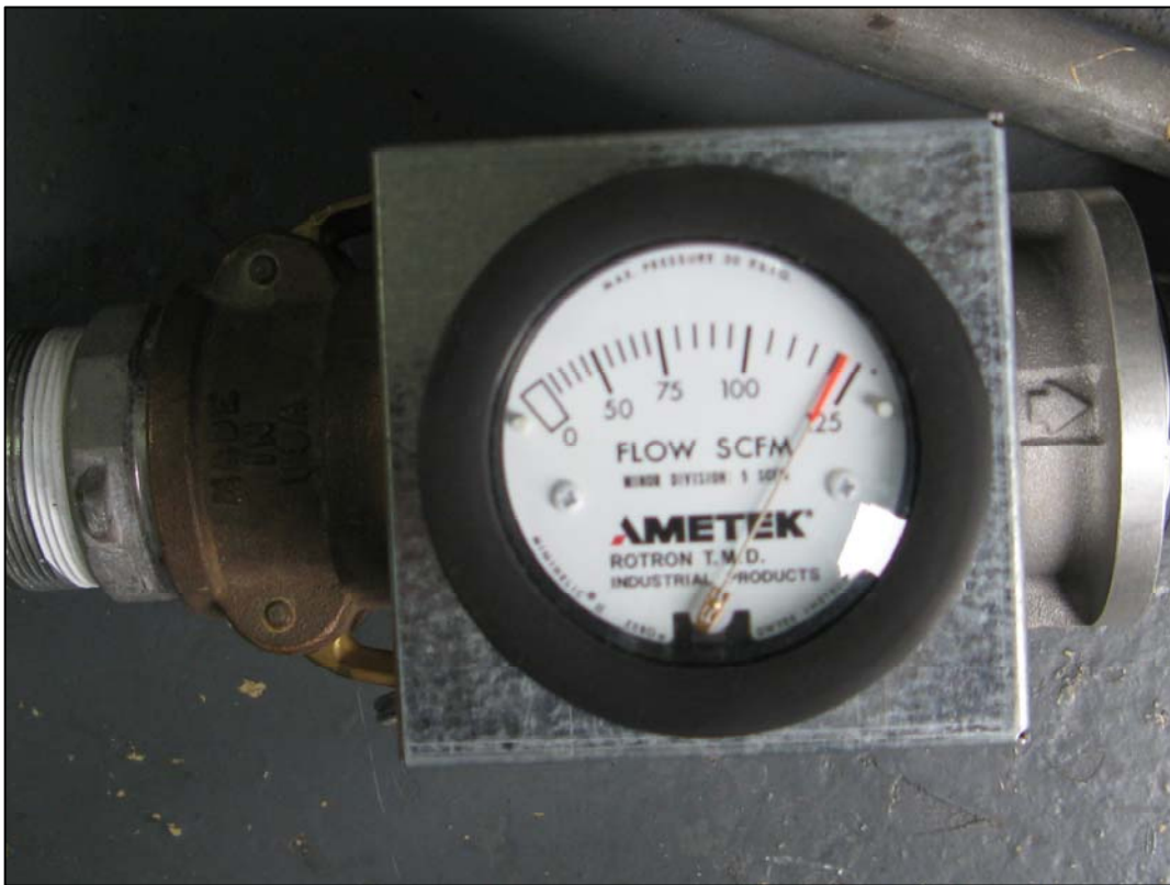
Photo 5. Air flow meter, blower on, no connection to XP2, 120 cfm.
