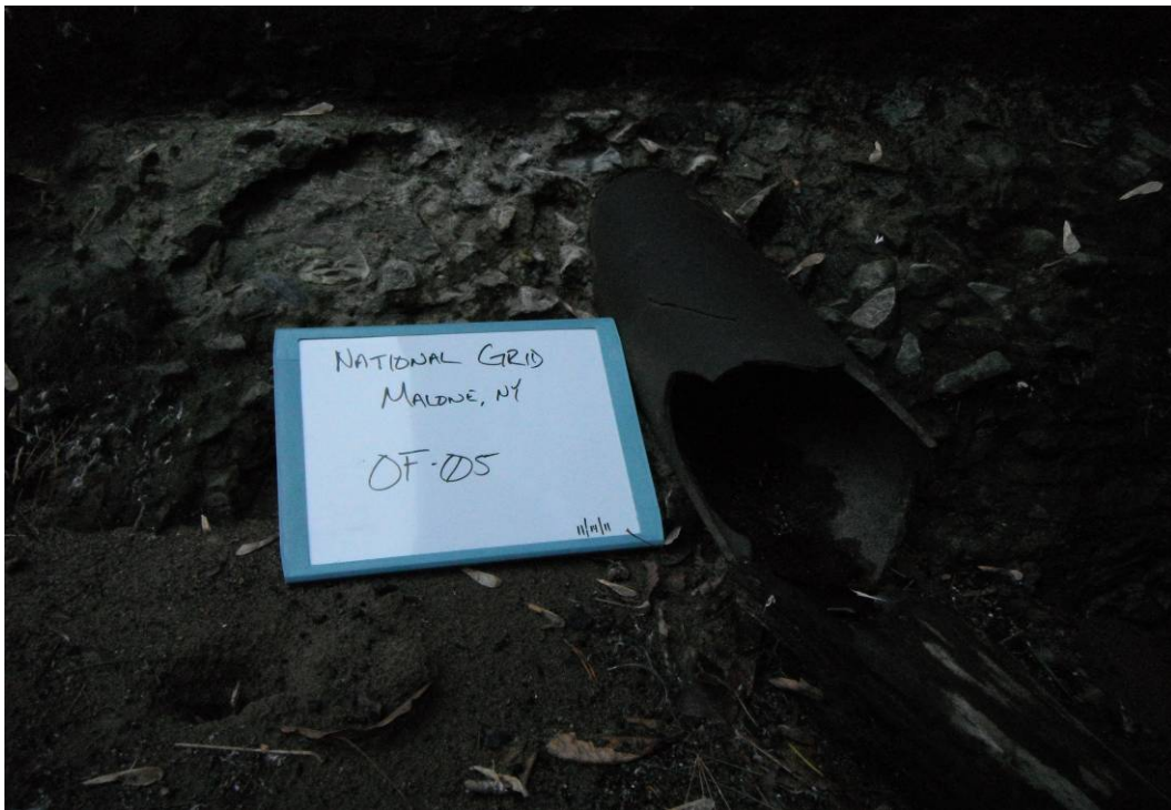
OF-05: 8" Cast iron pipe on east side of river bank and tucked into corner of building that has the old power-generator. This is also the general location of sediment sample NG-SR-SD-16. No discharge observed at time of photo.
