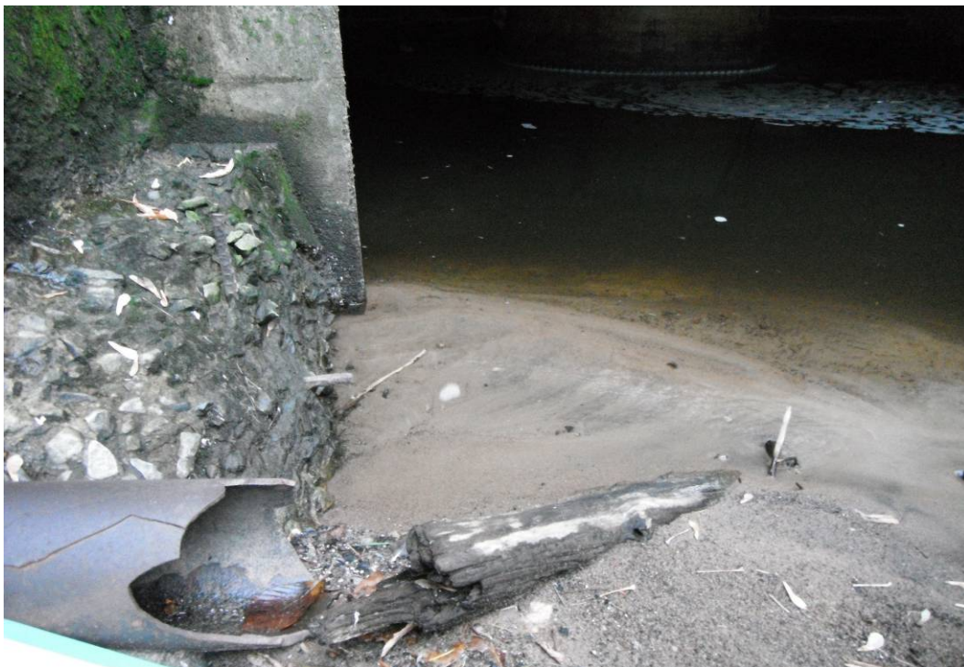
OF-05: In the background you can see the old power-generator looking upstream.
