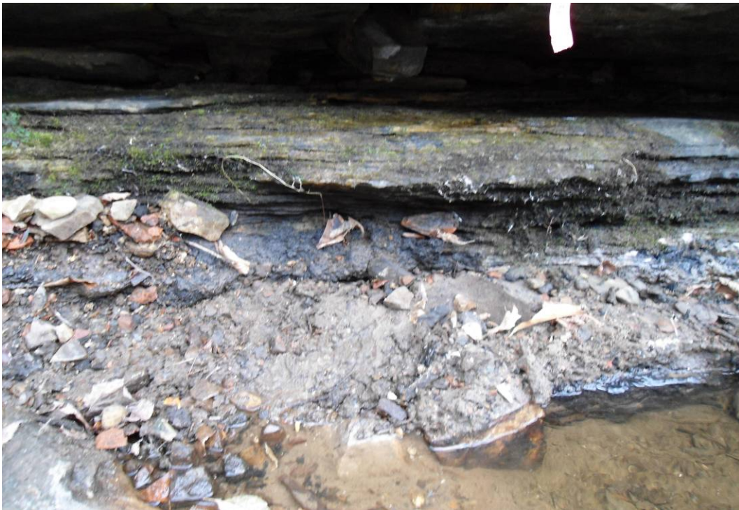
GP-04: West side of riverbank at a section of tar seam in the rock wall-face. Survey point in upper right hand corner is NG-SR-SD-02
