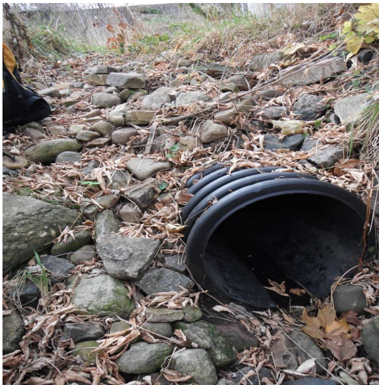
OF-03 (continued): Looking up the river bank on the west side.
