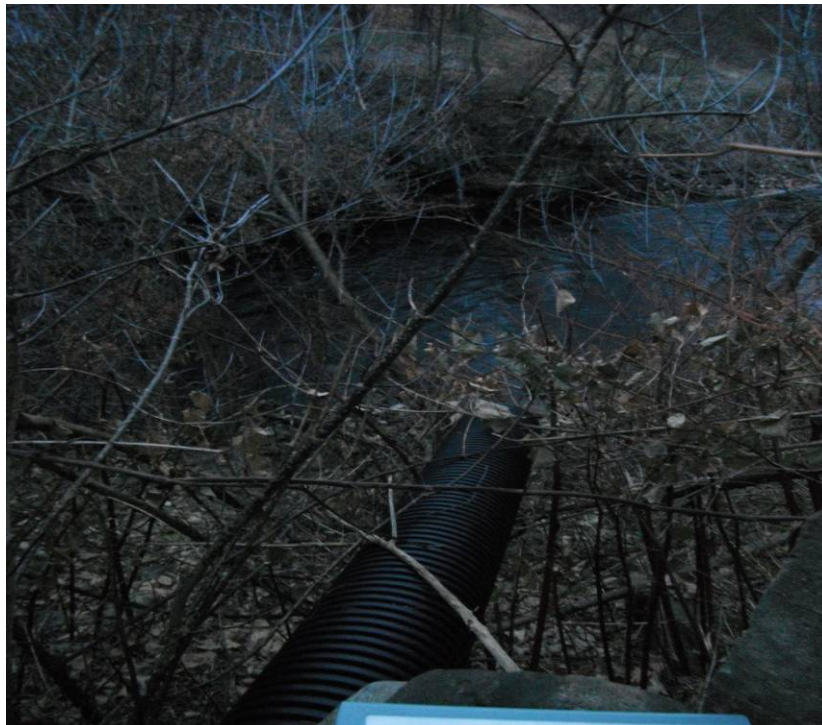
OF-08 (continued): From pipe looking west into river. Site is in the background on opposite side of river.
