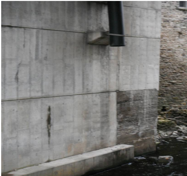
GP-14: Picture of the more downstream of the two 24" metal pipes under bridge on west side of river.
