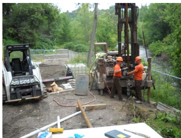
Figure 2-1 Typical Setup for Drilling Borings, Monitoring Well MW-8R shown, looking north
