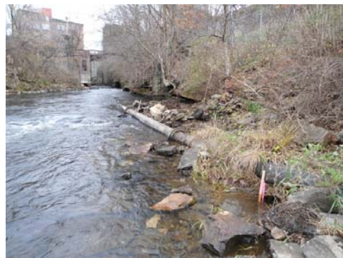
Figure 2-3 Salmon River adjacent to site, facing south, Notice sanitary sewer pipe on riverbed.
