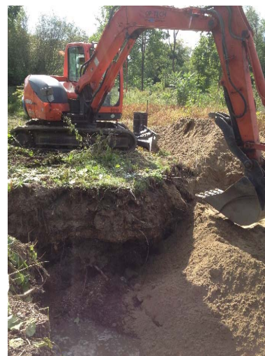
Figure 1-3 Backfilling IRM excavation with clean fill
