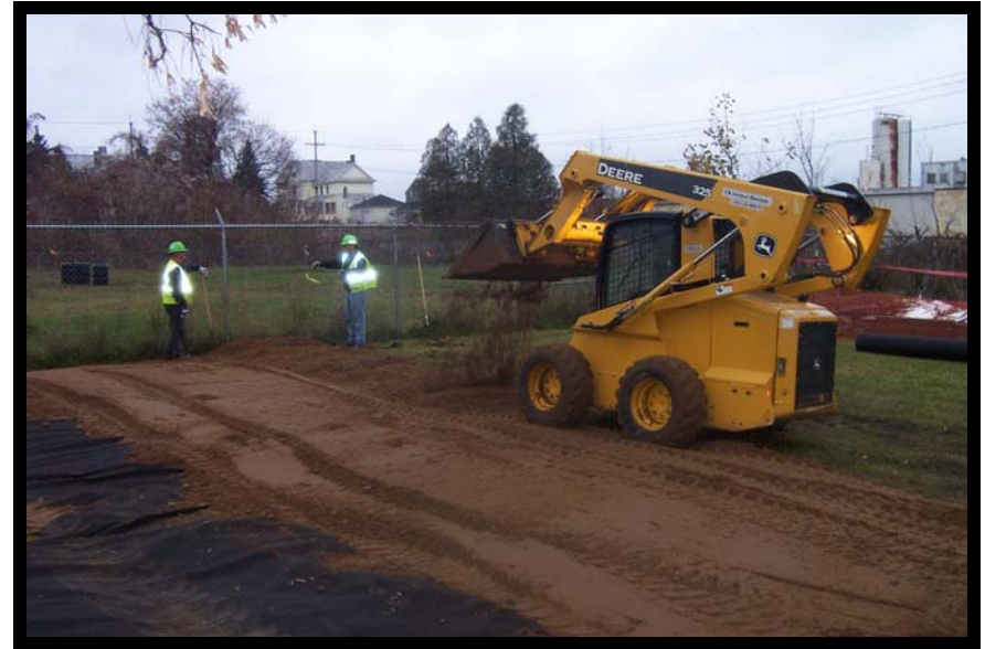
Placement of Select Fill Material
