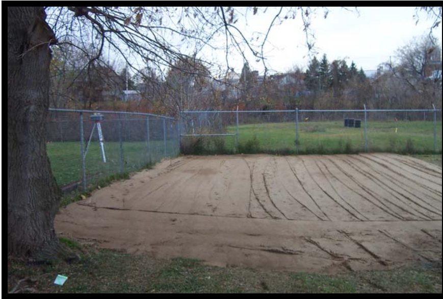
Completion of First Layer of Select Fill Material
