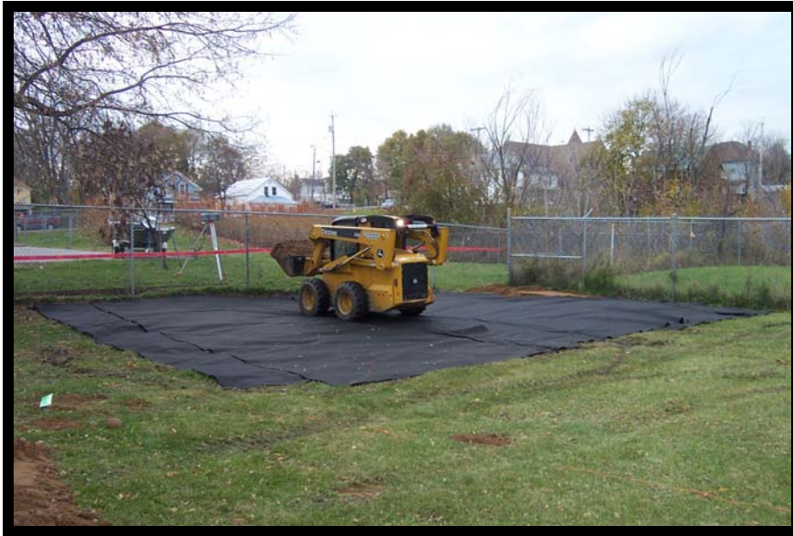
Placement of Geotextile Material
