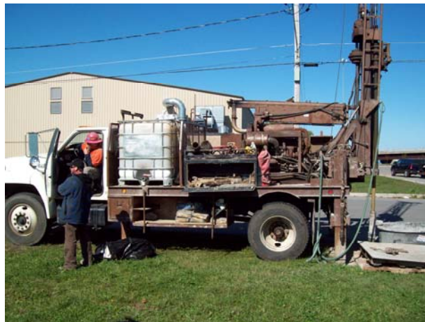
Figure 2.1: Typical Setup for Drilling Borings, monitoring well MW-20R shown, looking north
