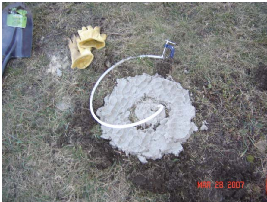
Photo 2 Sampling Location VP-1A Bentonite Seal Installation – Adjacent to 2 King Street
