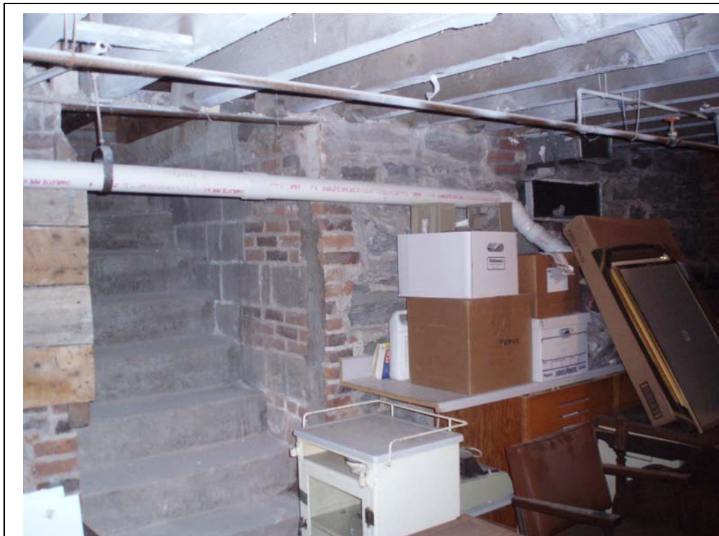
Photograph #3 – View of old stairwell to outside located at eastern end of basement.
