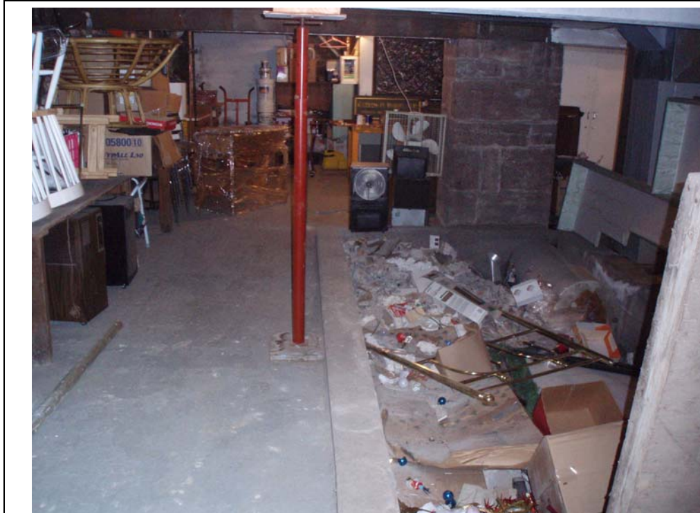
Photograph #2 – General view of basement. Top of photo is west.
