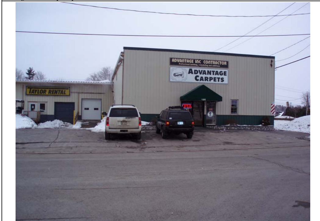
Photograph #6 – View of exterior of Advantage Carpets portion of building. Top of photo is east.
