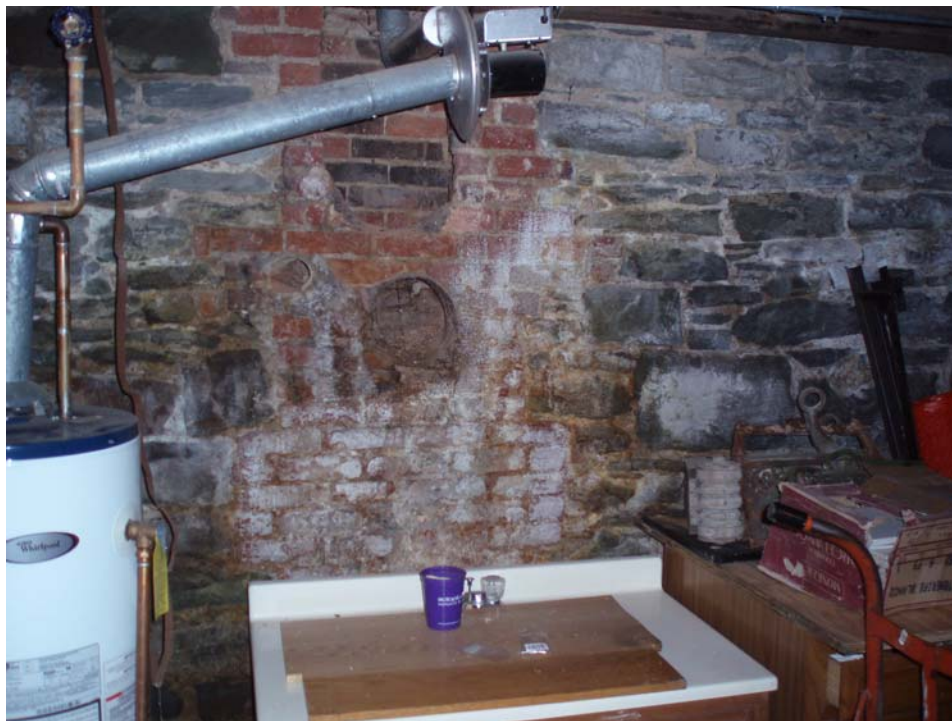
Photograph #5 – View of foundation wall condition.
