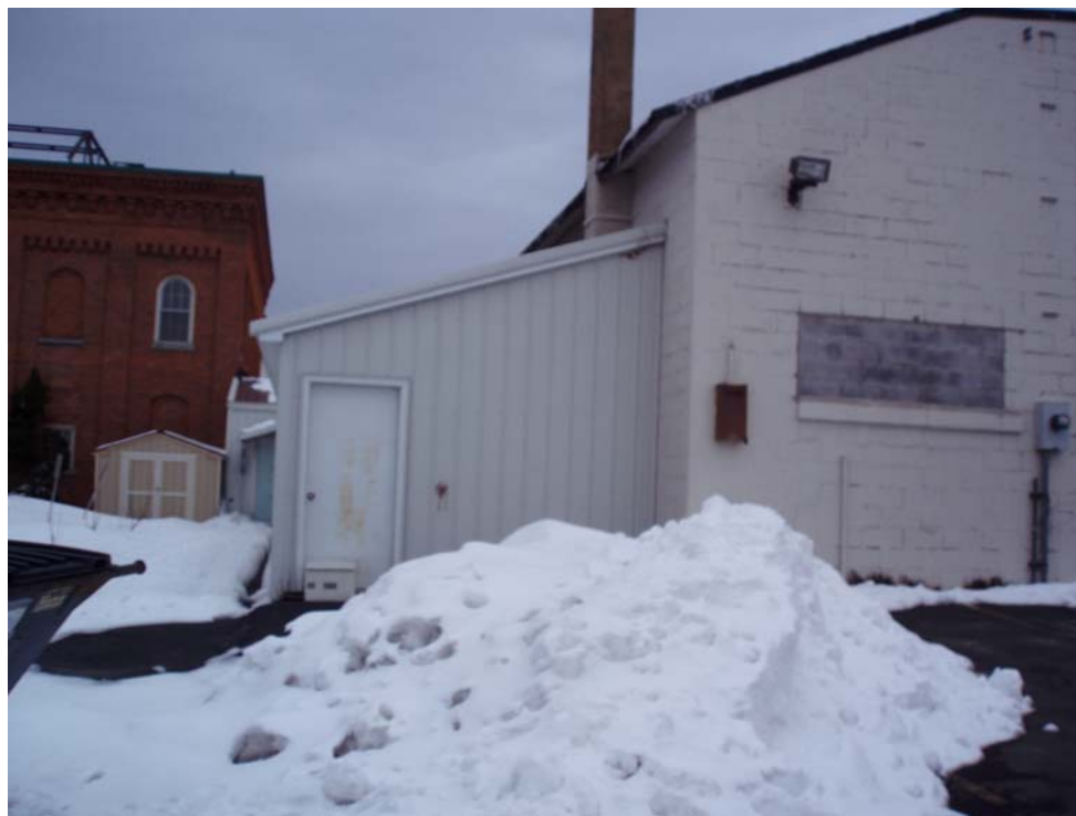
Photograph #6 – View of exterior of storage area, where sampling of sub-slab vapor and indoor air was performed.
