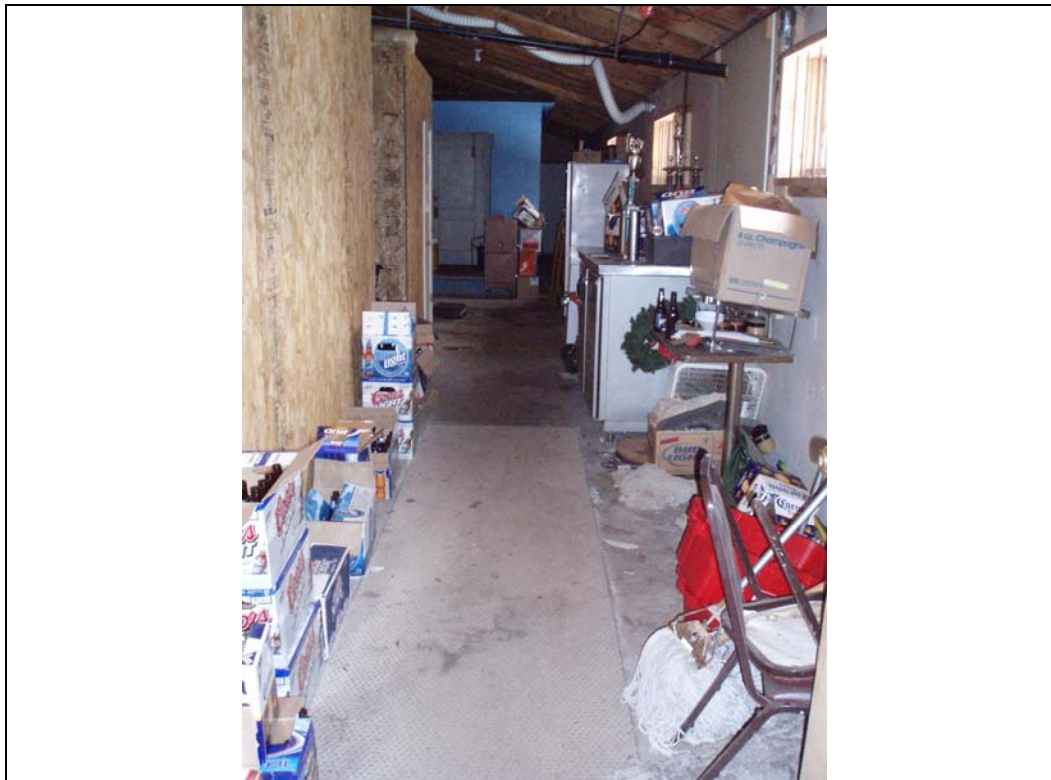
Photograph #1 –General view of storage area. Top of photo is south.
