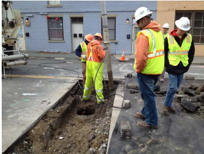
Test pit TP-1-13 in Hill Street near the southern tar well
