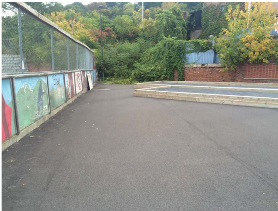
Soil Cover System (asphalt) at Site, looking east toward bocce courts.
