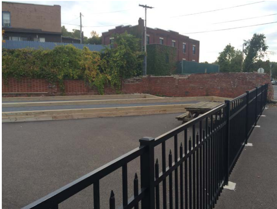
Soil Cover System (asphalt) at Site, looking southeast along re-installed fencing. The southern tar well was located below the soil cover shown here.
