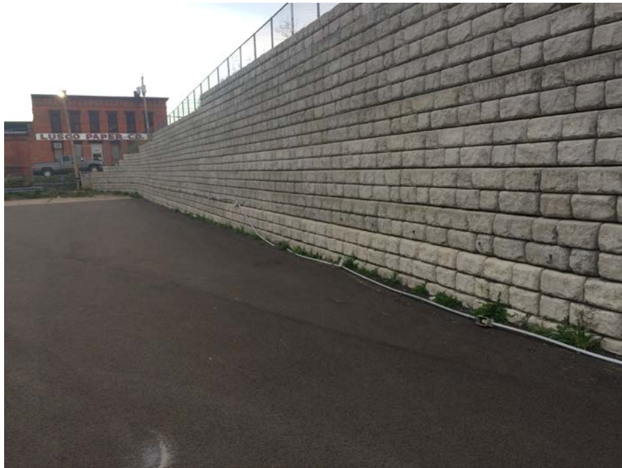
Soil Cover System (asphalt) at Site, looking north along the retaining wall on the east side of the Site.
