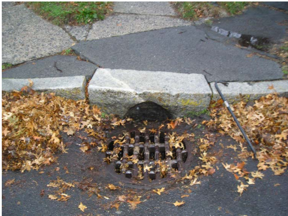
Photograph #3 – View of catch basin (CB#3) located along northern side of Huyck Square, near intersection of Huyck Sq. and Washington St. Substantial amount of debris within catch basin; unable to determine flow direction, appeared to be stagnant. Top of photo is north-northeast.
