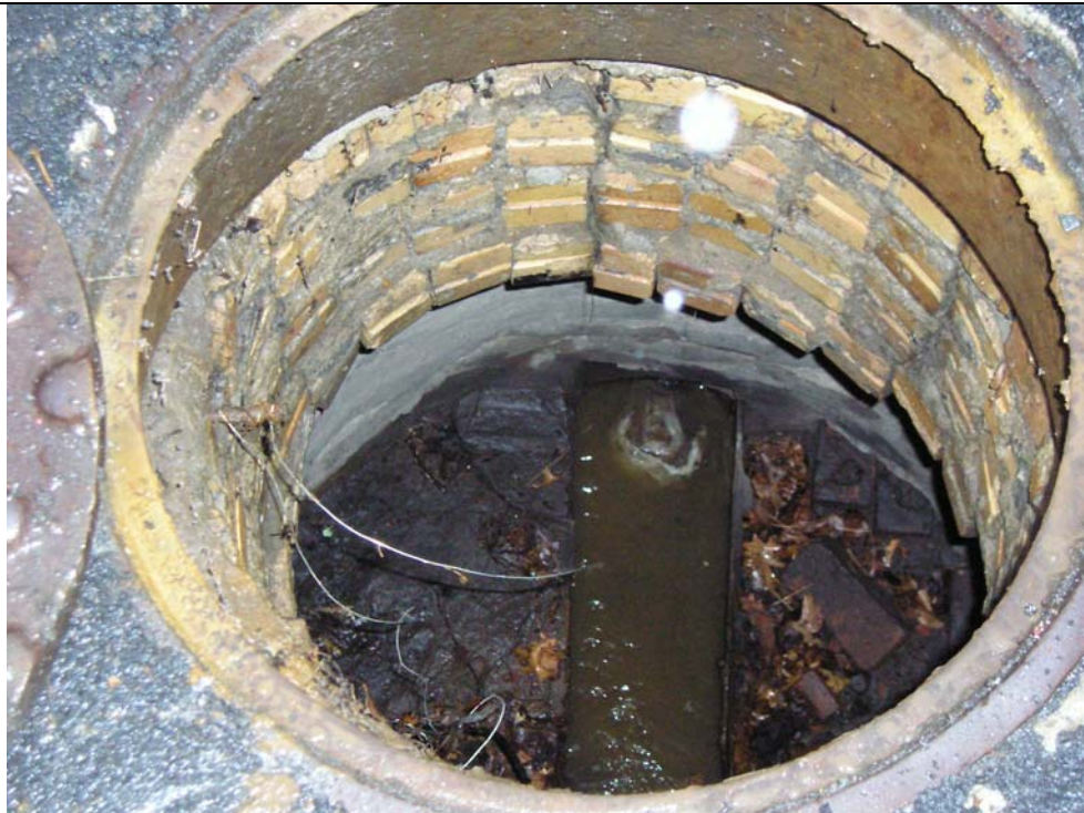
Photograph #5 – Close-up view of flow within sanitary sewer. Top of photo is south.
