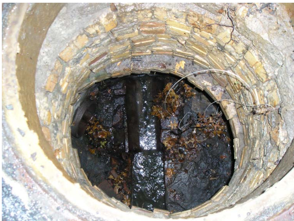
Photograph #4 – Washington St. manhole (MH#1) for sanitary sewer line. Flow direction is to the south. Slight sewage odor.
