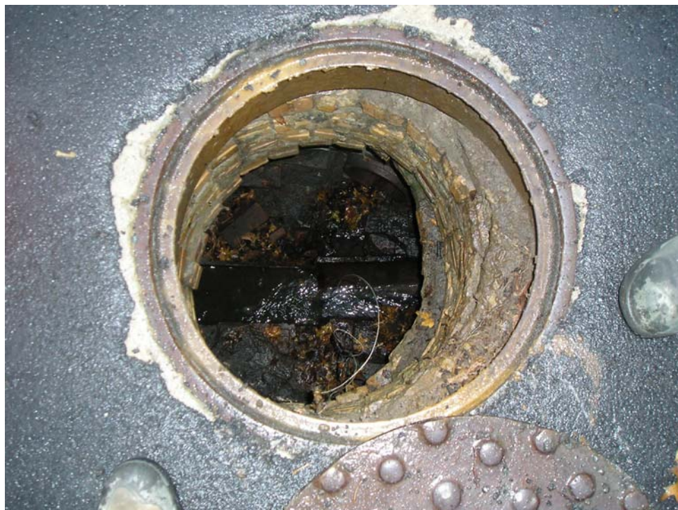
Photograph #7 – Overhead view of MH#1.
