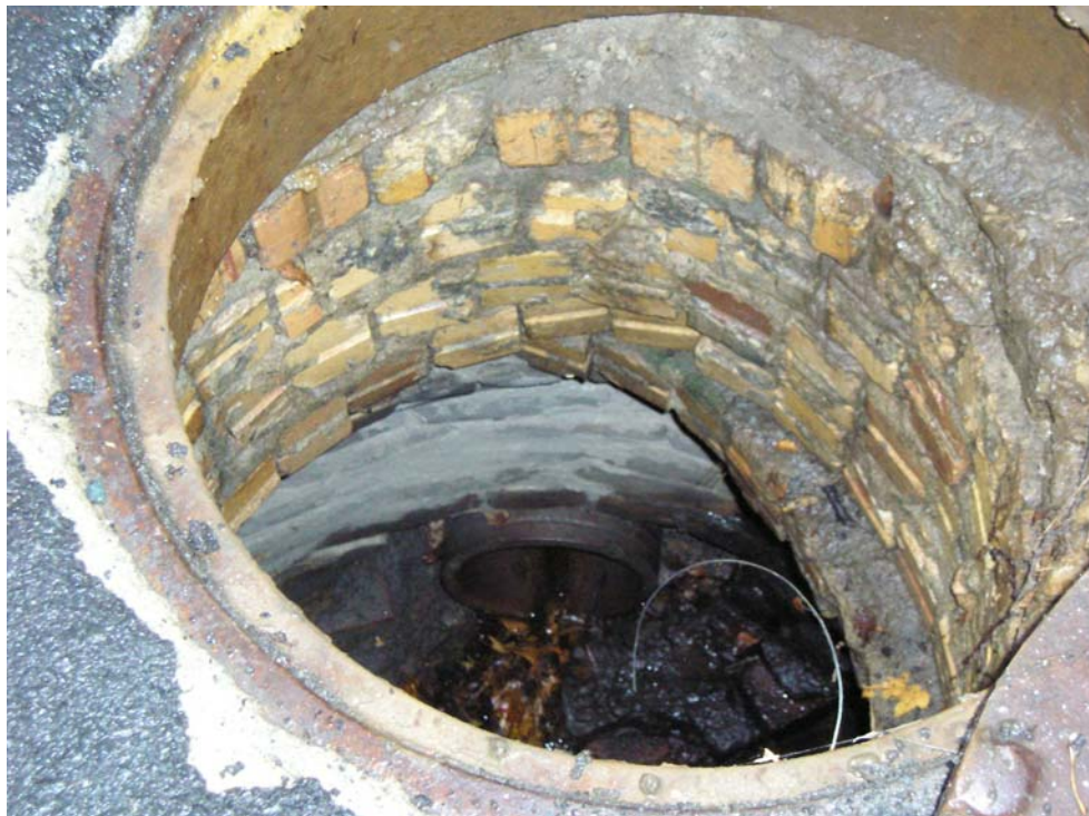
Photograph #6 – View of NW-SE oriented inlet pipe observed within MH#1, pipe is approximately 14" in diameter. Minimal flow observed exiting pipe into sewer.
