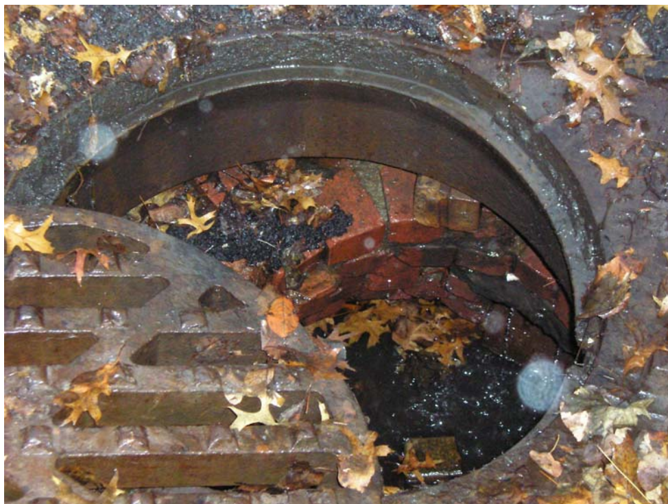
Photograph #2 – View of infiltrating storm water into catch basin (CB#2) located along western side of Washington St., near intersection of Huyck Sq. and Washington St. Top of photo is east.
