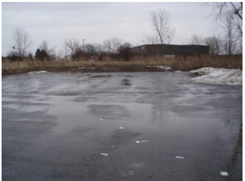
Completed Driveway Expansion
