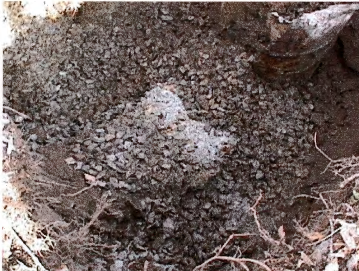
Crushed stone used in dry well construction – photo taken 1/29/03
