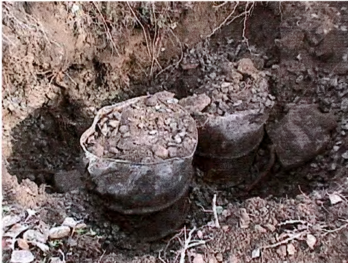
Drums used to construct dry well – photo taken 1/29/03
