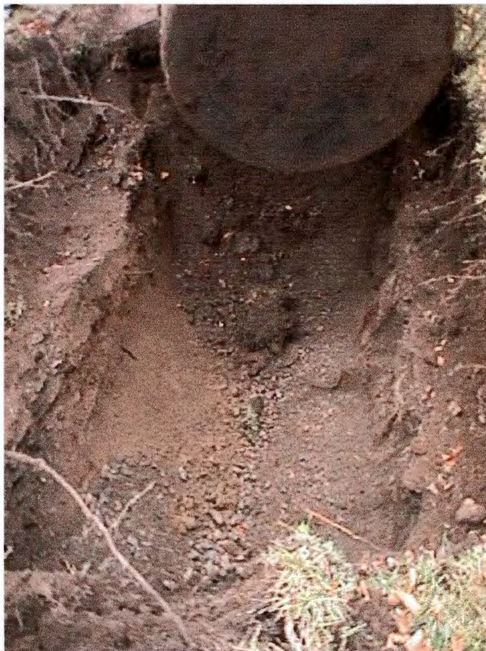
Excavation bottom – photo taken 1/29/03
