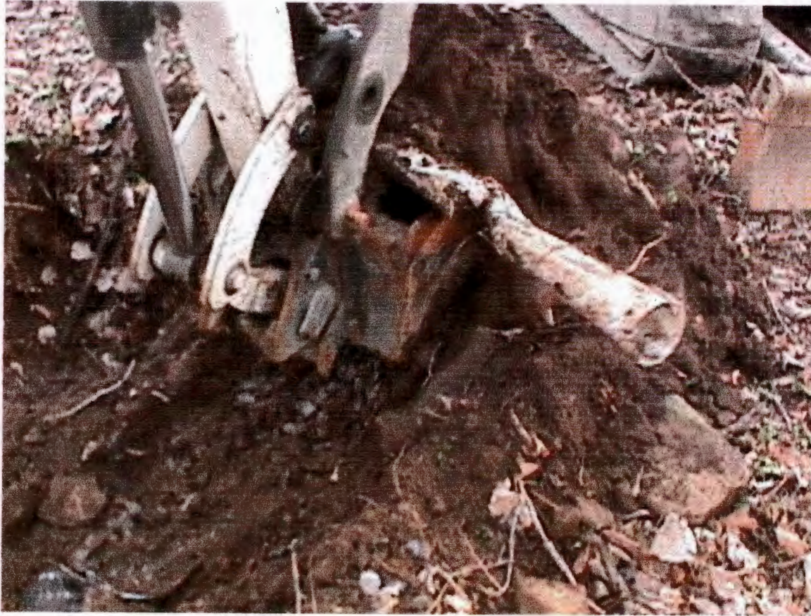
Excavation of dry well – 1/29/03
