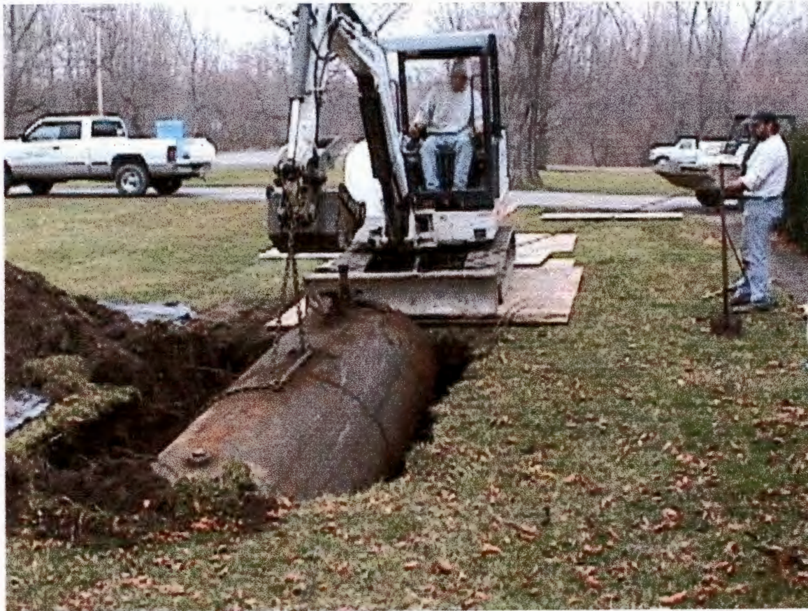
Removal of 1,000-gallon fuel oil UST – 1/29/03
