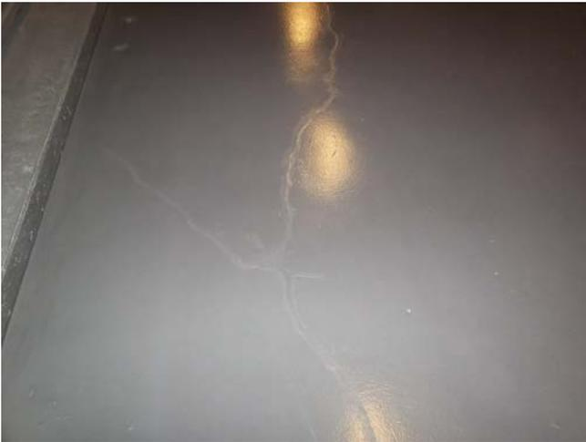
Photo 5: View of sealed crack in Room 0021.
