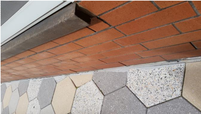
Photo 9: View of recaulked areas around the perimeter of the school.
