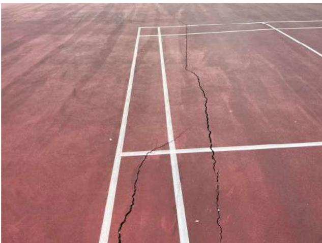
Photo 11: View of typical moderate crack on the tennis court.
