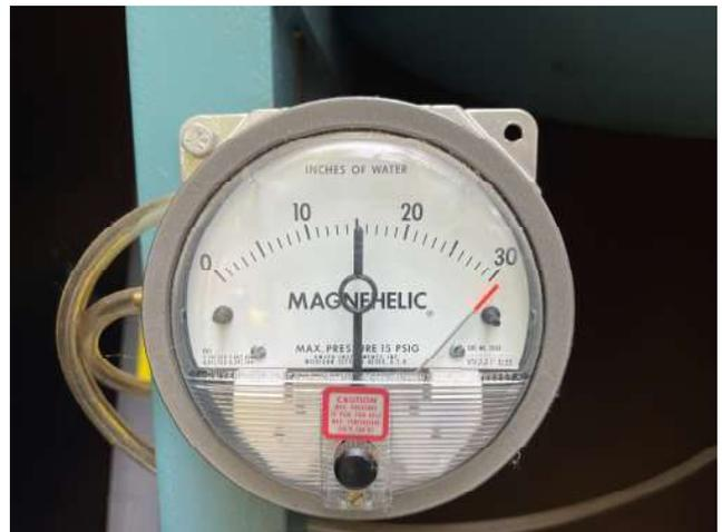
Photo 4: View of the SSDS vacuum gage.
