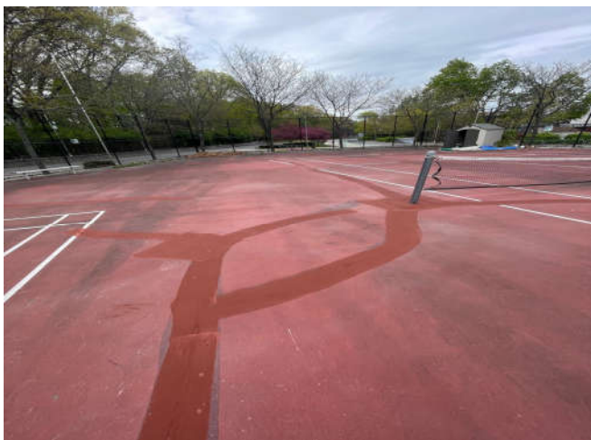
Photo 11: View of crack repairs on the tennis court.
