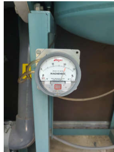
Photo 4: View of the SSDS vacuum gage.
