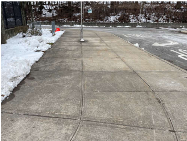
Photo 9: View of typical exterior pavement.
