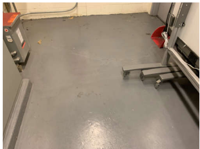
Photo 68: View of typical bare concrete floor in Room 0023
