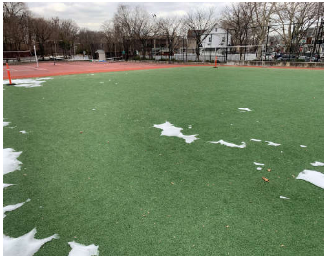
Photo 8: View of typical artificial turf around the tennis courts.
