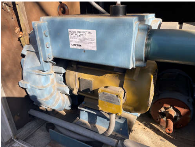
Photo 3: View of the active SSDS fan motor.
