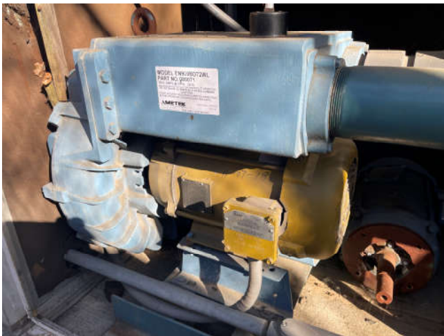
Photo 3: View of the active SSDS fan motor.
