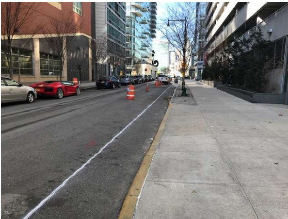
Photo 3. View of micro-trench (white line) along 46 th Ave. (facing west).
