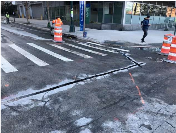
Photo 7. View from 5 th St. and 46 th Ave. intersection and tar sealed micro-trench (facing northwest).
