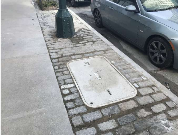
Photo 13. View restored pavers at Site cover inspection.
