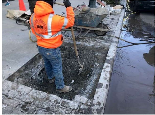
Photo 10. Beginning of trench excavation along Center Blvd.
