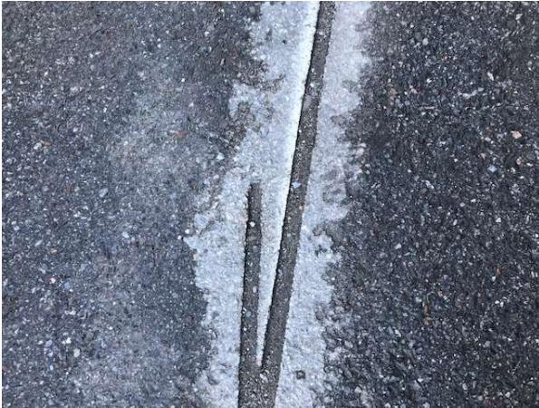
Photo 5. Close-up of micro trench.
