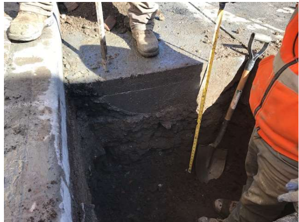
Photo 4. Small trench on 5 th Street to connect conduit box to telecommunications infrastructure.
