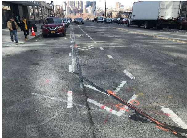
Photo 16. View of sealed micro-trench from intersection of Center Blvd. and 46 th Ave. (facing northwest).
