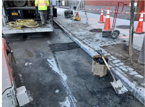
Photo 6. Trench on 5 th St. refilled and recovered with asphalt.
