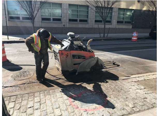
Photo 2. Walk behind concrete saw opening up conduit micro trench on 46 th Ave. (facing south).
