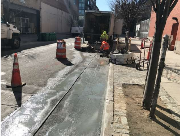
Photo 1. Excavation work on 5 th St. with P.S. 78 on the left. (facing south).
