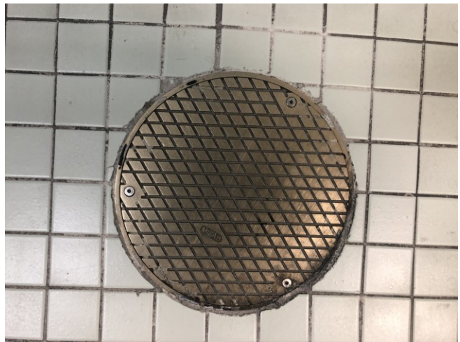
Photo 6: View of typical monitoring point in Room 127.
