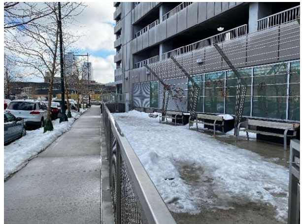
Photo 10: View facing east along North Basin Blvd. with 45-45 Center Blvd. to the right (C241096)
