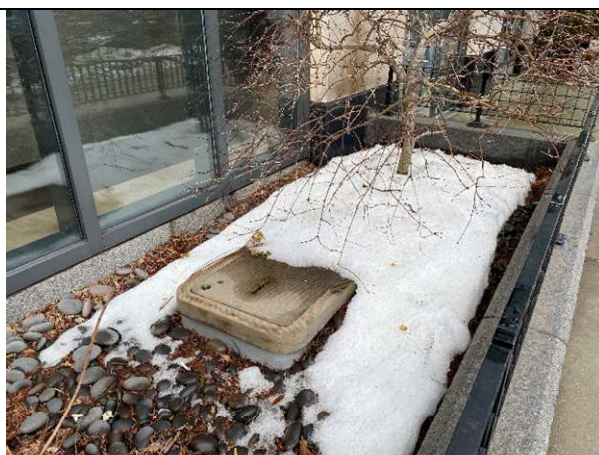
Photo 28: Cover for upgradient ORC injection points at 47-20 Center Blvd. (V00505A)
