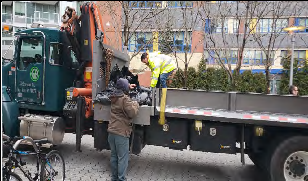
Photograph 2 - Loading heavy duty plastic bags containing soil/fill into a truck.
