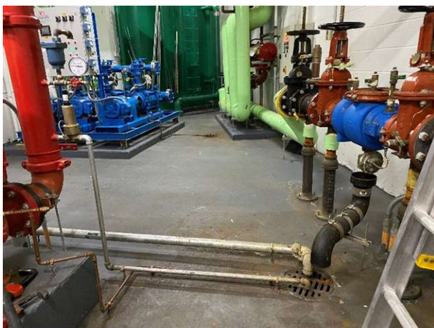
Photo 19: View of slab in water pump room of 46-10 Center Blvd. (C241096)
