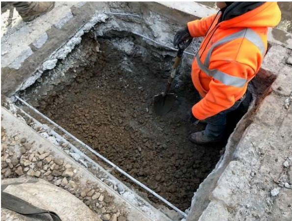
Photo 11. Final trench depth along Center Blvd.
