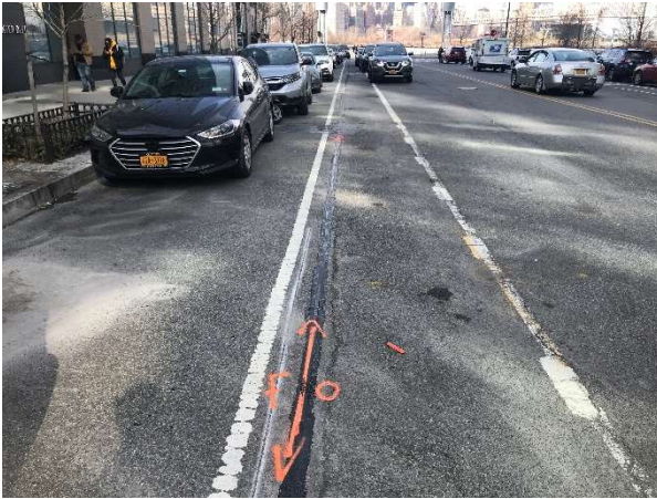
Photo 15. View of sealed micro-trench on Center Blvd. (facing northwest).
