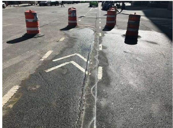
Photo 12. View of micro-trench for conduit along at intersection of 46 th Ave. and Center Blvd. (facing south).
