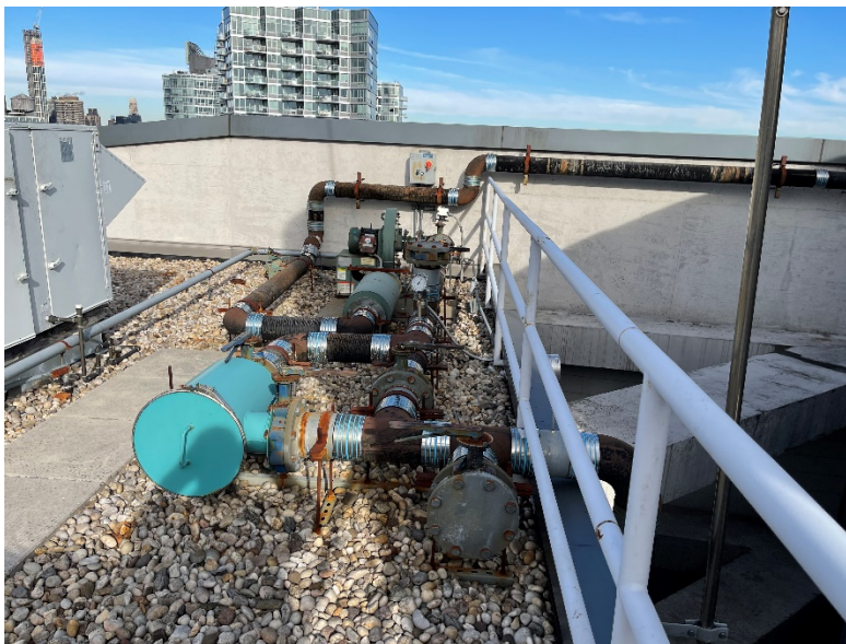
1. Sub-Slab Depressurization System Operational On Roof
