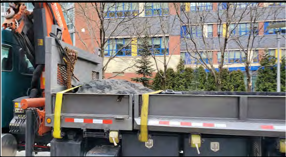
Photograph 3 - Heavy duty plastic bags containing soil/fill covered with tarp and secured in a truck.
