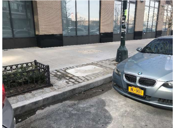
Photo 14. View restored pavers at Site cover inspection from Center Blvd.
