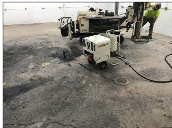
Photo 6: GP-300 used to inject HRC.
