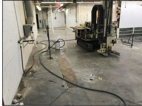
Photo 2: GeoProbe unit parked next to injection points.
