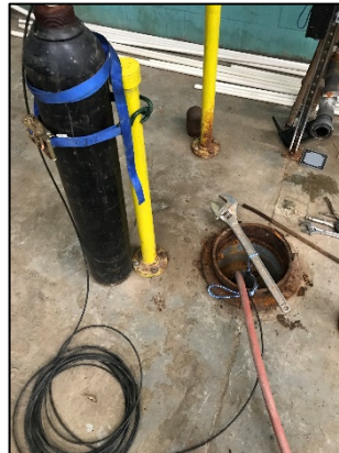
Photo 4: Close up of well packer set up in PW-1R.
