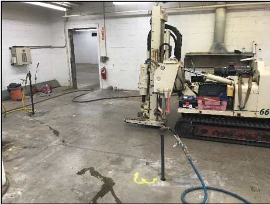
Photo 3: View showing 3 injection points.
