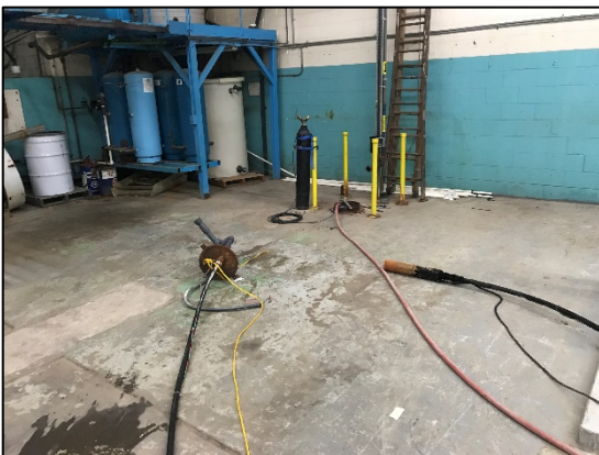
Photo 5: Pumping system removed from PW-1R.
