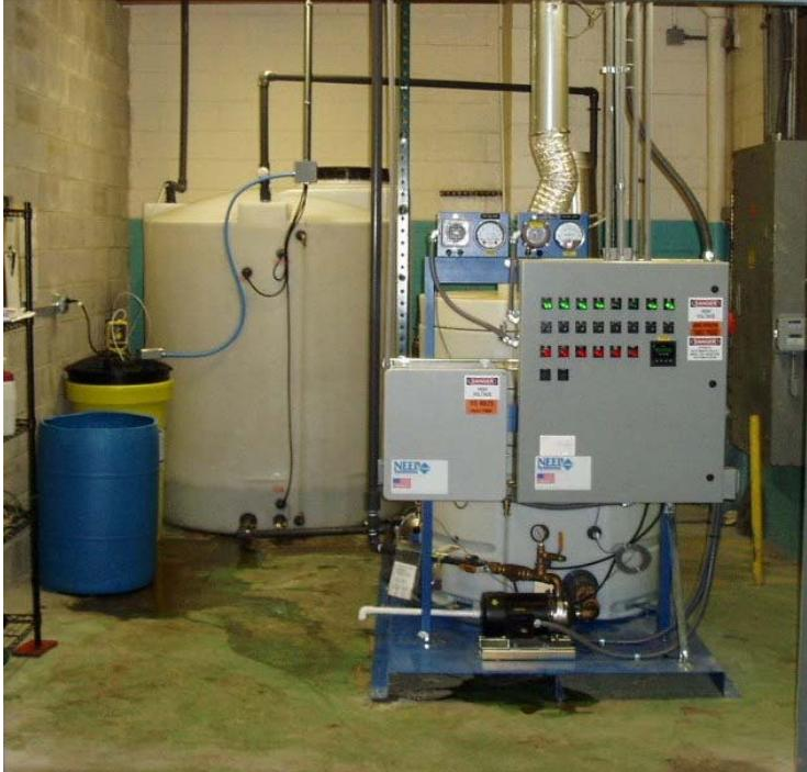
A photograph showing a pretreatment system in a industrial setting. The system consists of a large white vertical tank, a smaller blue drum, and a control panel with various gauges and valves. The floor is concrete and shows some staining. The background includes brick walls and other industrial equipment. |                                     |
