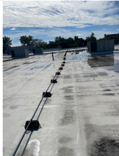
Typical existing electric conduit across roof to blower
