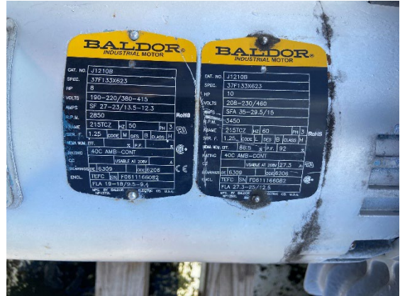
Blower #1 specification placard (9.26.25)
