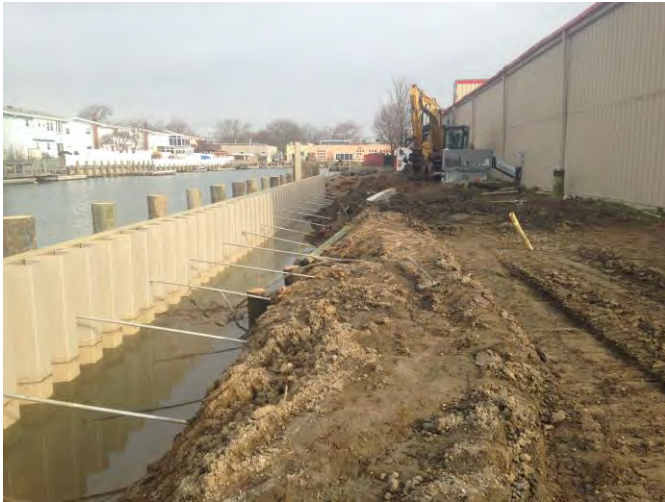
Figure 1. View of bulkhead work area along the western side. No activities were performed today.
