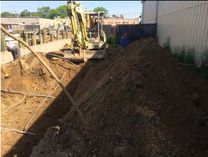
Figure 1. View looking north
