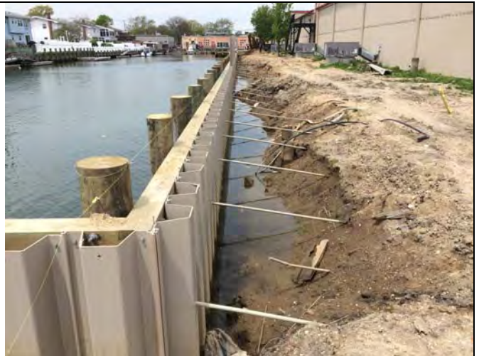
Figure 2. View looking north.
