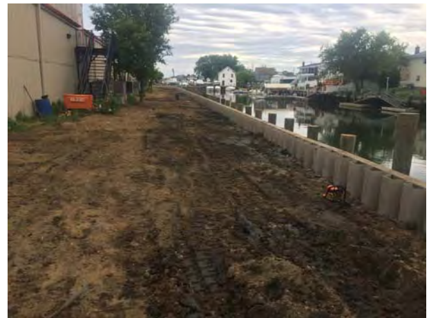
Figure 4. view from north
