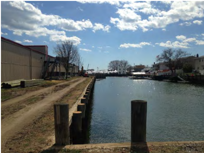
Figure 3. View of bulkhead to be replaced along western side.
