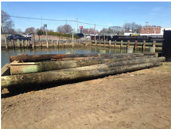
Figure 3. View of former pilings removed during work activities.
