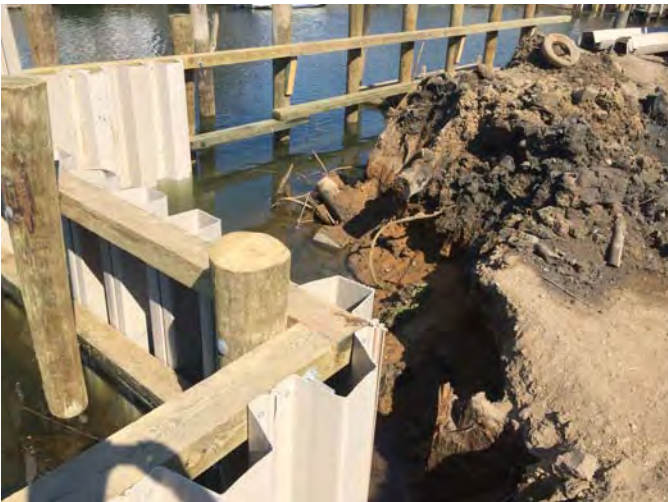
Figure 3. northwest area of bulkhead
