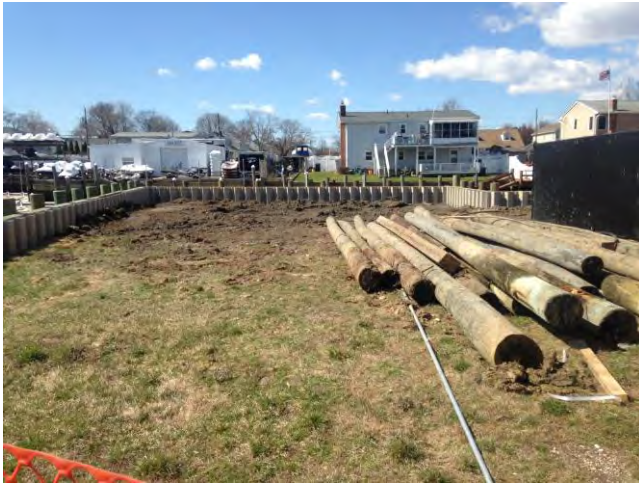
Figure 1. View of previously replaced bulkhead along the southwestern side.
