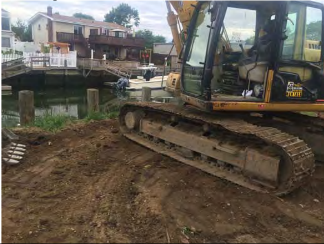
Figure 1. Northwest corner of bulkhead
