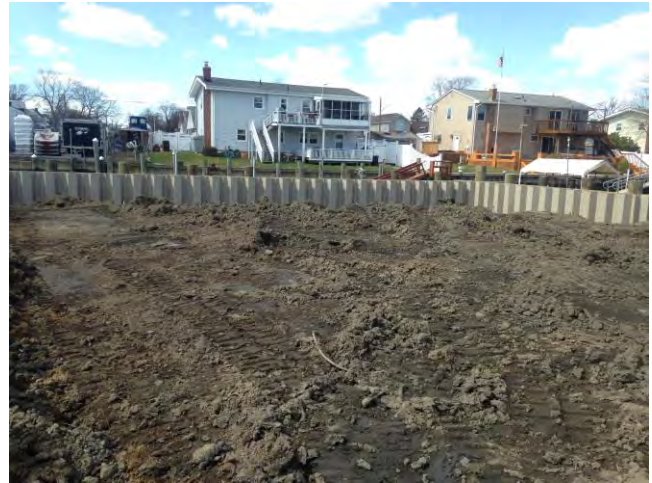
Figure 2. View previously disturbed surface soils.
