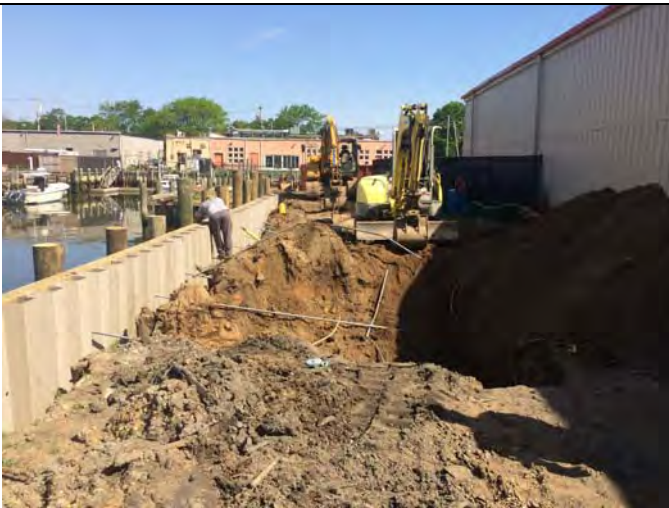
Figure 3. View looking north.
