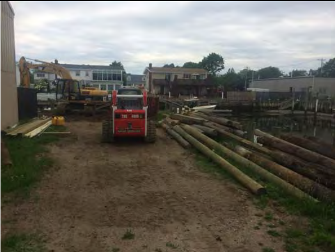
Figure 3. view from east
