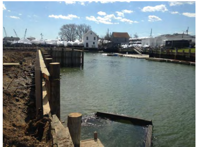
Figure 2. View new bulkhead section with soils back in place.
